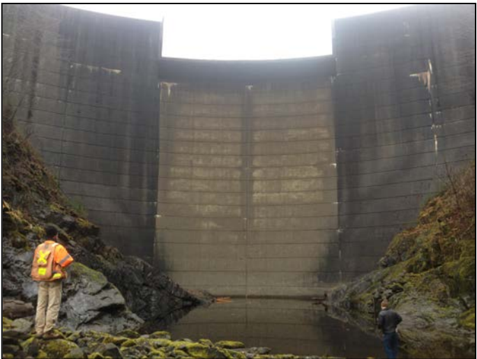
Jacobs Associates assessing geologic conditions at and above the Swan Lake plunge pool.
