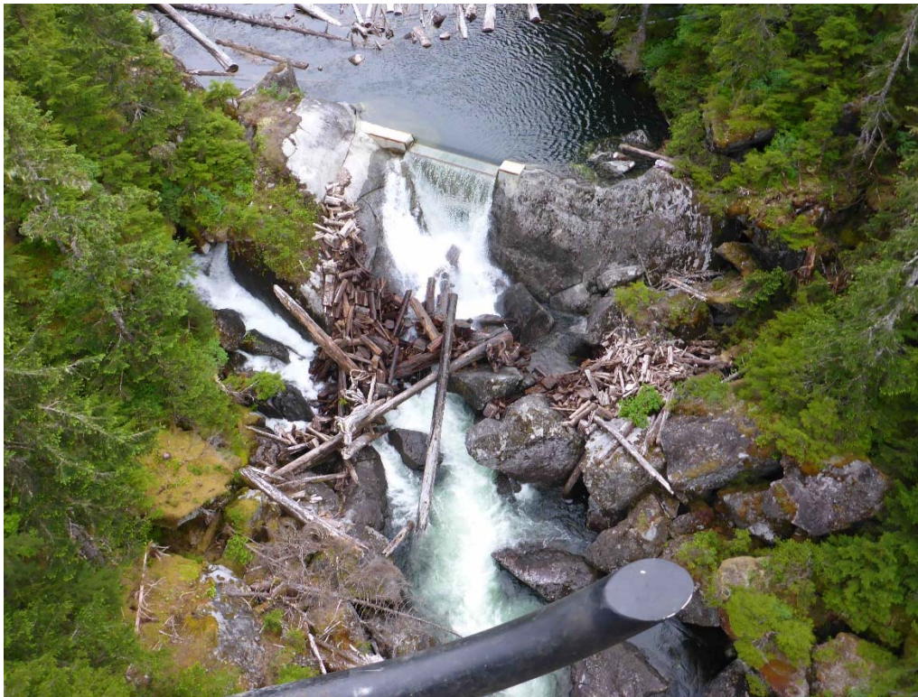
Weir spill – June 2016
