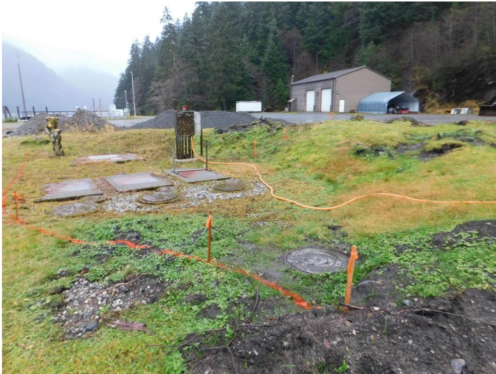
Above: Existing waste water system with new septic field outline.
