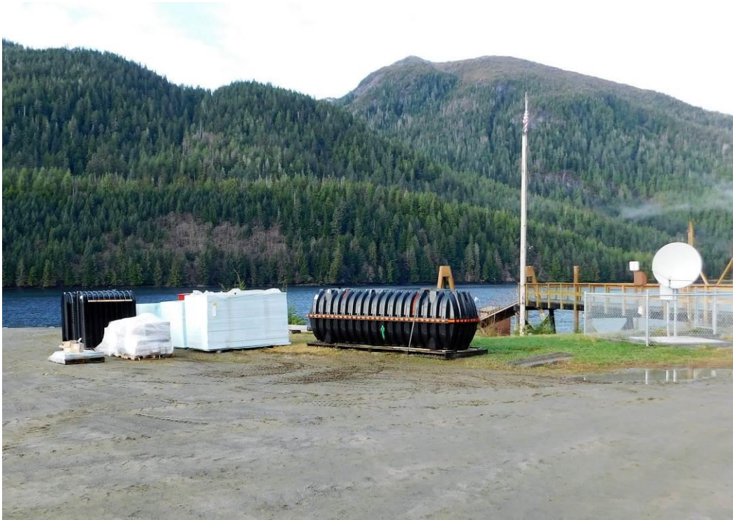
Above/Below: Parts (primary tank & foam sheets) for new septic field system arrive
