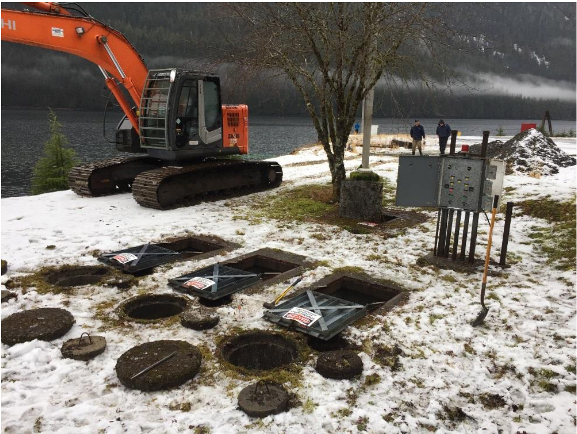
Swan Lake Wastewater Treatment Plant
