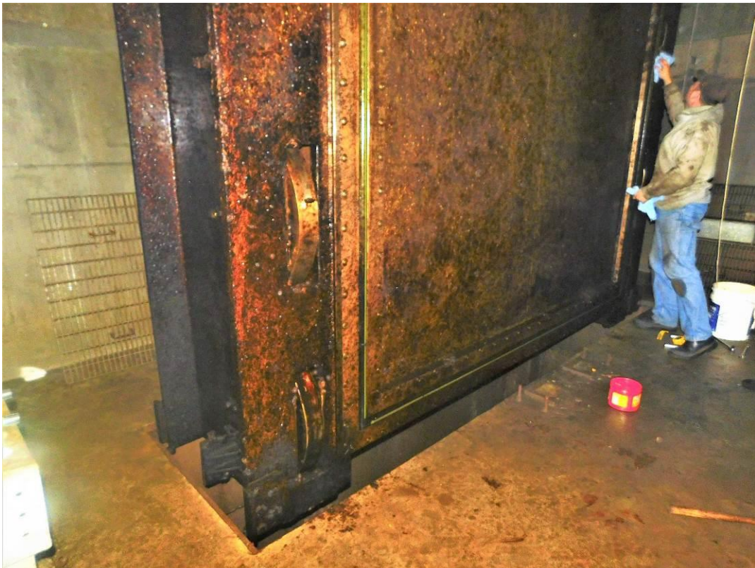
Above/Below: intake gate inspections
