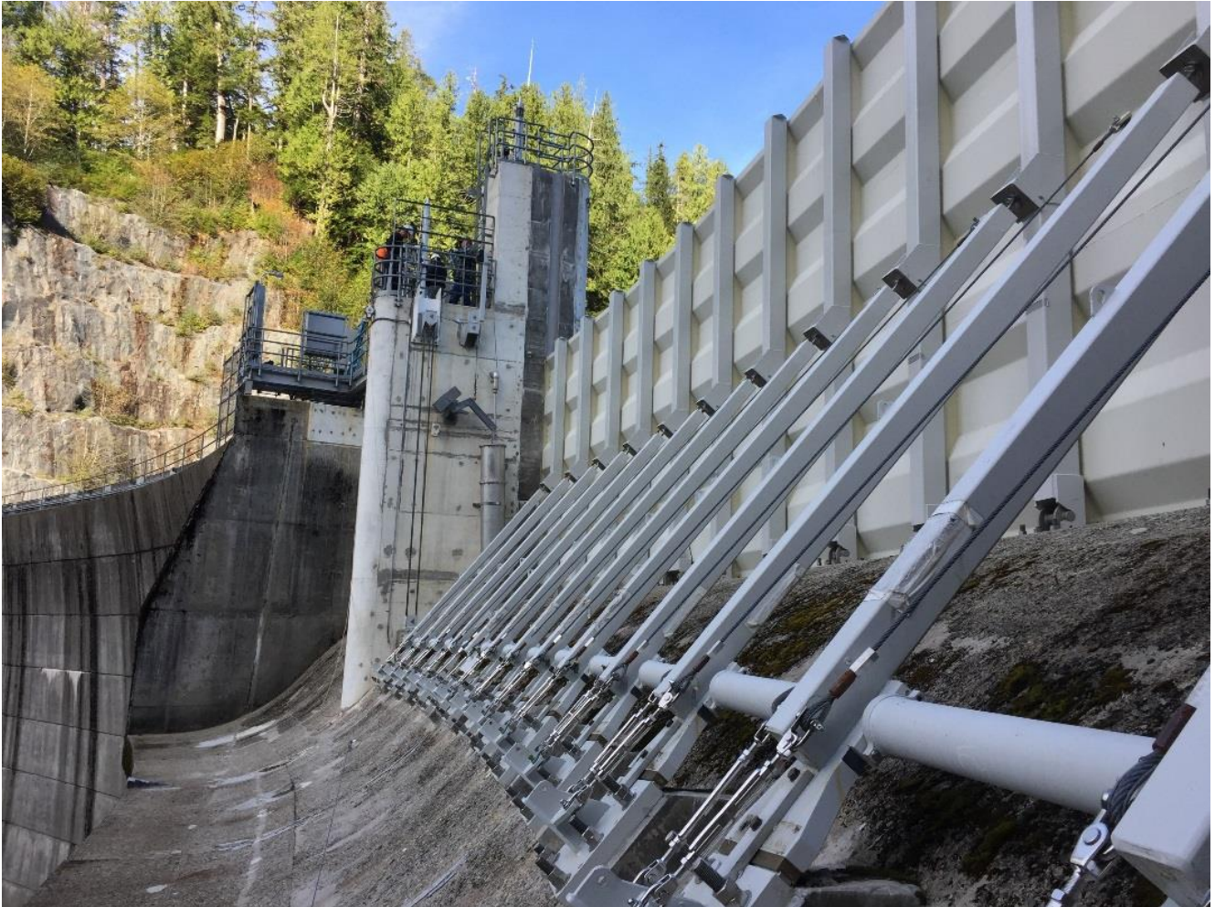
Swan Lake Flash Board Gate System
