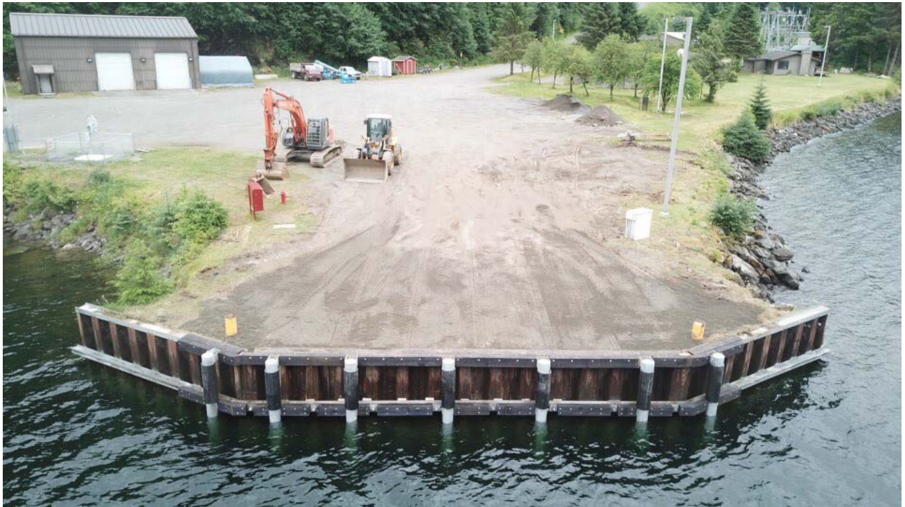
Renovated Swan Lake Marine Bulkhead July 11, 2018
