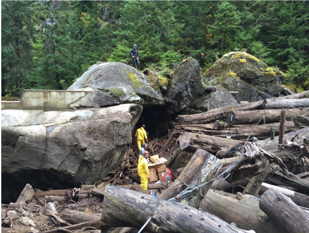
Foam Filling Voids in Weir Rock Foundation Abutments
