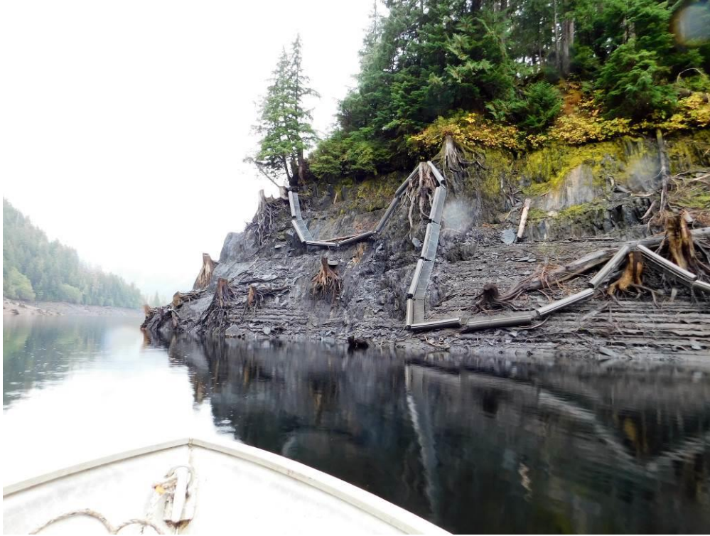
Above: a broken aux. log boom along the lake bank. Higher lake level needed for recovery
