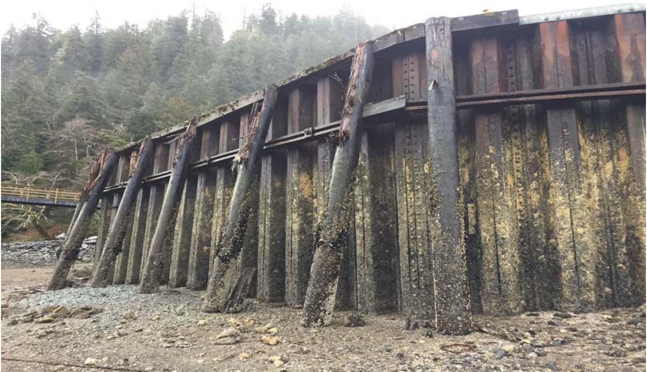
Bulkhead Prior to Renovation
