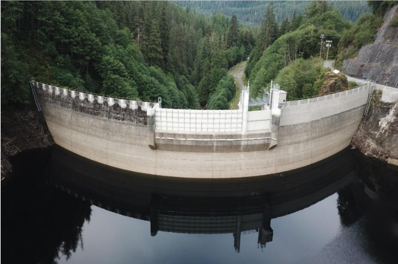
Swan Lake Dam Access Ladders / Right & Left Abutments
