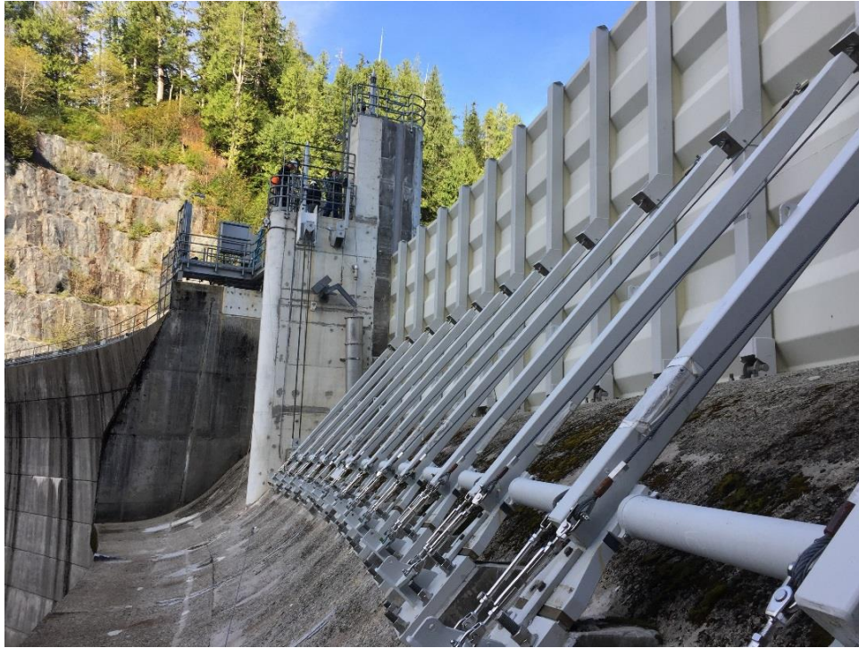
Swan Lake Flashboard Gate System
