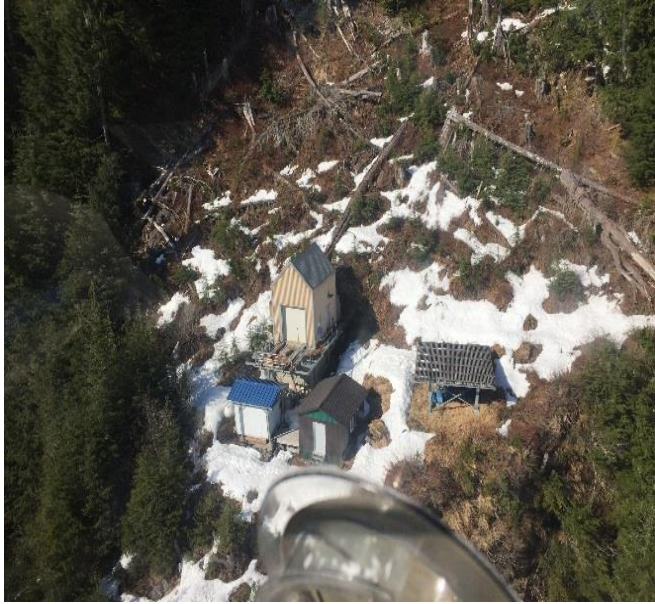
Tyee Lake Intake Gatehouse
