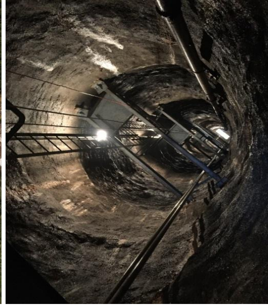
Tyee Lake Intake Gate Shaft
