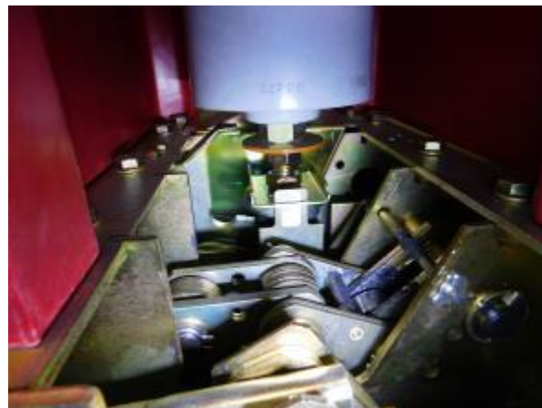
Unit #2 A-Phase interrupter indicator
