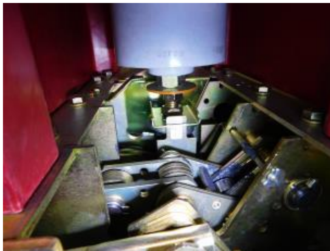
Unit #1 A-Phase interrupter indicator
