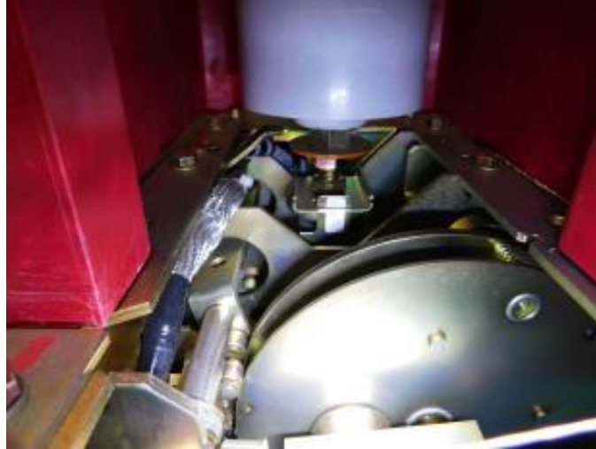
Unit #1 C-Phase interrupter indicator
