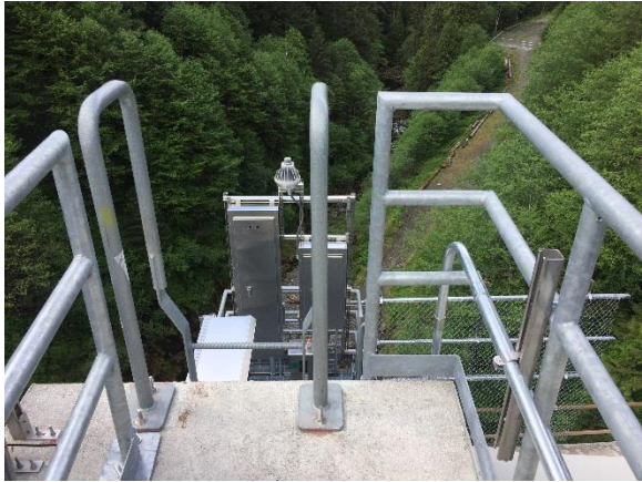
North Pier Top Handrail
