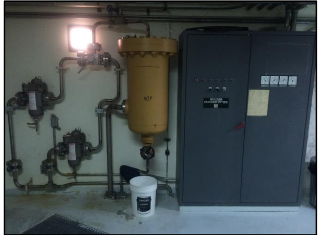
Filter system to left of control cabinet
