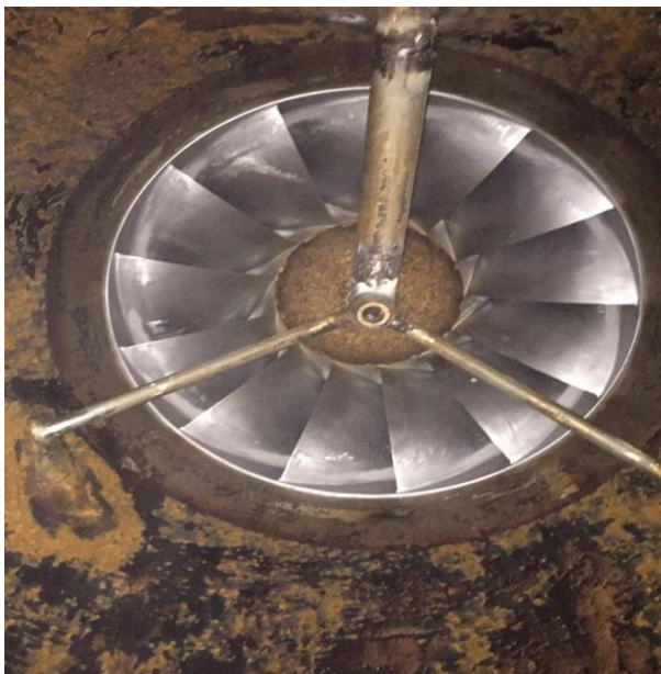
View of Runner from Draft Tube
