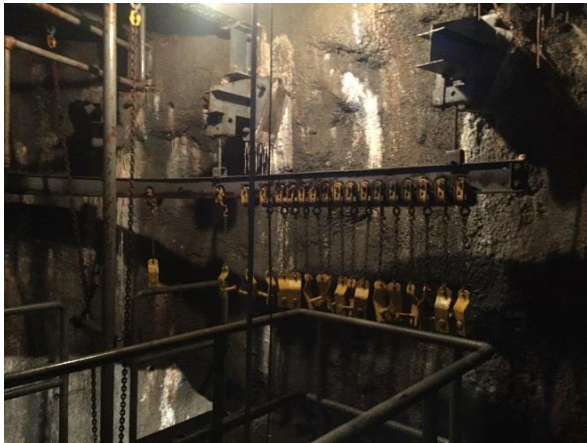
Lift Cylinder Stem Rack El. 1432.0'
