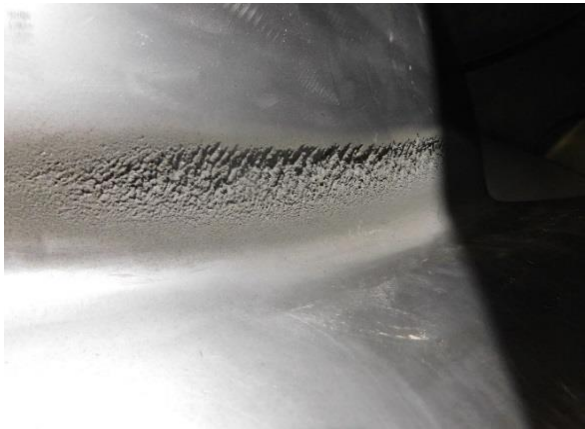
SWL Runner Cavitation Damage
