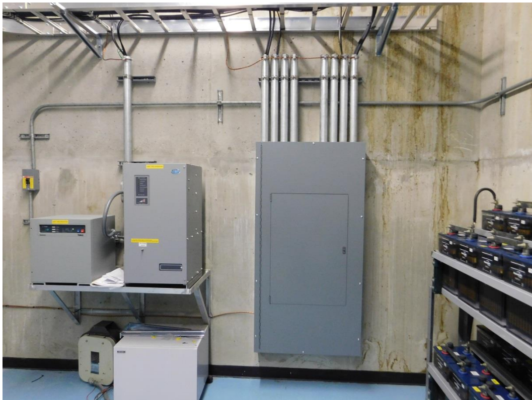
Above photo: Continuation of the DC Distribution System Upgrade
