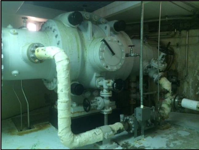
Unit #1 TSV, by-pass pipe and valve, control cabinet and filter on floor above
