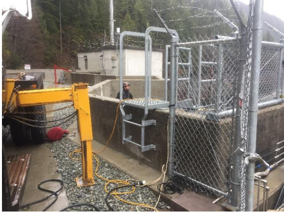
North Abutment Reservoir Access Ladder
