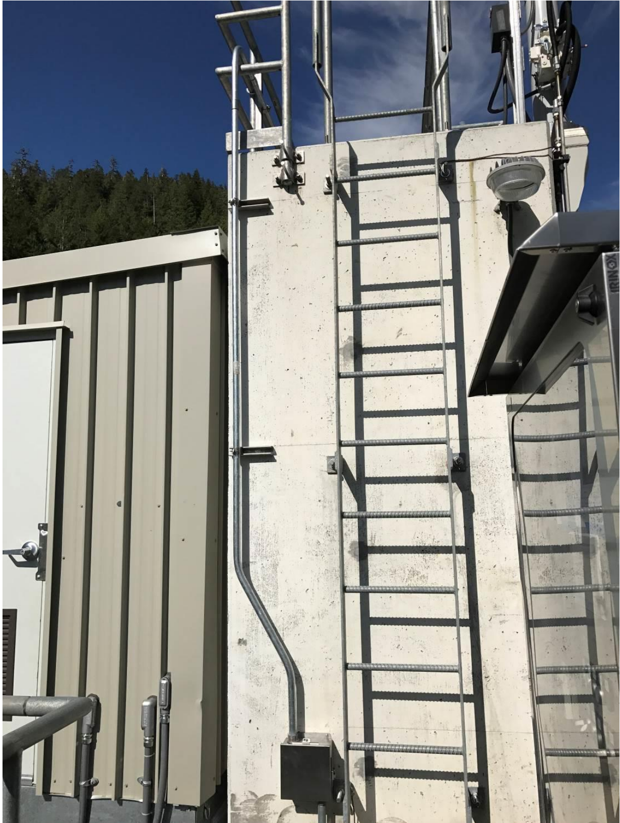
Above photo: new ladder and hand rails to top of Dam structure
