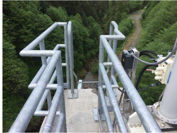
Center Pier Top Handrail
