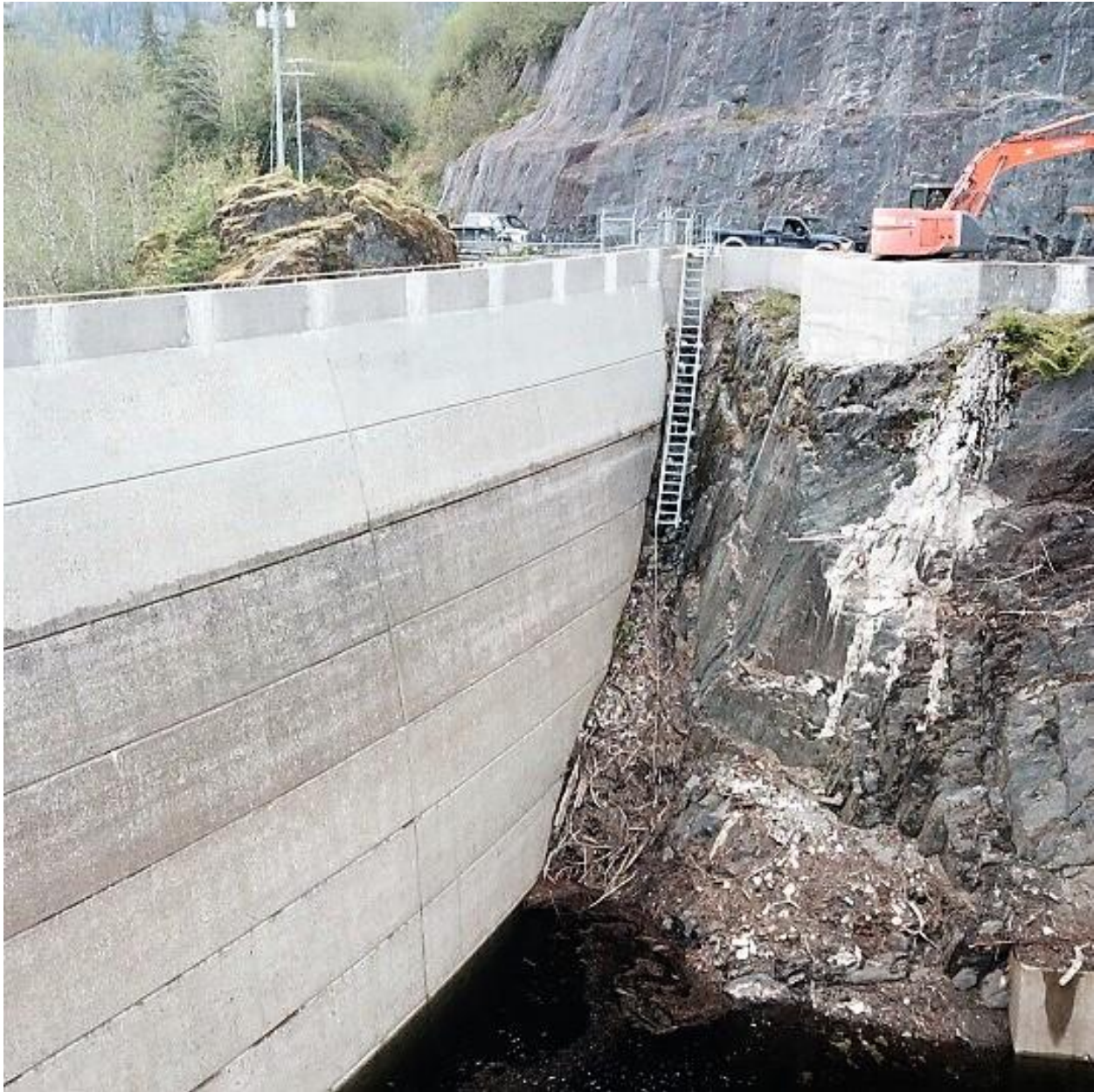
Above photo: Ladder fabrication and install by BAM along Dam abutments
