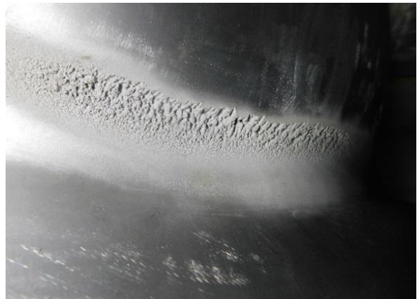
SWL Runner Cavitation Damage
