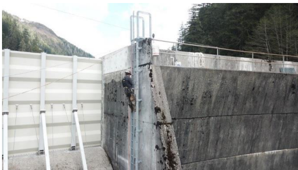
Swan Lake Spillway Access Ladder
