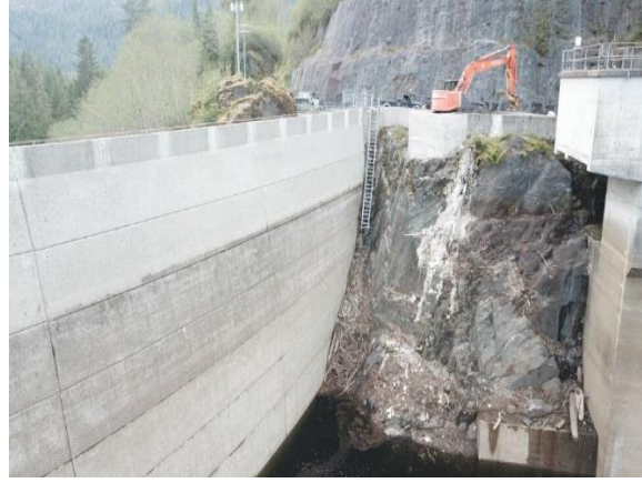
North Abutment Reservoir Access Ladder
