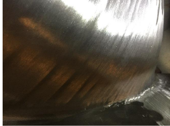
Runner Blade after Repair
