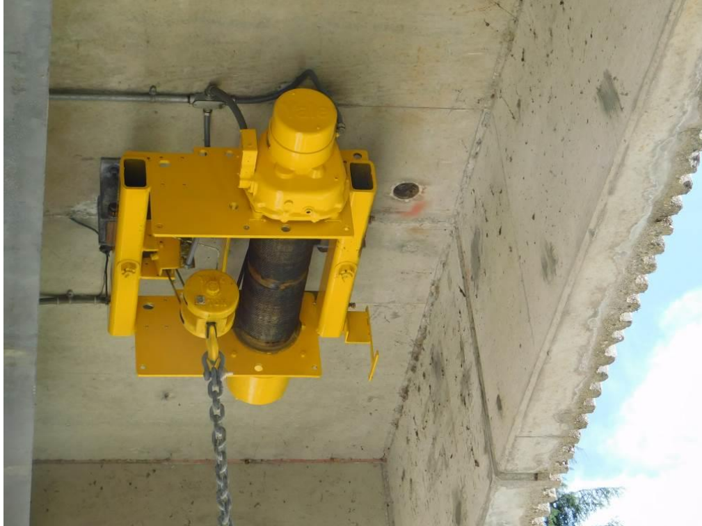
Above photo: Winch PMs and chain replacement for Draft Tube Stop Logs (gates)
