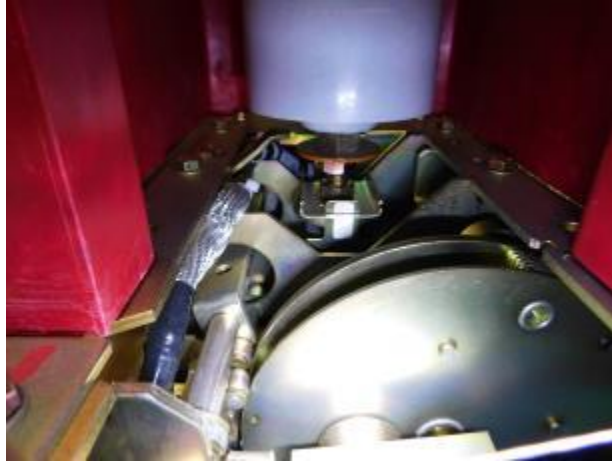
Unit #2 C-Phase interrupter indicator
