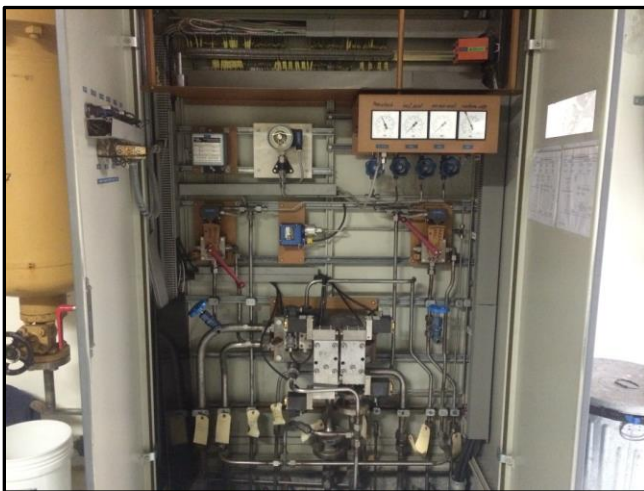
Control valves, timers and switches internal to cabinet
