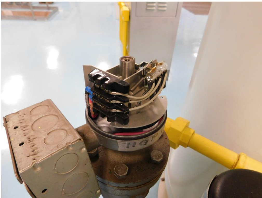
Photo Below: Governor Oil pressure switch service
