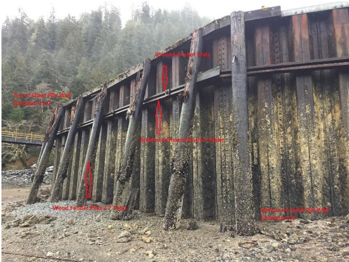
Swan Lake Marine Bulkhead (2017 photo)
