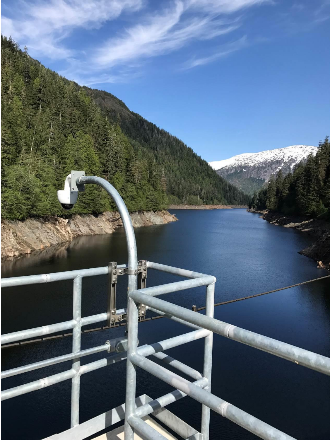
Above photo: New hand railing provides a perfect place for a security camera install
