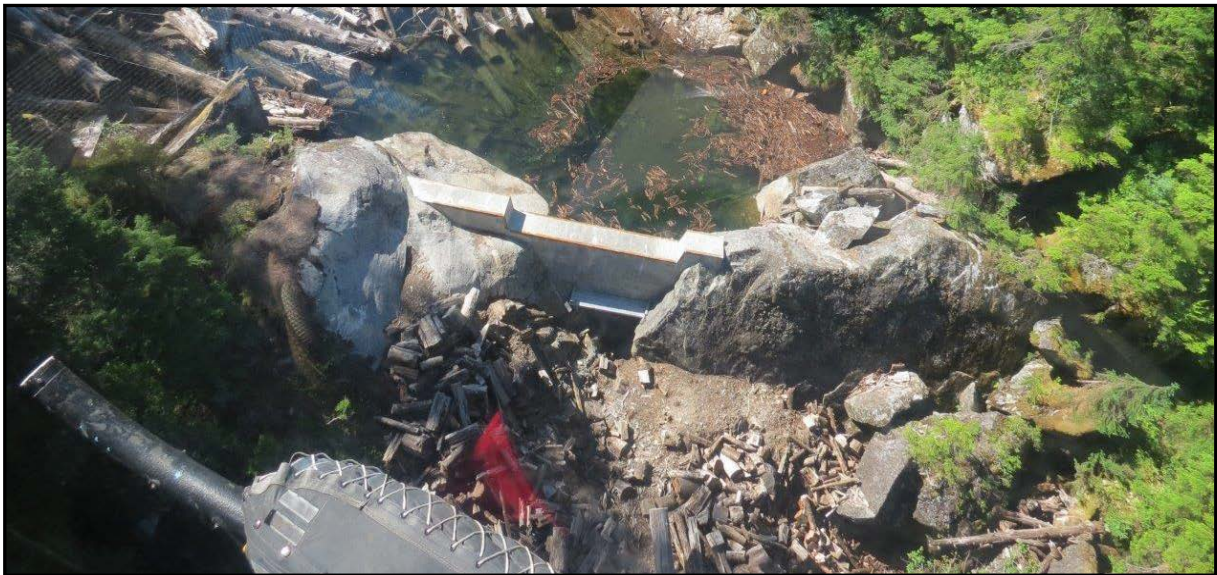
Photos of Tye outlet from Summer of 2014; water surface elevation approximately 1395 ft.; leakage occurring at and under the right abutment
