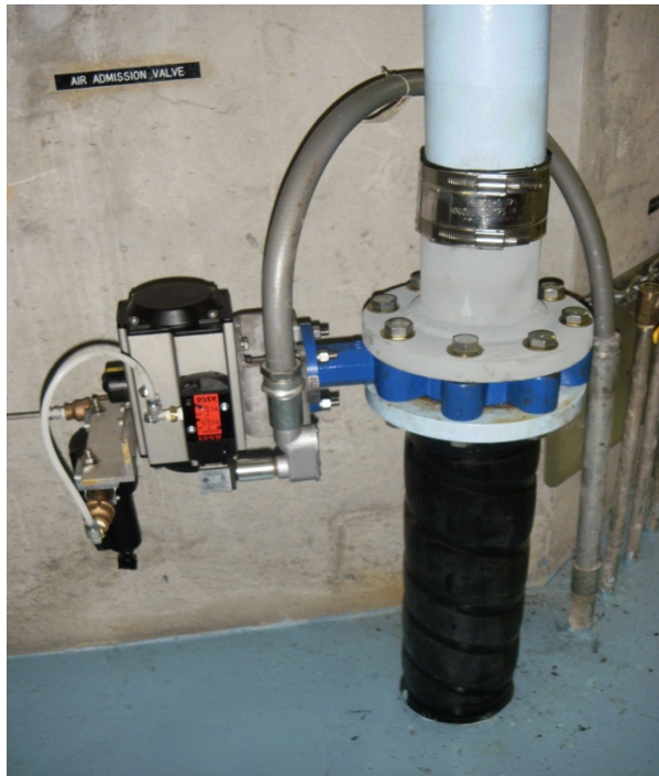
Air admission valve & actuator
