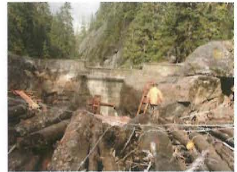
(Tye weir, upstream side)
