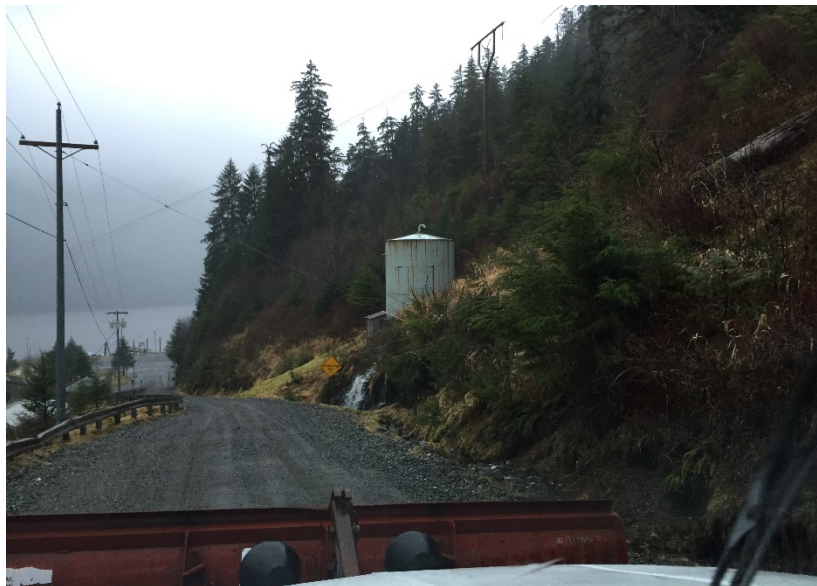
Swan Lake Water Tank
