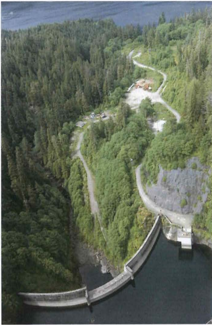
Swan Lake Aerial View (Intake Structure to Right)
