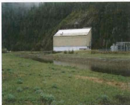
Tyee Lake Power House
