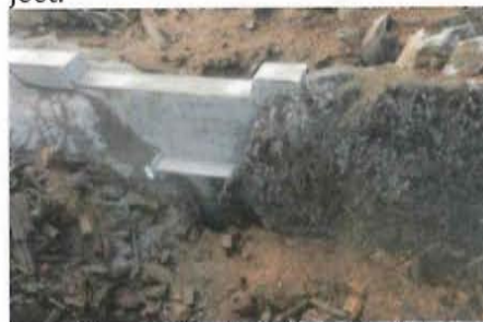
(Tye weir, downstream side)
