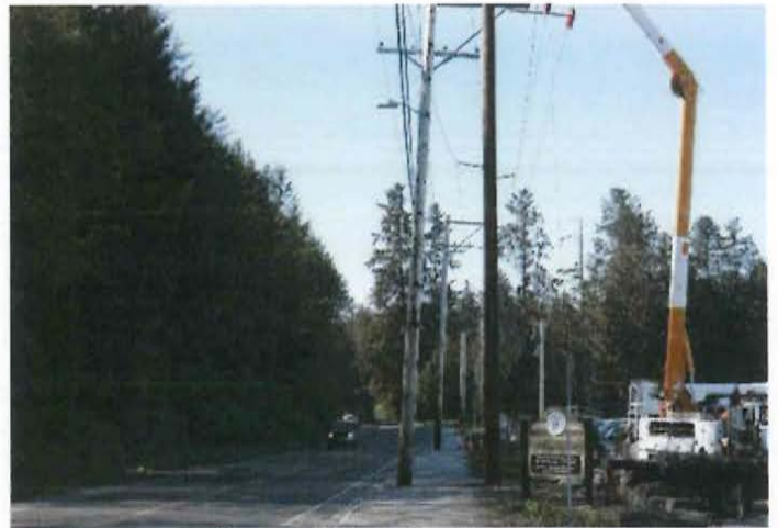
Wrangell Pole Realignment
