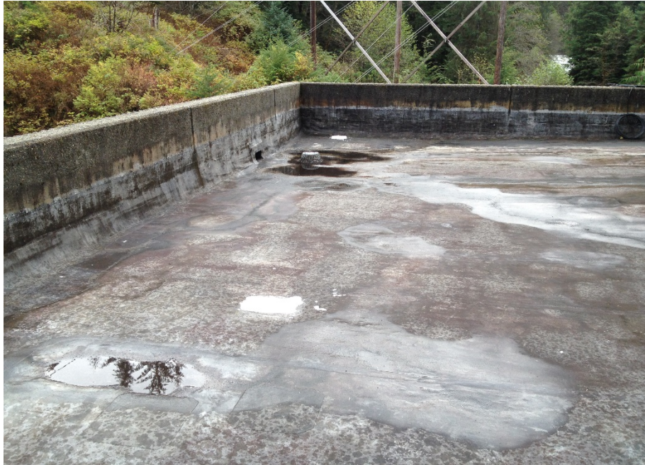
Swan Lake Powerhouse Roof
