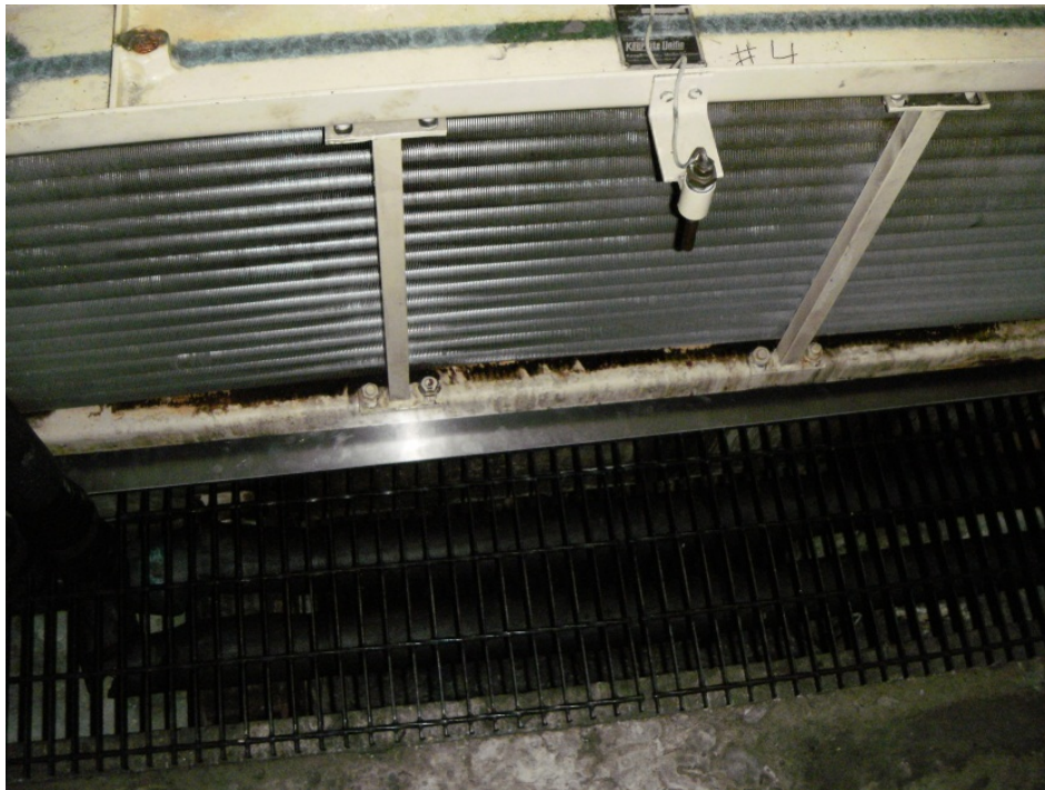
Drip pan under cooler
