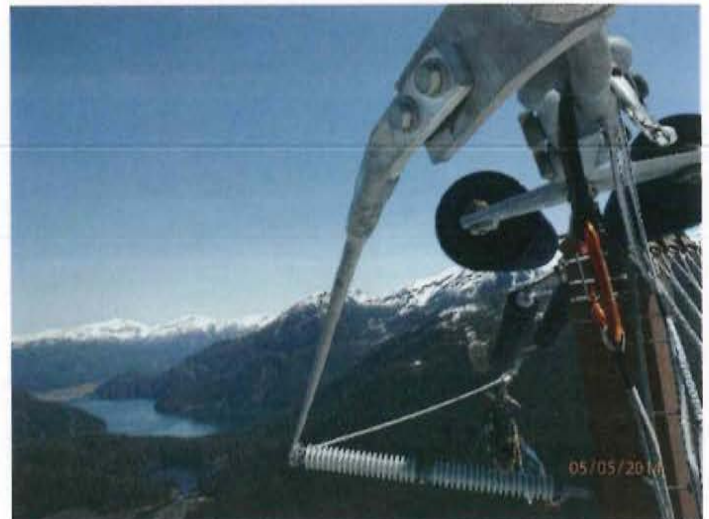
Look close and you'll see a line maintenance worker!
