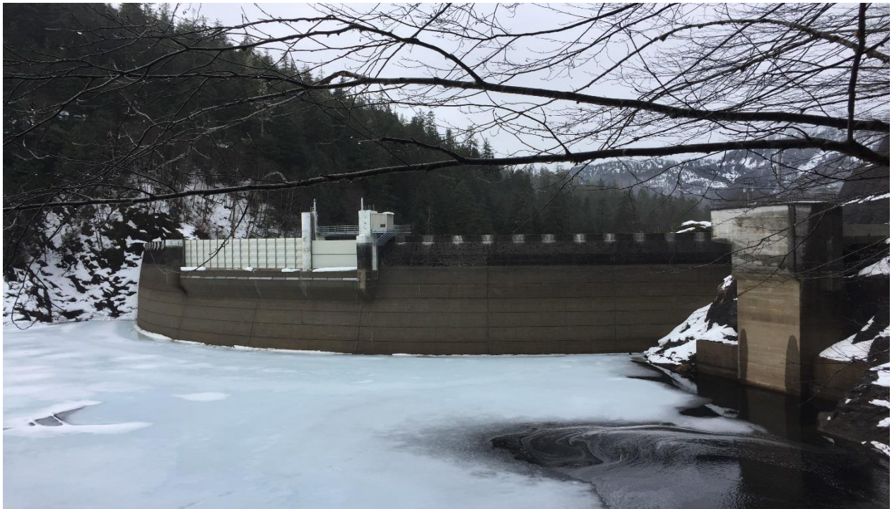
Swan Lake Dam with New Flood Control Gates / Reservoir Elevation 285.4'
