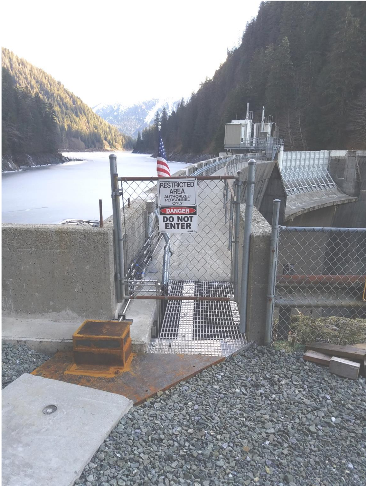
Above: Gate installed for gangway access to dam gate & compressor equipment
