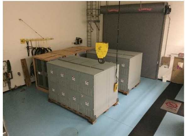
Replacement Exciter and Breaker Cabinets
