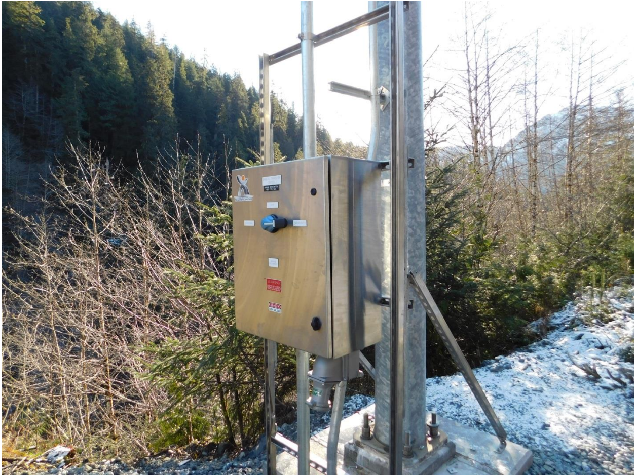
Above: Emergency Gate House Generator Transfer Switch
