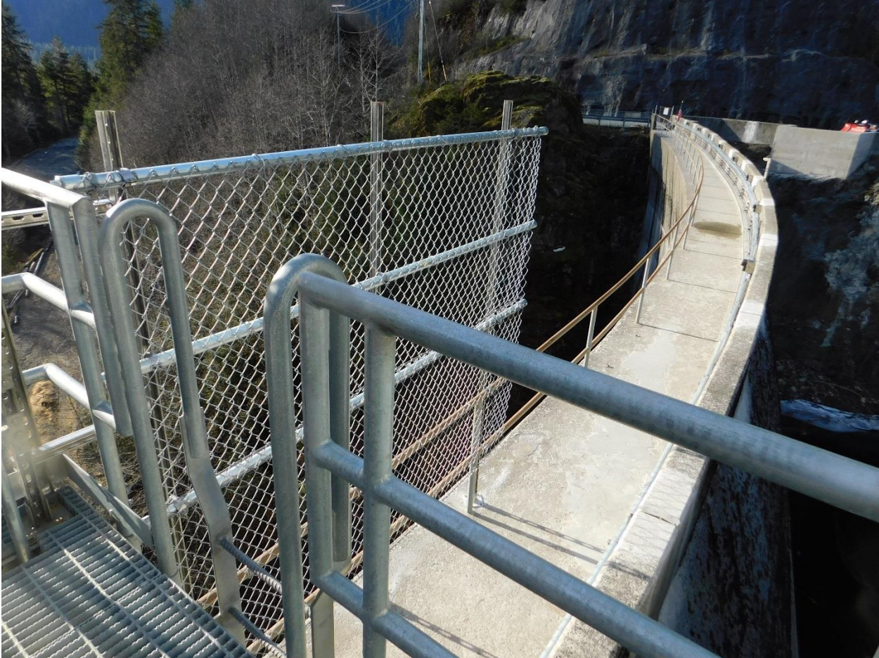
Below: protective fence/ guards
