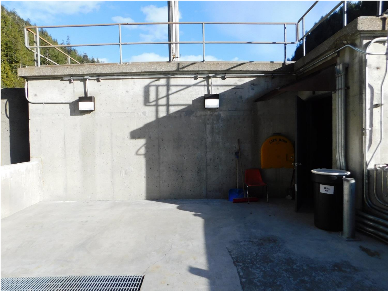
Below: Conduit and yard lights installed at Gate House
