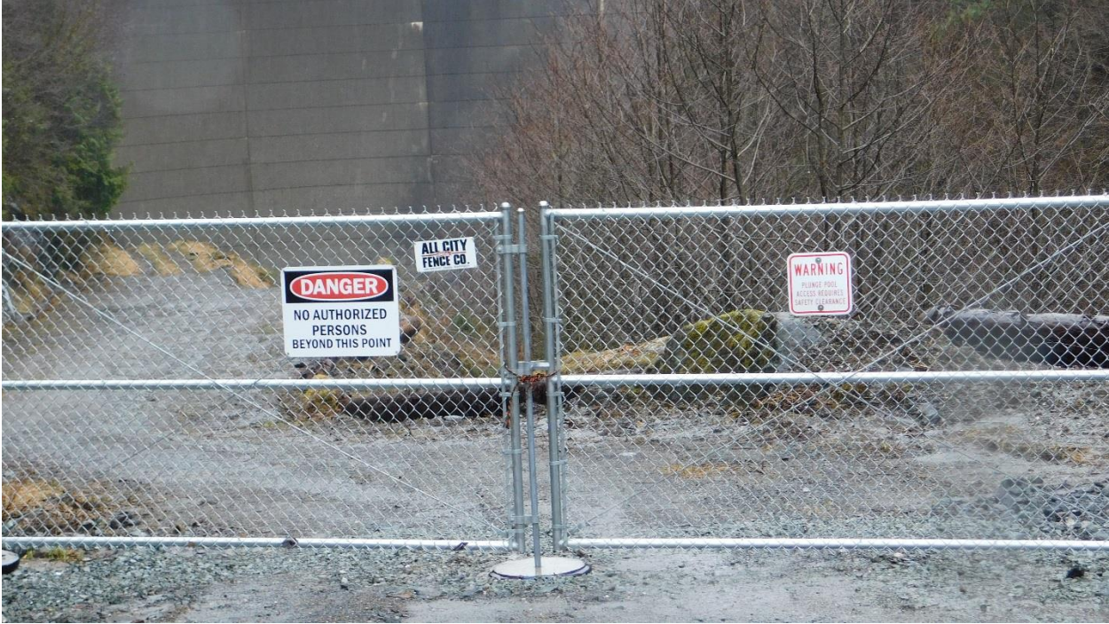
Above: New fencing and signage to secure the plunge pool area
