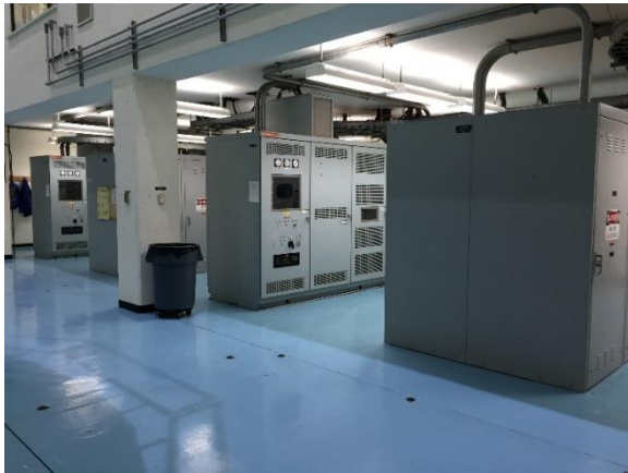
Existing Exciter and Breaker Cabinets
