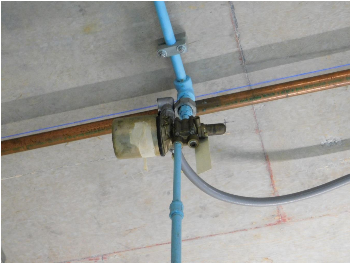
Above: Governor compressor air solenoid valve
