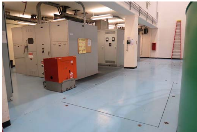
Unit 2 Generator Breaker Racked Out
