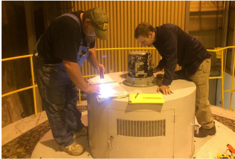
SEAPA's Chris Barnett and Segrity LLC's James Volk inspecting the Governor over-speed switch (part of the protection review).
