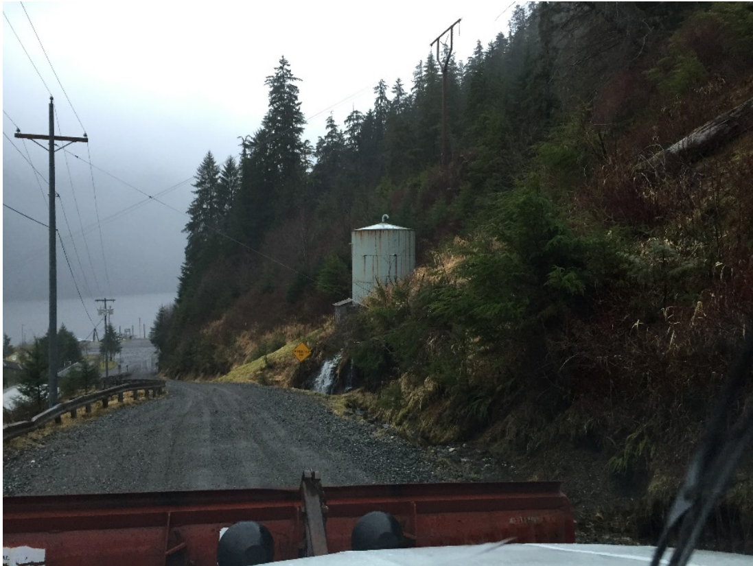
Swan Lake Water Tank
