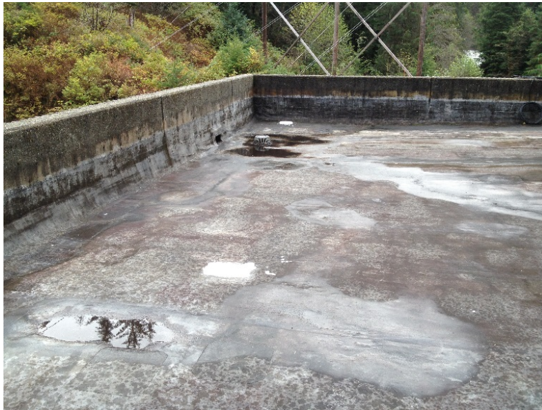
Photo of existing Swan Lake Powerhouse Roof
