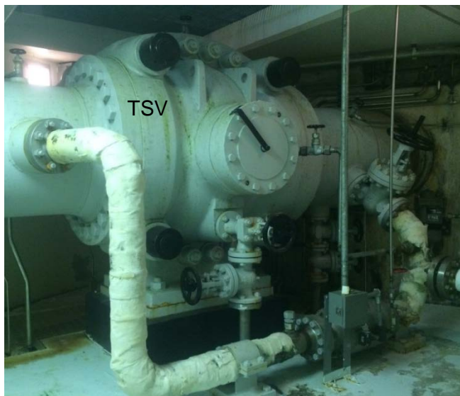
Tyee Turbine Spherical Valve and smaller bypass on the lower pipe; the turbine inlet is on the left side of TSV; the penstock is on the right side (upstream).
