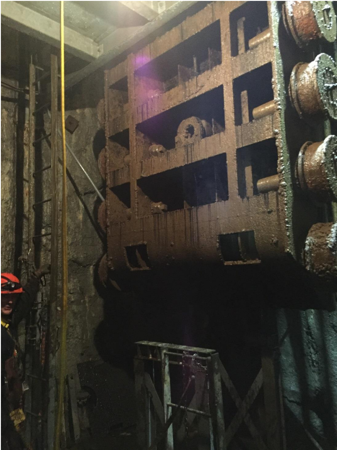
Tye intake gate pulled for inspection July 2018.
