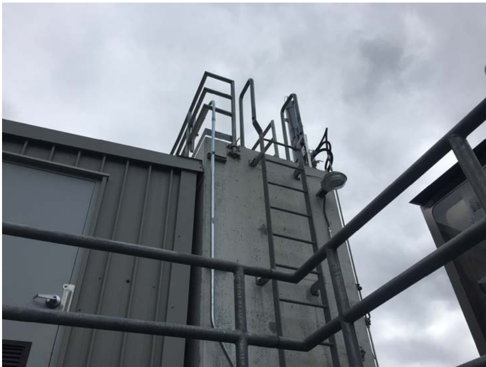
Handrail on Top of the North Pier
