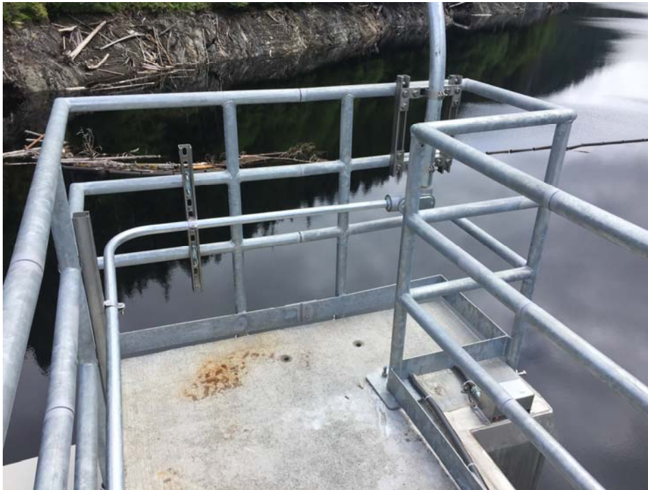
Handrail on the top of the Middle Pier
