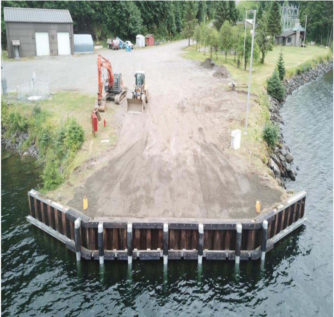
Completed Swan Lake Marine Bulkhead
