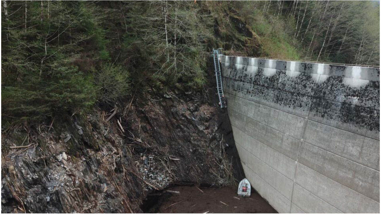
South Dam Abutment Access Ladder
