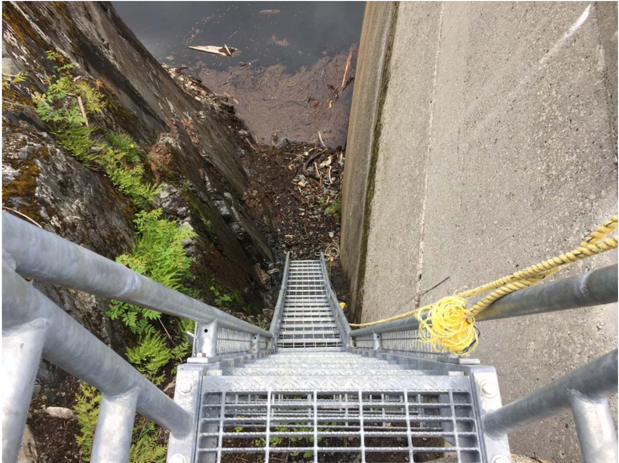
Reservoir Access Ladder North Dam Abutment
