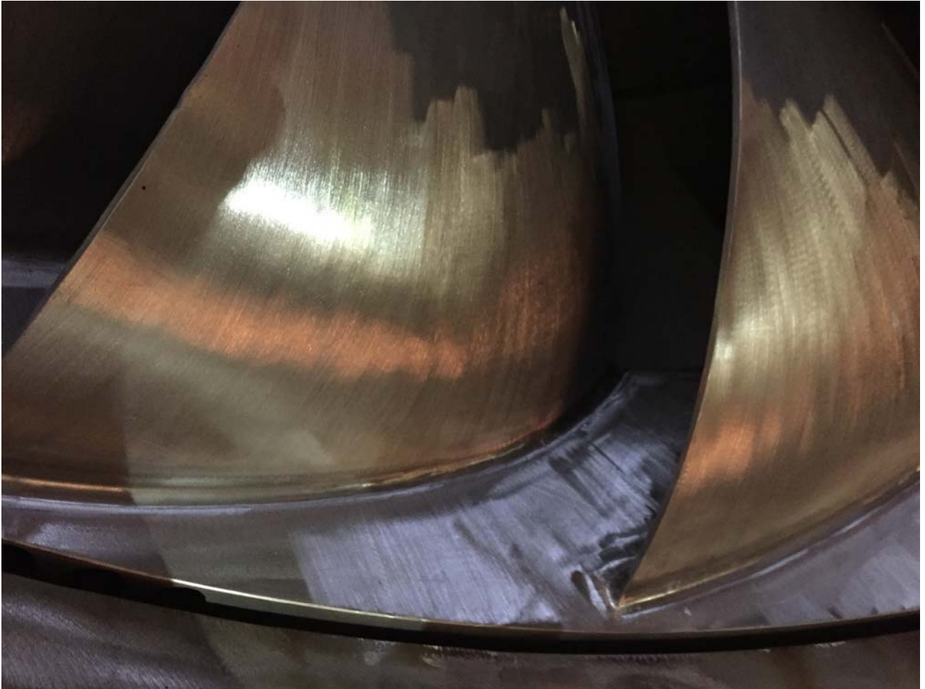
Swan Lake Completed Runner Welding Repair
