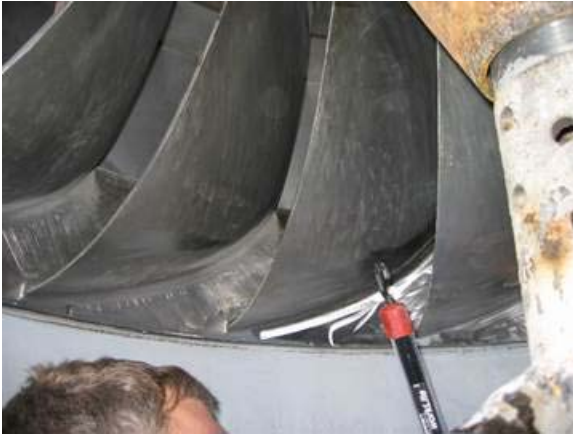
Runner cavitation monitoring inspection
