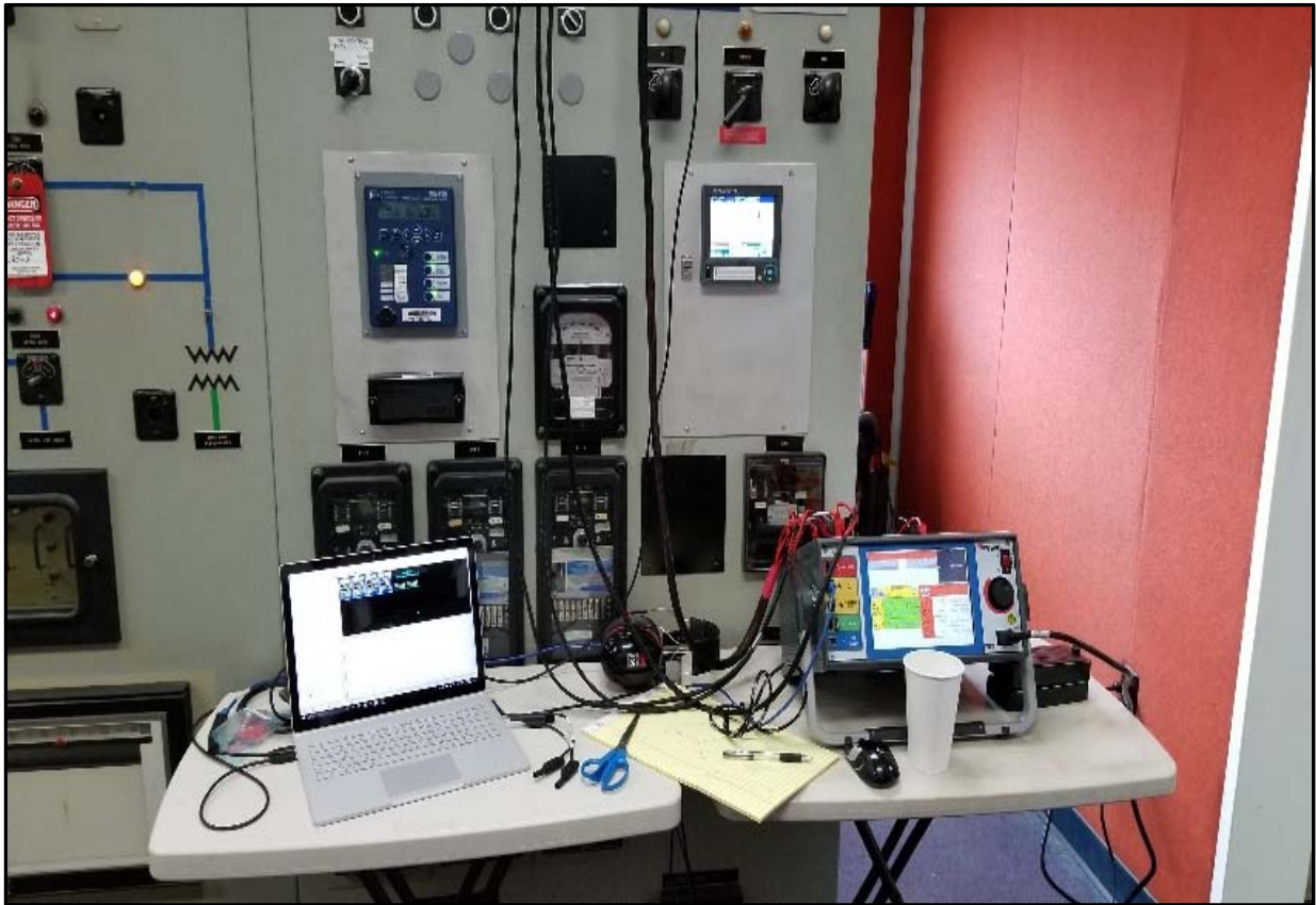
Bailey 311C Line Differential Testing
