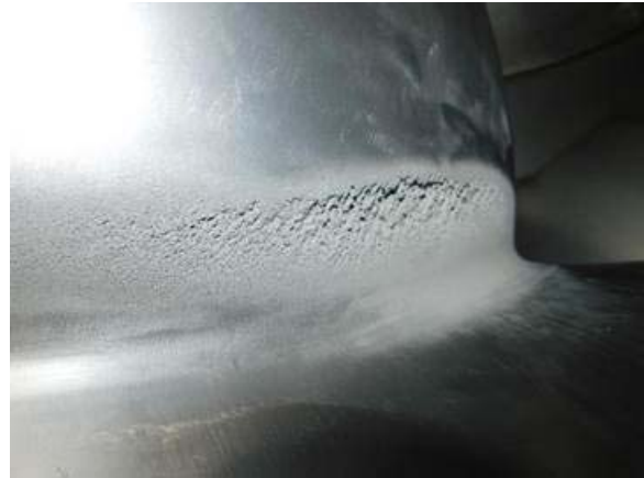
Closer view of runner cavitation damage
