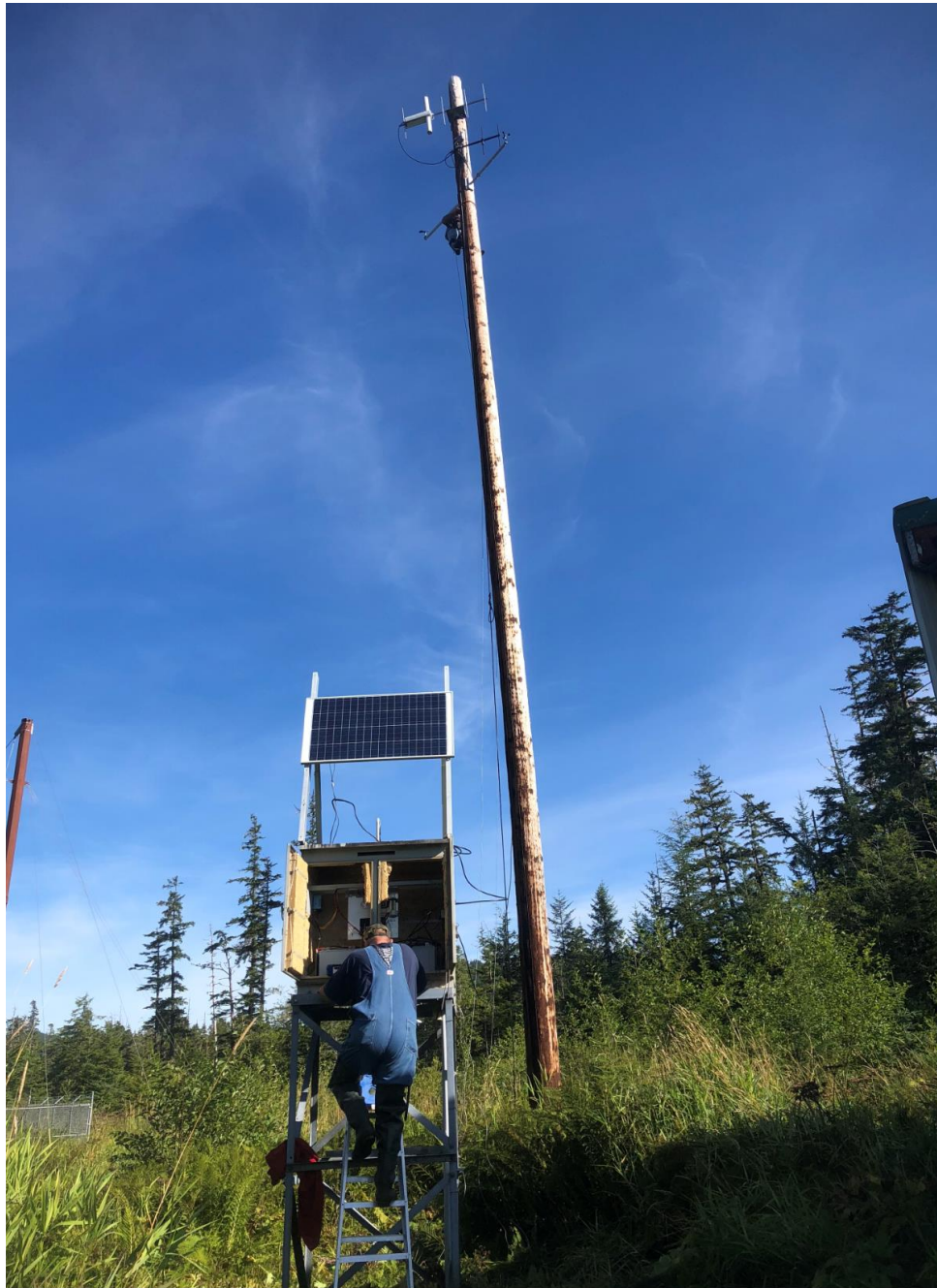
Tyee electrician, Chris Barnett, installing data collection module while Brushing Foreman, Robert Robbins, installs weather vane and anemometer on pole.
