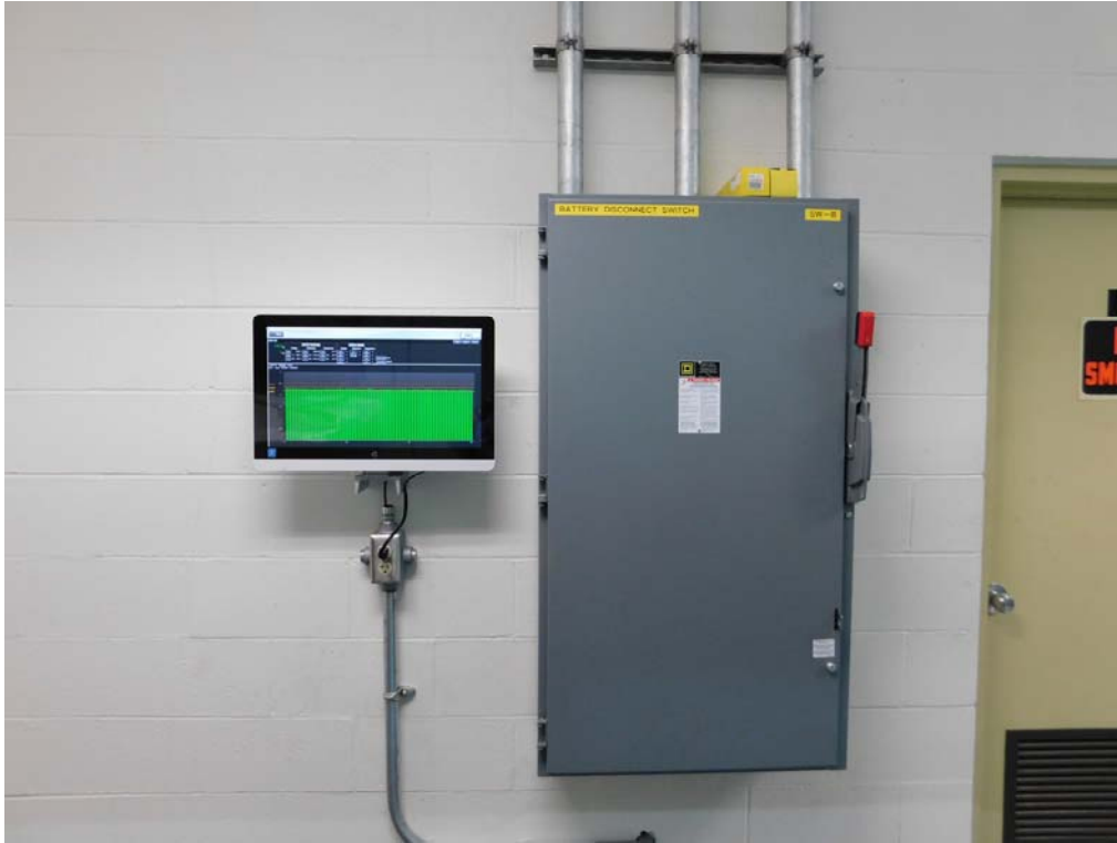
Swan Lake: Installed Battery Monitor System with HMI
