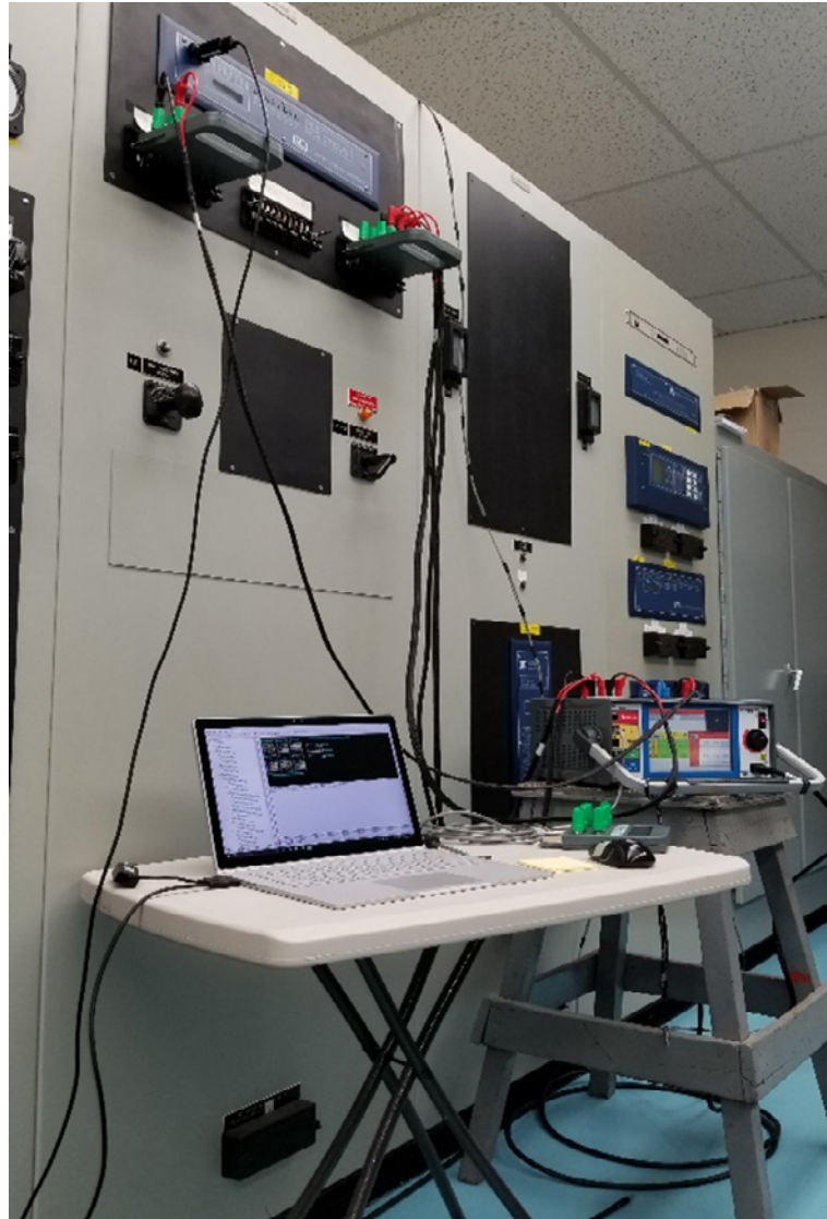
Swan Lake 387E Transformer Differential Testing
