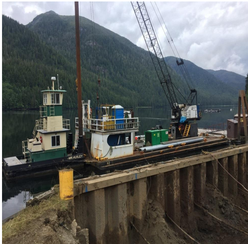
Swan Lake Marine Bulkhead Ground Anchor Excavation
