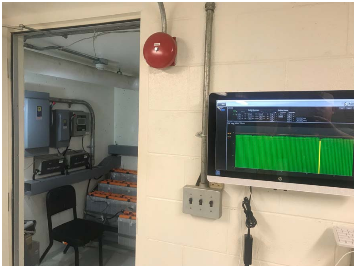
Tye Lake: Installed Battery Monitor System with HMI
