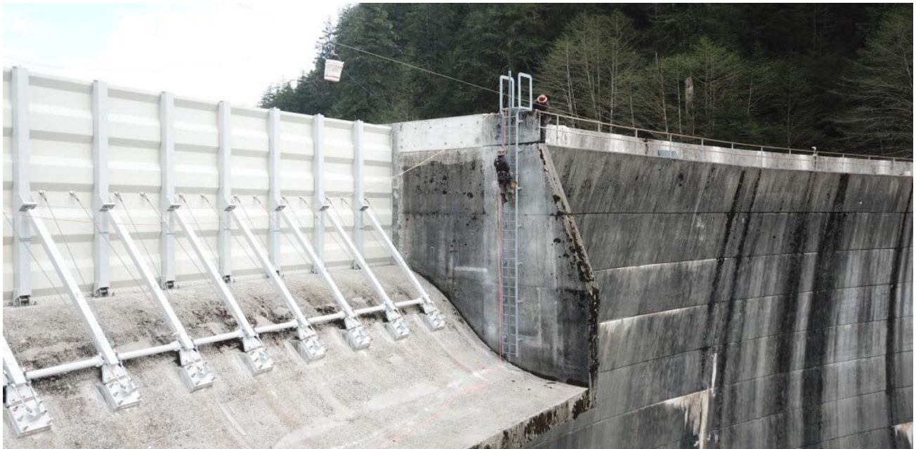
Spillway Access Ladder
