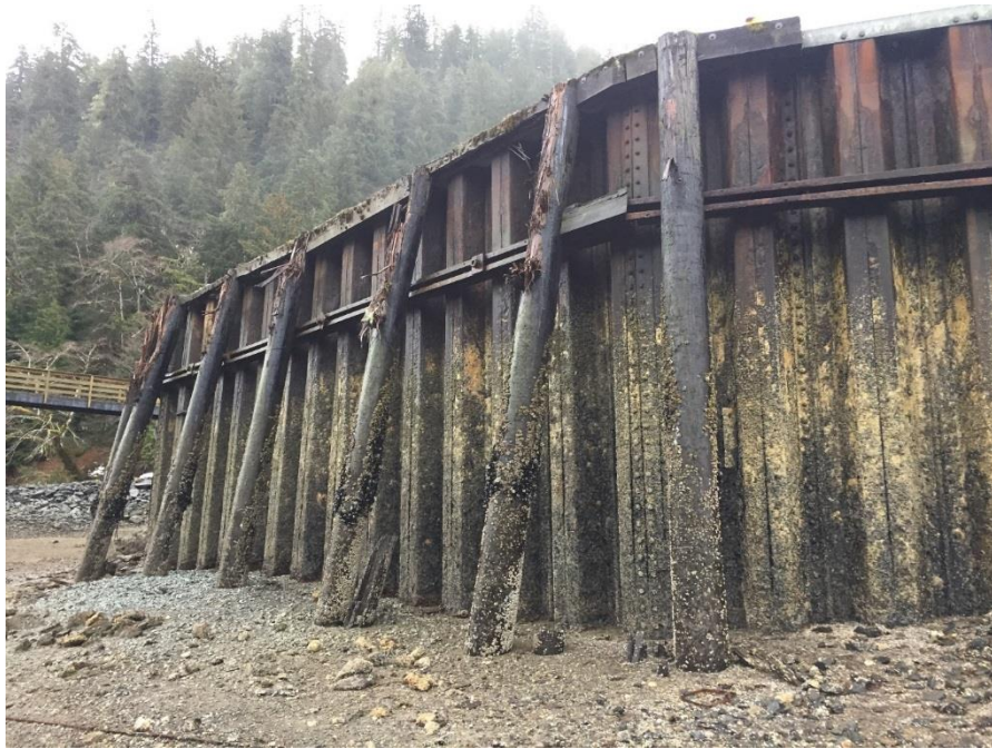
Swan Lake Marine Bulkhead prior to restoration.
