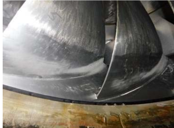
Typical cavitation damage appears as light gray areas on the runner (known as frosting)
