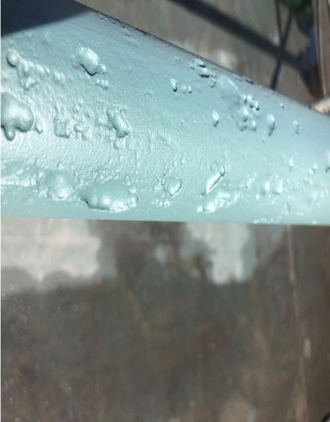
Gate stem rust damage found during sandblasting.
