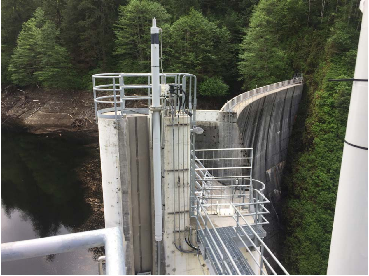
Flash Board Gate Trigger Guard & Middle Pier Top Handrail
