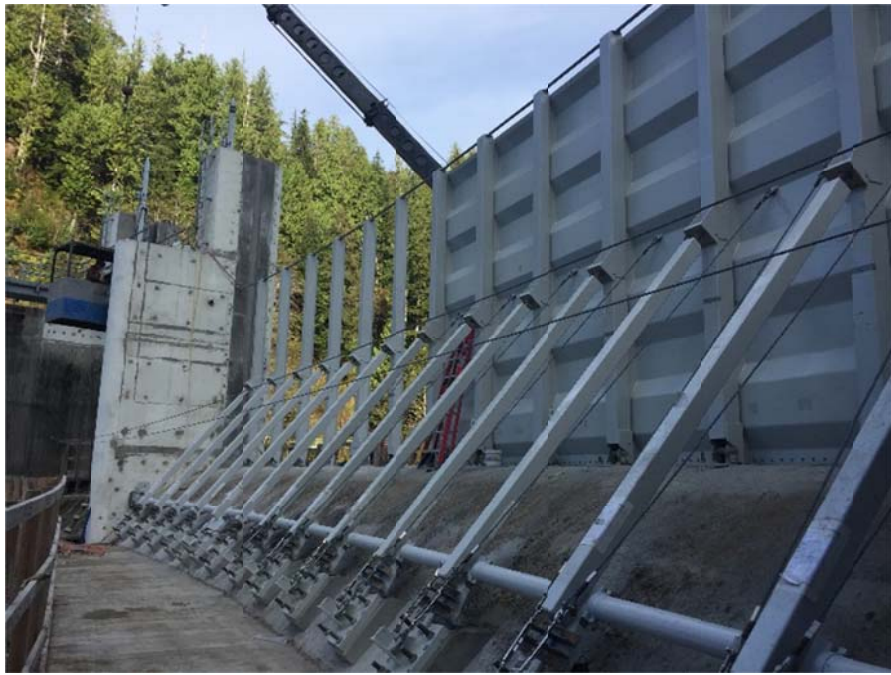
Flash Board Gate Installation
