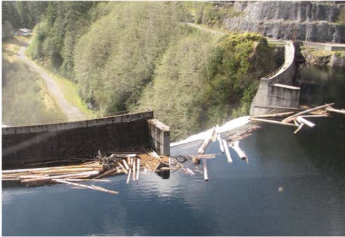
Figure 1 - Swan Lake Spillway, May, 2015
