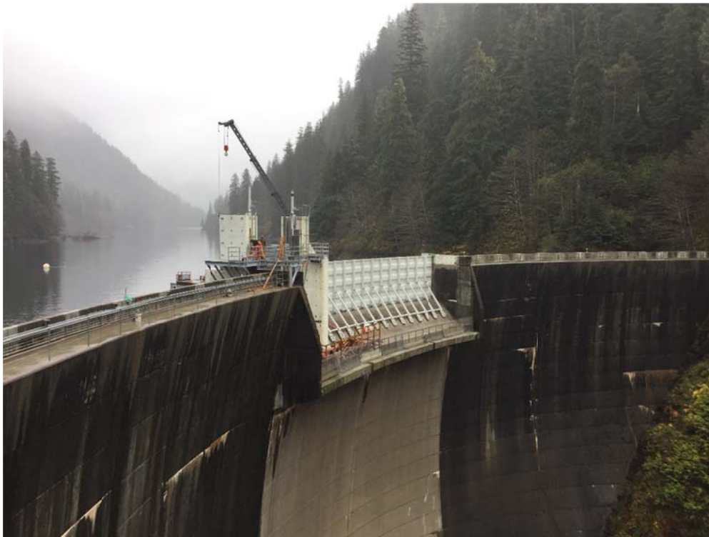
Installation Complete for all Spillway Structural Components
