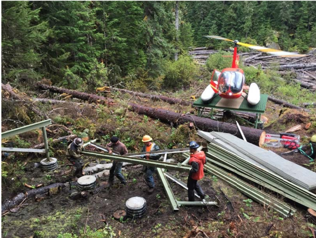
Reassembly of Emergency Shelter Foundation
