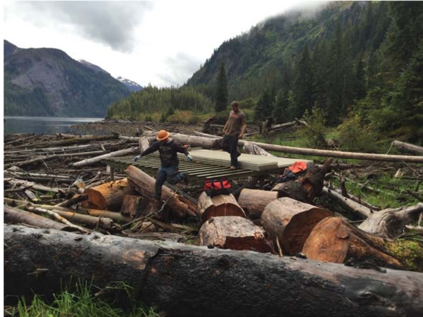
Disassembly of the Existing Helicopter Pad and Preparation for Transport by Helicopter
