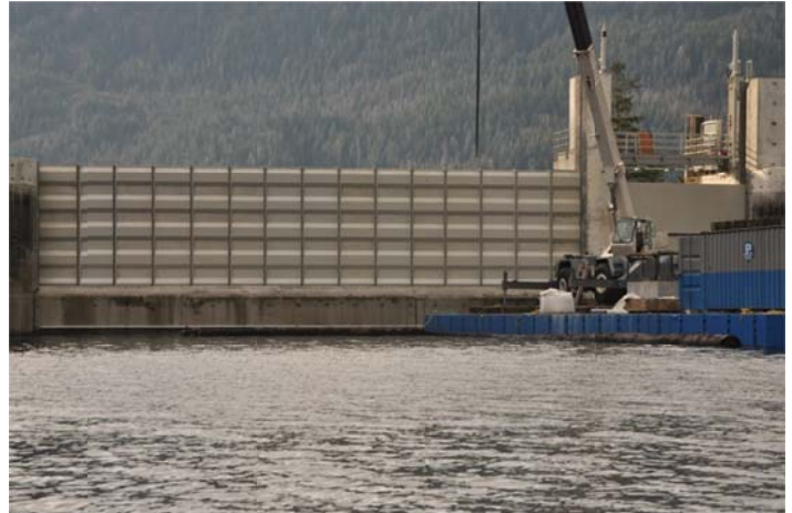
Figure 2 - Swan Lake Spillway, October, 2016
