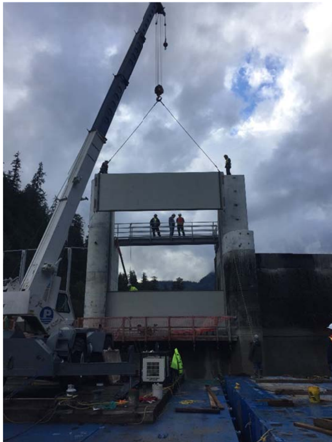
Installing Second Section of Fixed Wheel Gate
