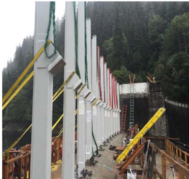
Flash Boards Columns Installed
