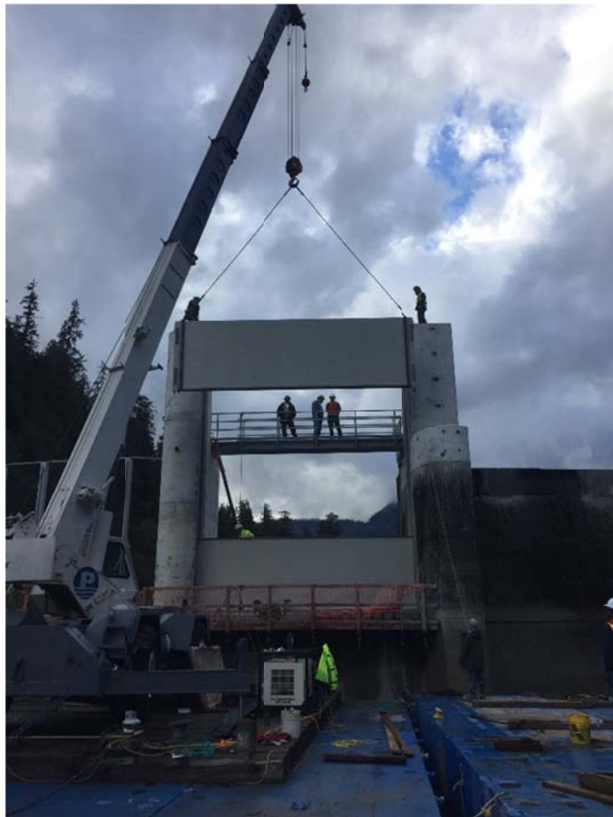
Installing Second Section of Fixed Wheel Gate
