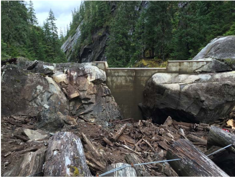
Tyee Lake Outlet Discharge Measurement Weir
