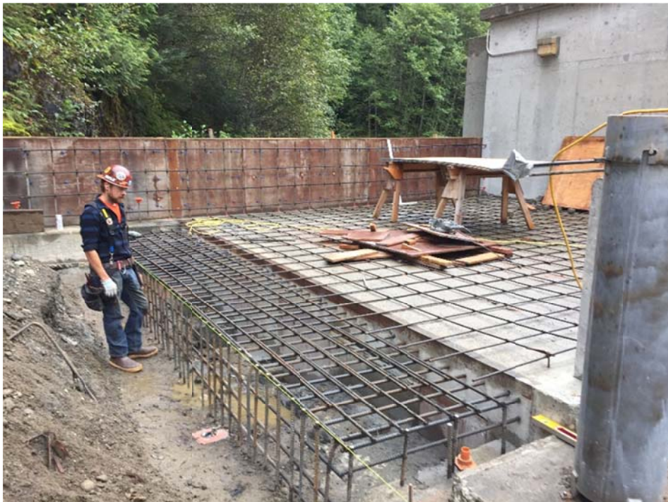
Intake Building Bulkhead, Parapet Wall & Apron Slab Reinforcement Steel Installation
