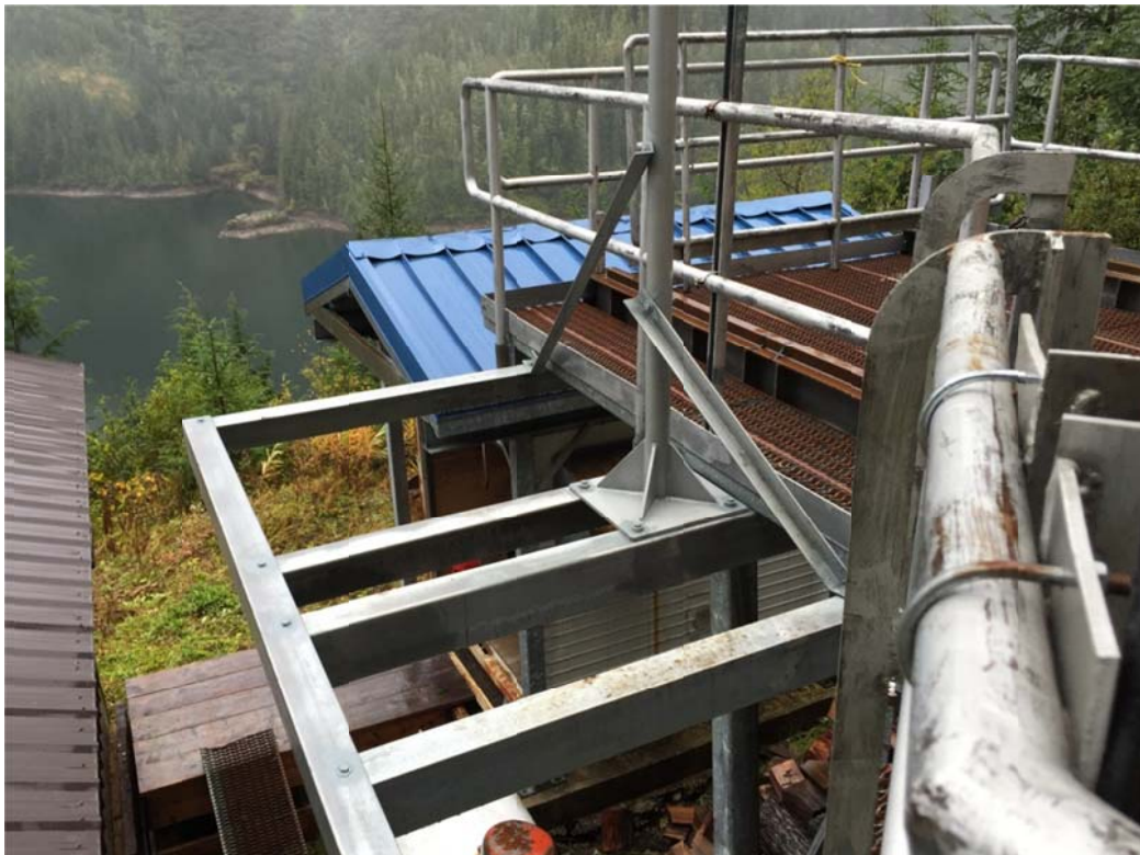
Satellite Bracket Complete & Ready for Dish Installation
