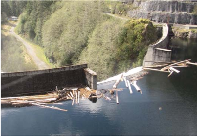
Figure 1 - Swan Lake Spillway, May, 2015
