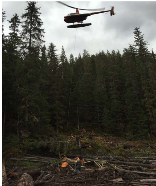
Lifting Disassembled Helicopter Pad Sections to Emergency Shelter Location
