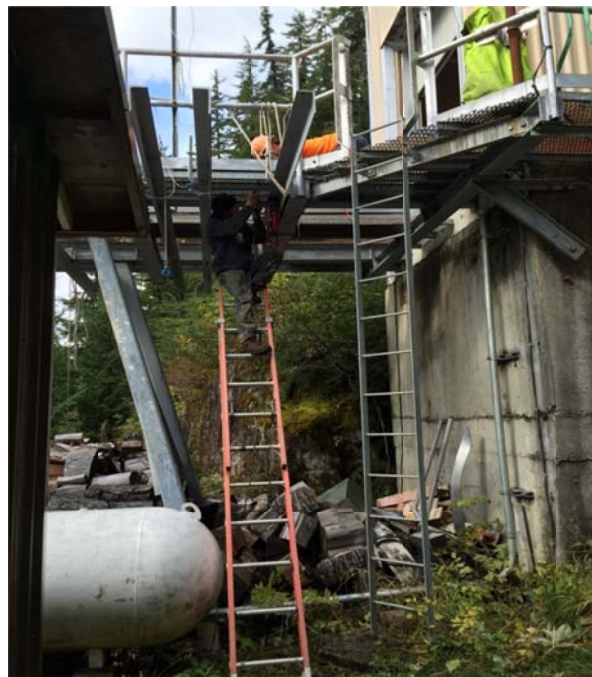
Installing Bracket to Tyee Lake Intake Gate Building
