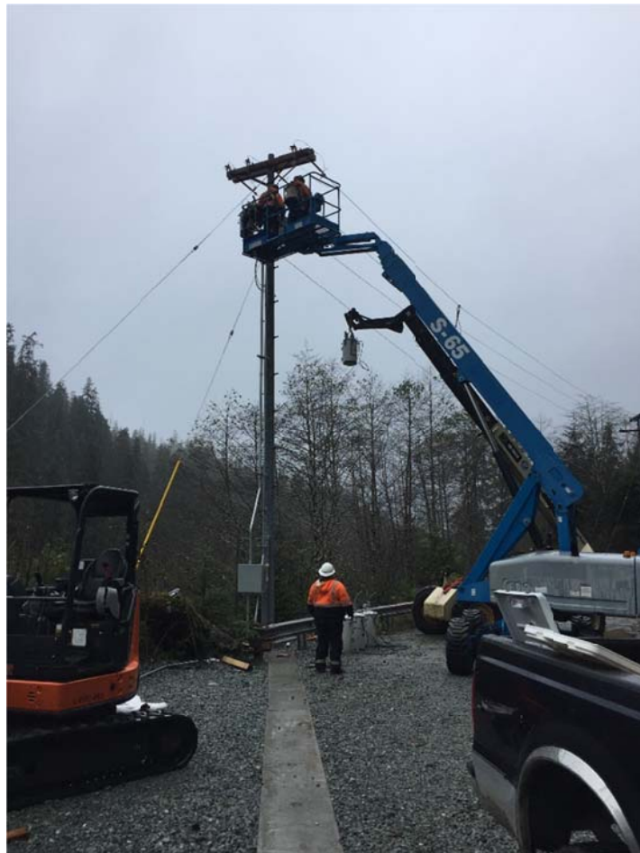
Intake Building Transformer Installation
