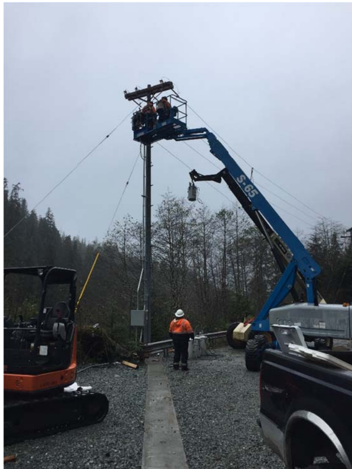
Intake Building Transformer Installation
