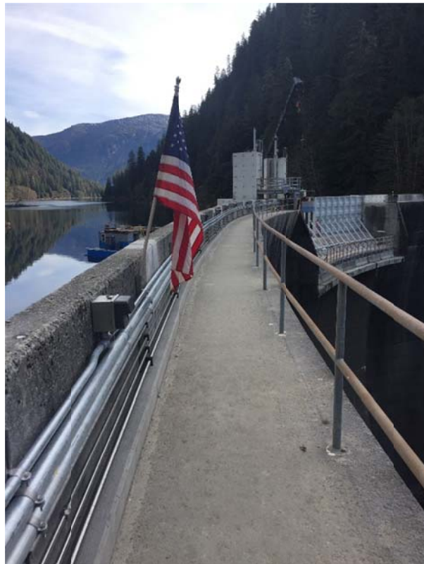
Electrical & Hydraulic Installation to Dam Spillway
