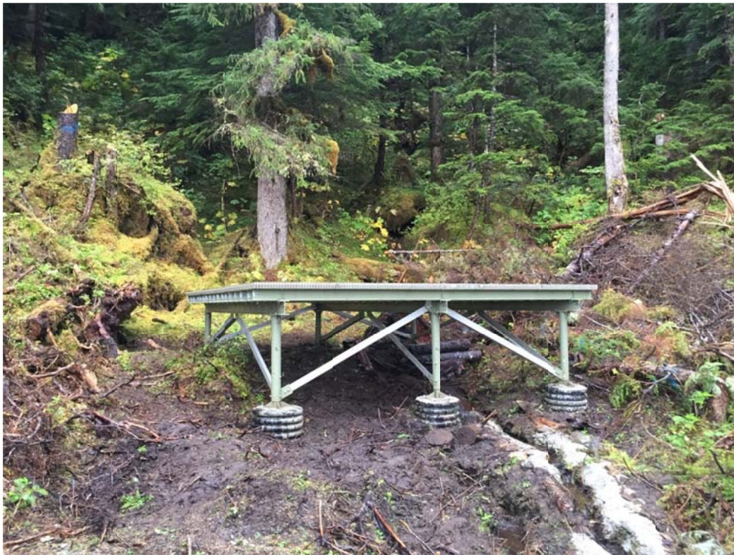
Emergency Shelter Foundation Complete
