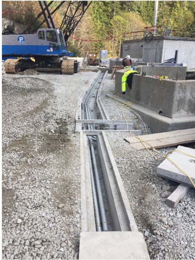
Installation of Intake Building Electrical & Hydraulic Corridor
