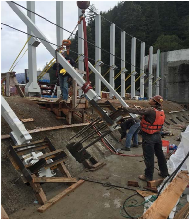
Column Kicker & Anchors Installation
