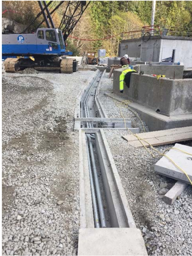
Installation of Intake Building Electrical & Hydraulic Corridor
