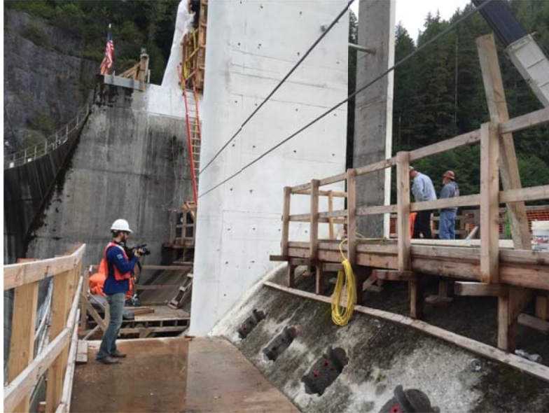
KPU TV Filming At Swan Lake Dam Spillway
