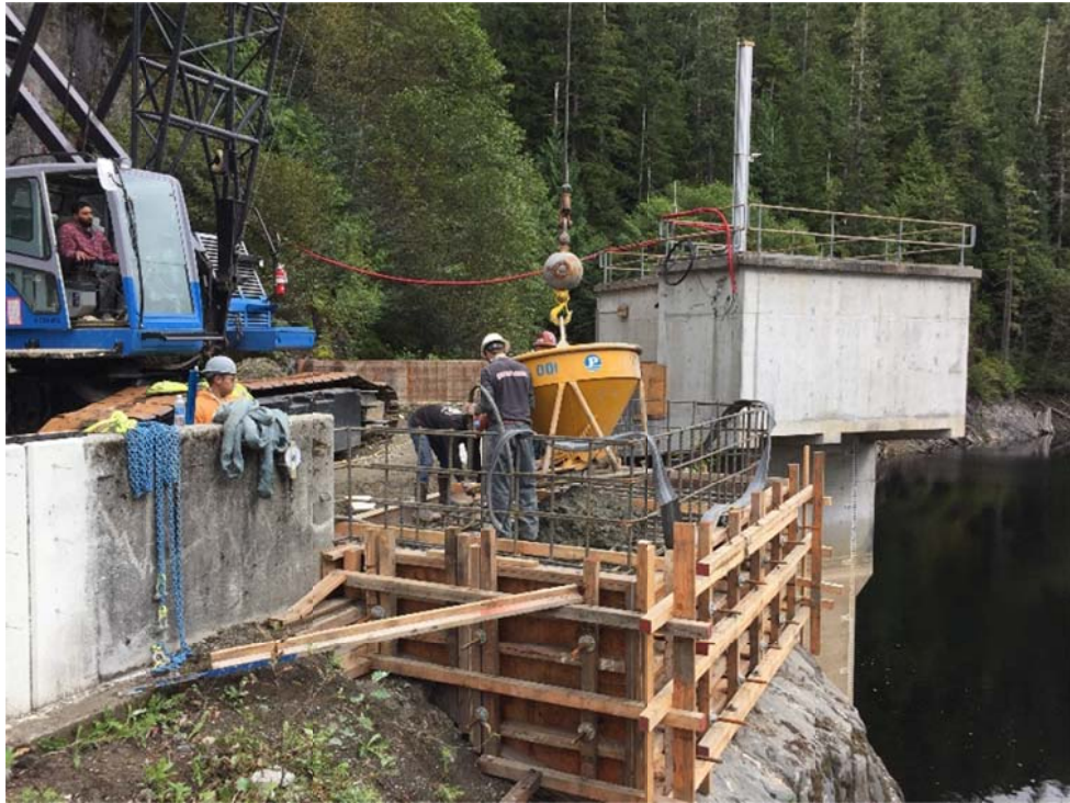
New Lake Debris Slab & Parapet Wall Installation
