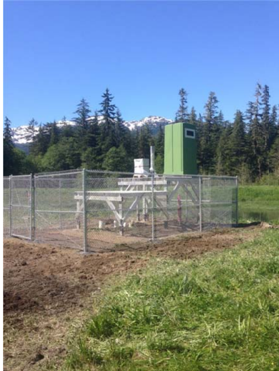
Tyee satellite platform has been installed by Alaska Clearing.
