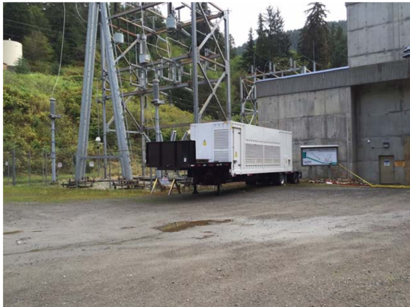
Crestchic 5 MW Load Bank at Swan Lake
