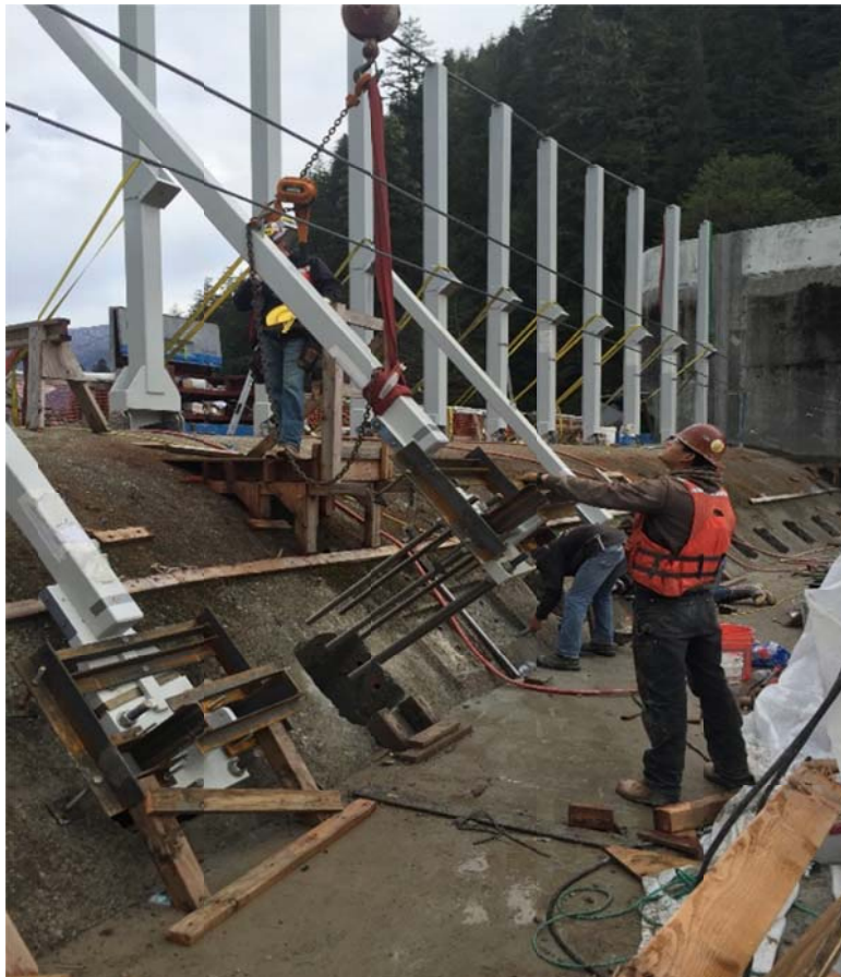
Column Kicker & Anchors Installation
