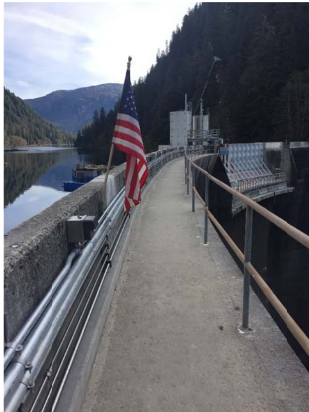
Electrical & Hydraulic Installation to Dam Spillway
