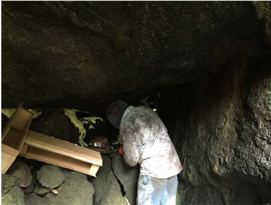
Expandable Foam Filling Voids of Right Abutment (Note Foam in Fissures) - Elevation 1380 Feet
