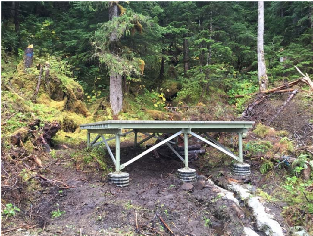
Emergency Shelter Foundation Complete
