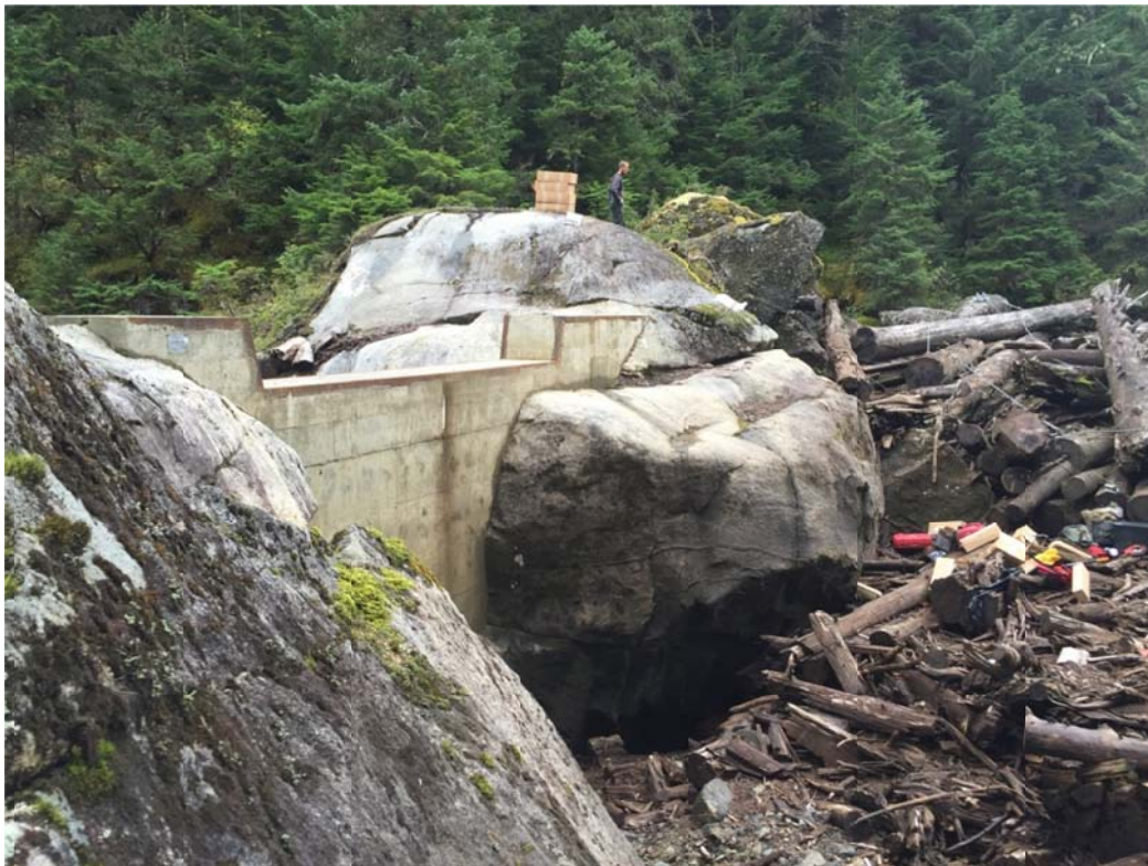
Right Abutment Upstream with Expandable Foam Boxes Staged for Placement on Downstream Side - Top of Weir Elevation 1396 Feet
