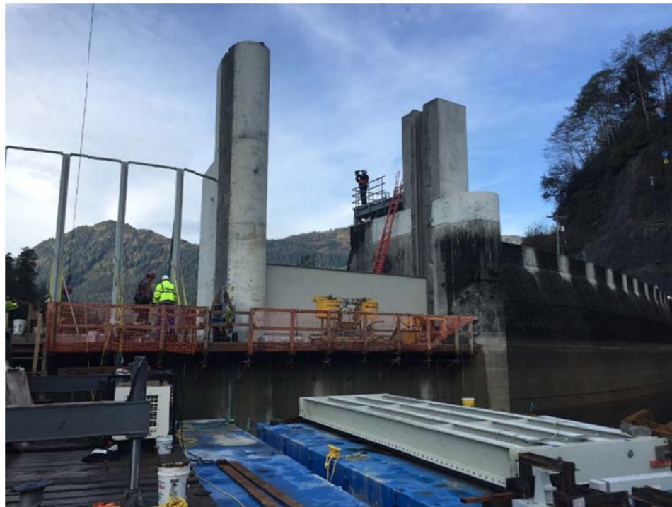
First Section of Fixed Wheel Gate Installed
