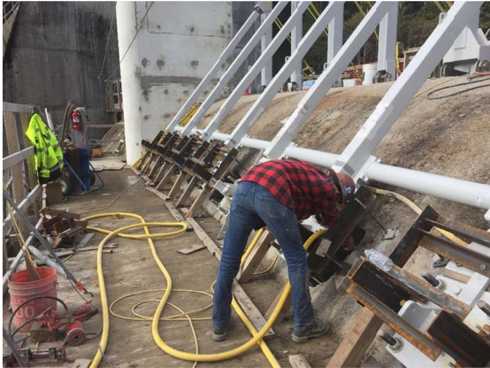
First Stage Grounding of Column Kicker Anchors
