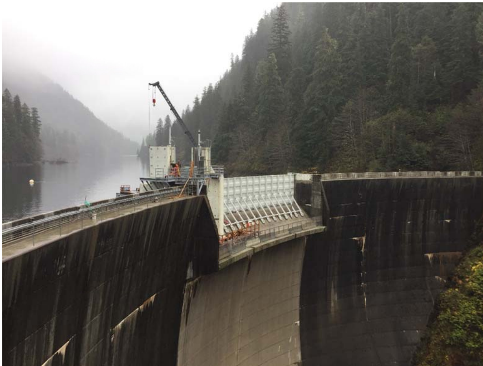
Installation Complete for all Spillway Structural Components
