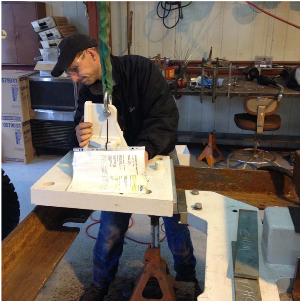
Swan crew member Rob Miller with fabricated jig for “kicker” column assembly
