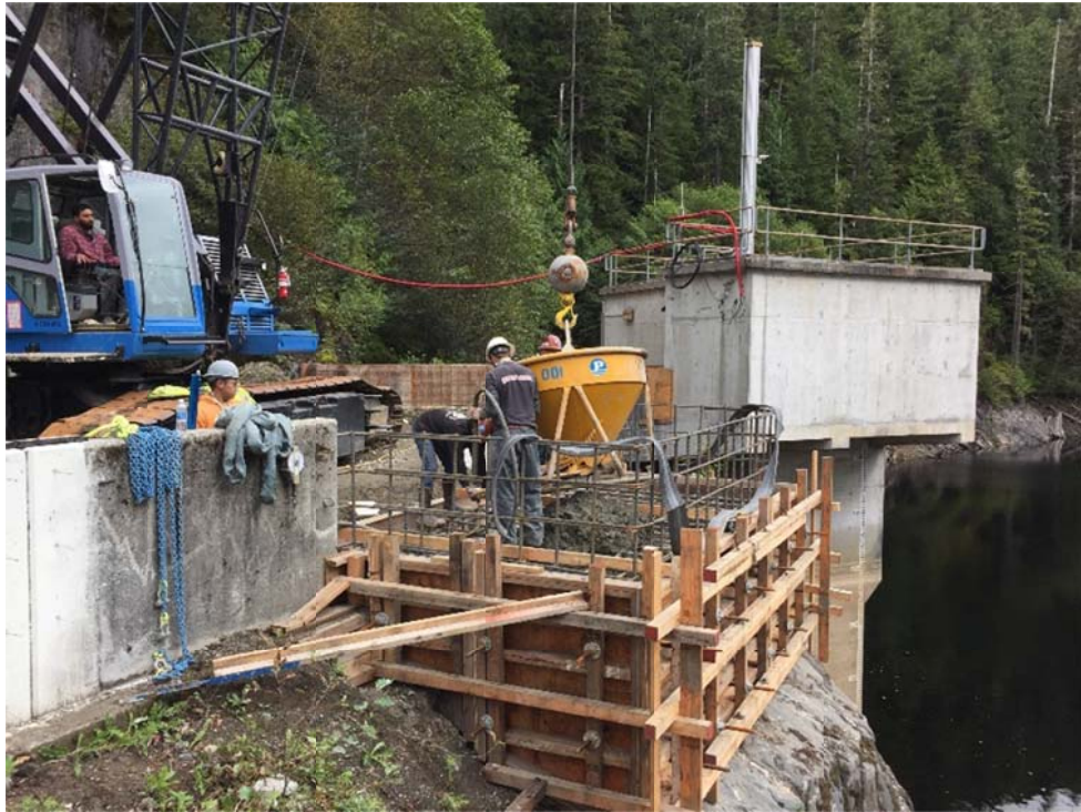
New Lake Debris Slab & Parapet Wall Installation
