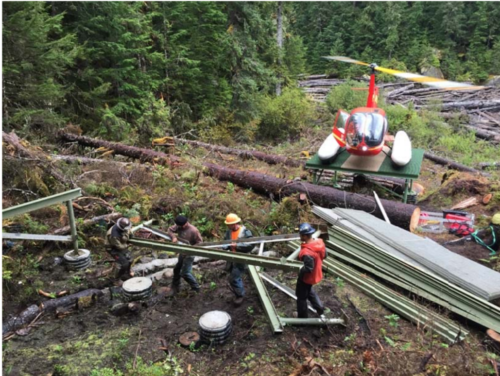
Reassembly of Emergency Shelter Foundation
