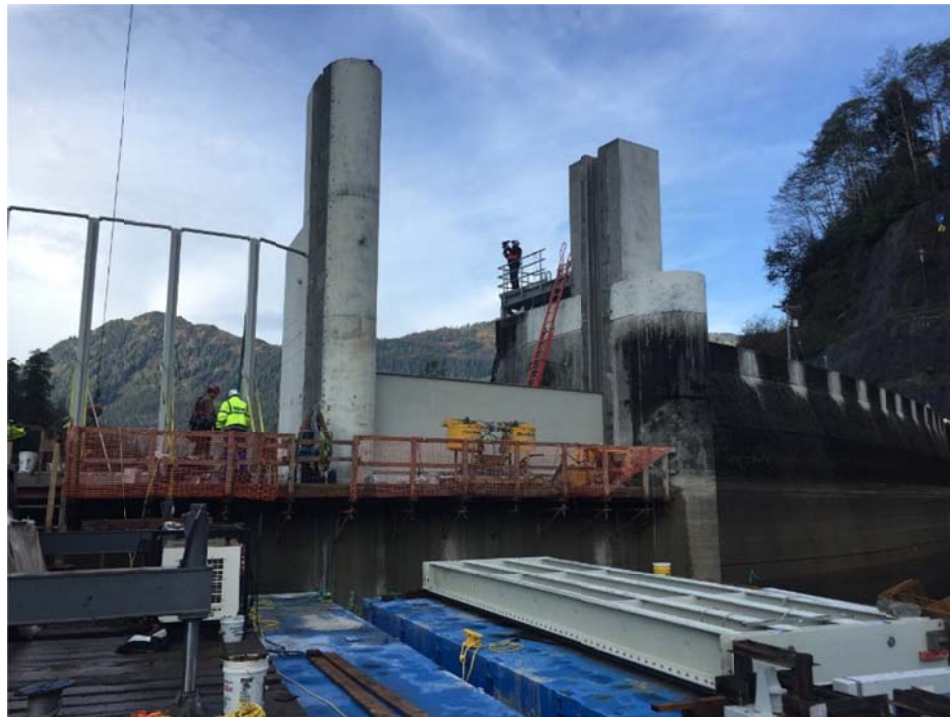
First Section of Fixed Wheel Gate Installed
