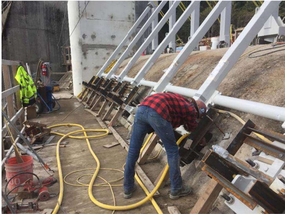
First Stage Grounding of Column Kicker Anchors
