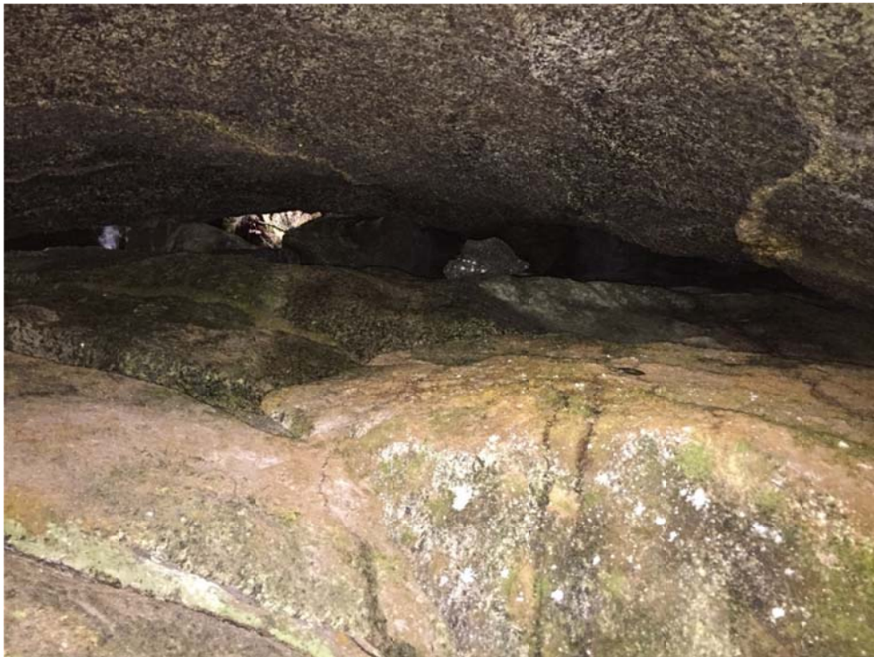
Typical Abutment Rock Voids Filled with Two-Part Expandable Foam During Phase 2 - Elevation 1395 Feet
