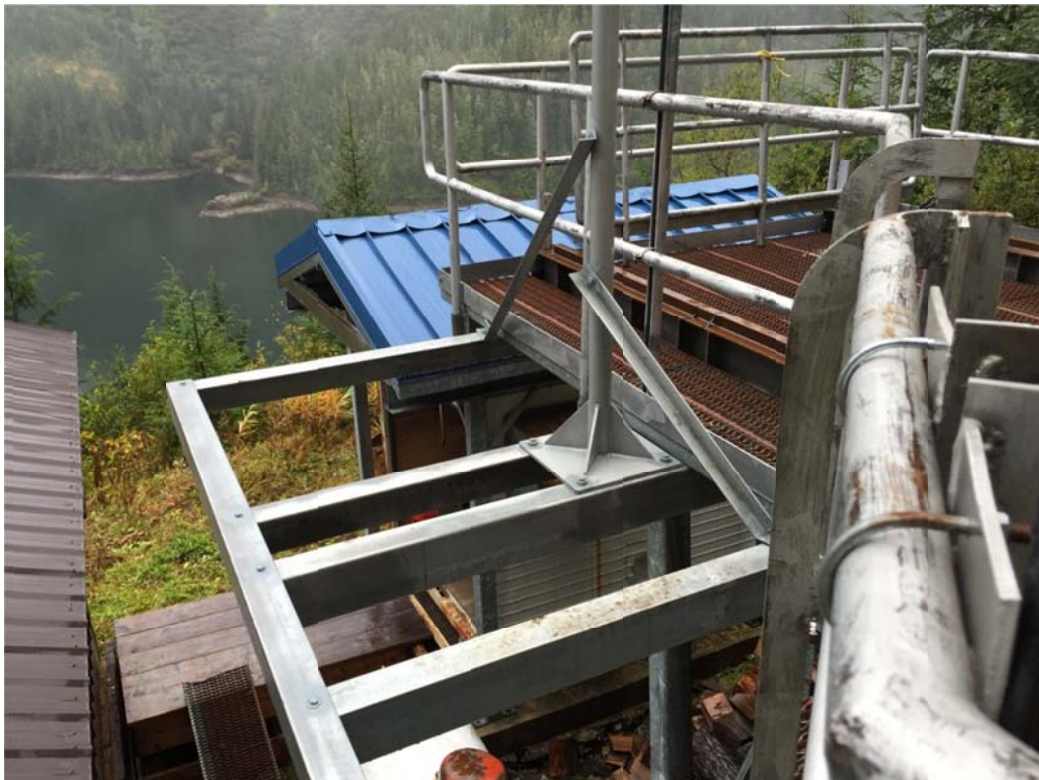
Satellite Bracket Complete & Ready for Dish Installation
