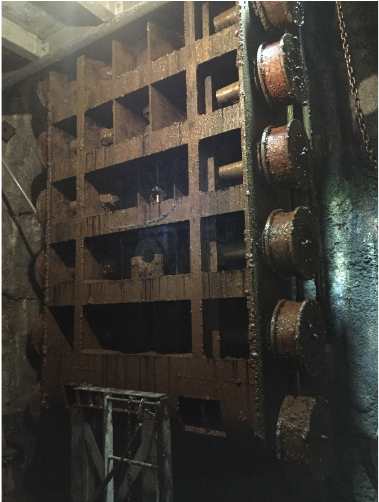
Tyee Intake Gate during 2018 Inspection
