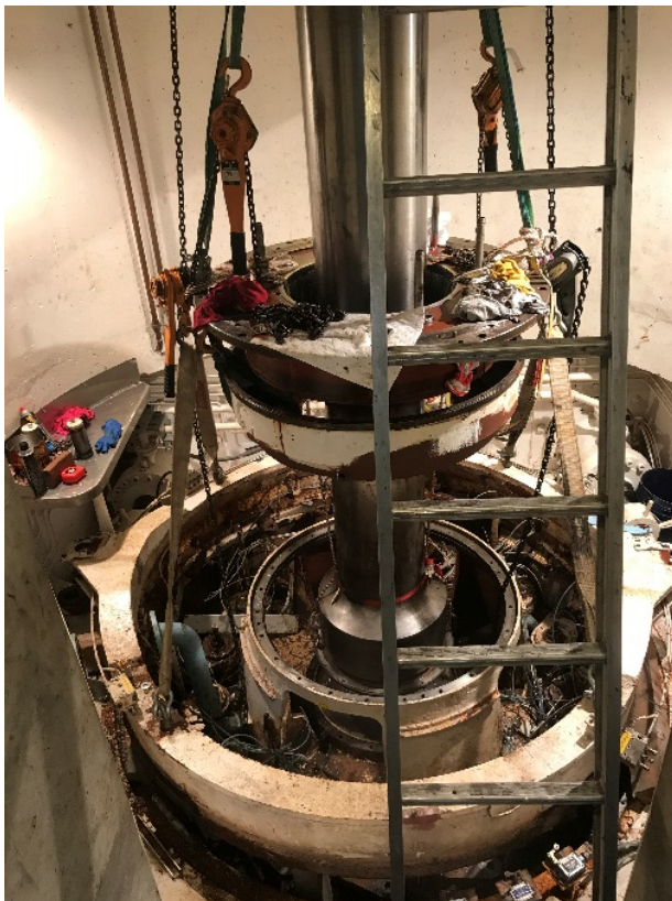
Unit 1 - Disassembly of Turbine End Guide Bearing Wicket Gate Control Ring and Stuffing Box Seal in 2019
