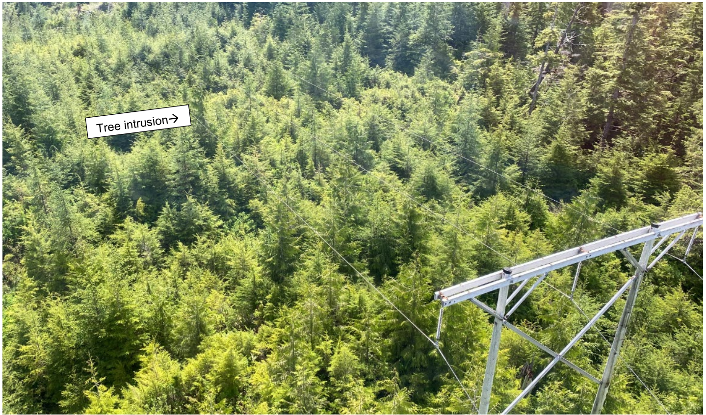
Tree Intrusion on Swan/Bailey Transmission Line Structure #250
