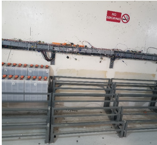
Removal of Existing Bank and Seismic Rack
