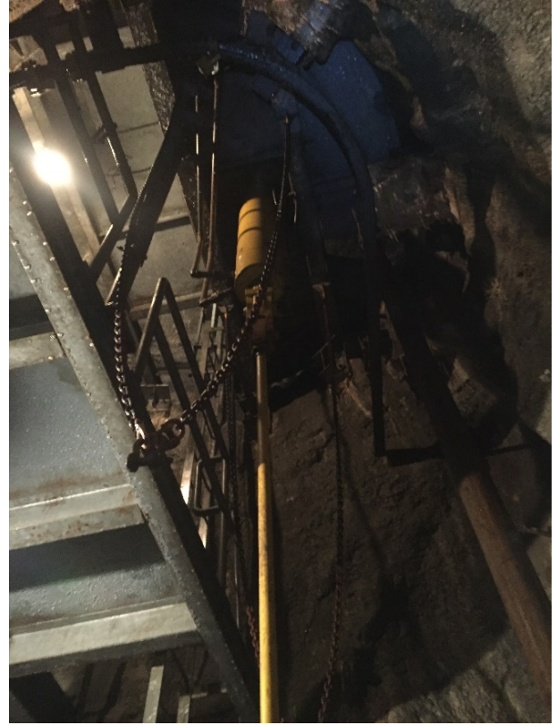
Gate Cylinder and Stem
