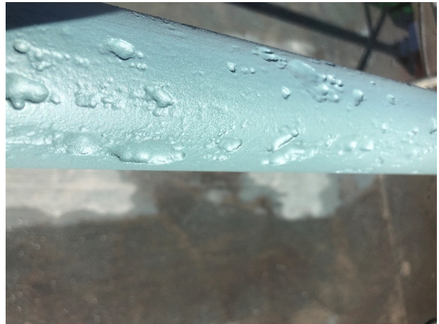
Gate Stem Corrosion
