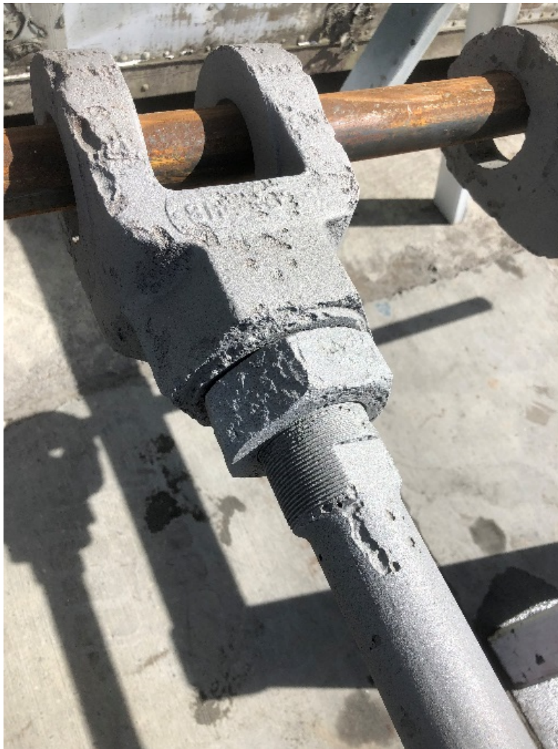
Gate Stem Clevis End Corrosion
