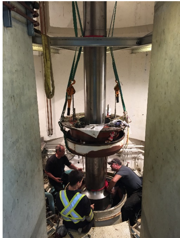
Unit 1 - Disassembly of Turbine End Guide Bearing Wicket Gate Control Ring and Stuffing Box Seal in 2019
