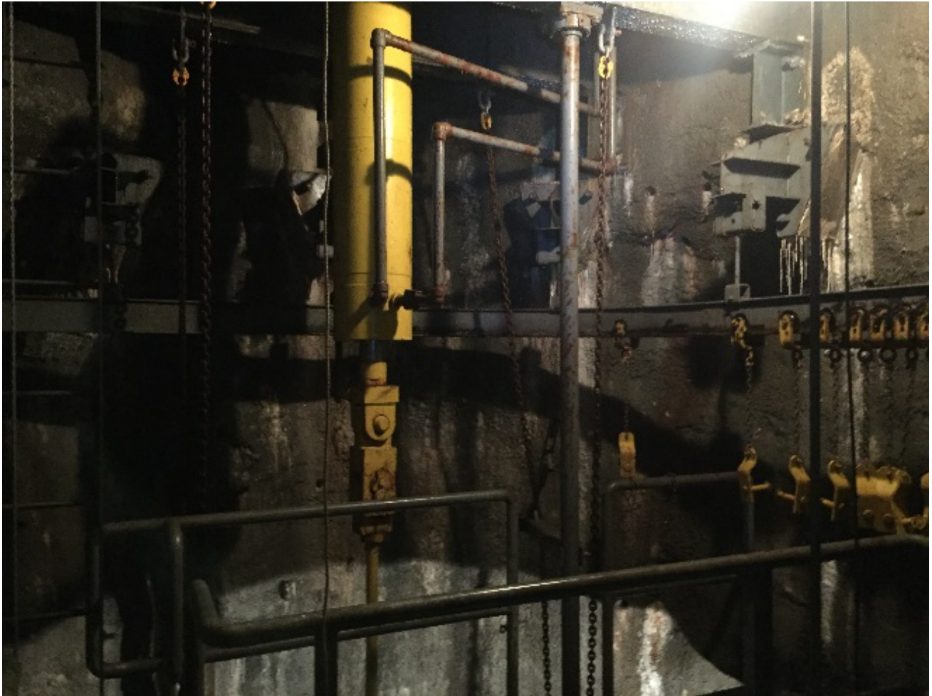
Gate Hydraulic Cylinder
