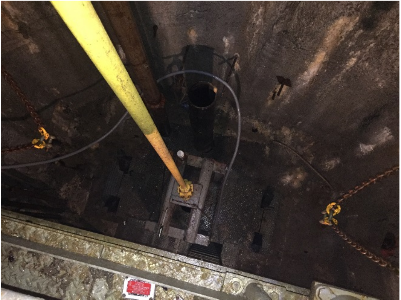
One of 18 Gate Stems connecting the Intake Gate to the Cylinder
