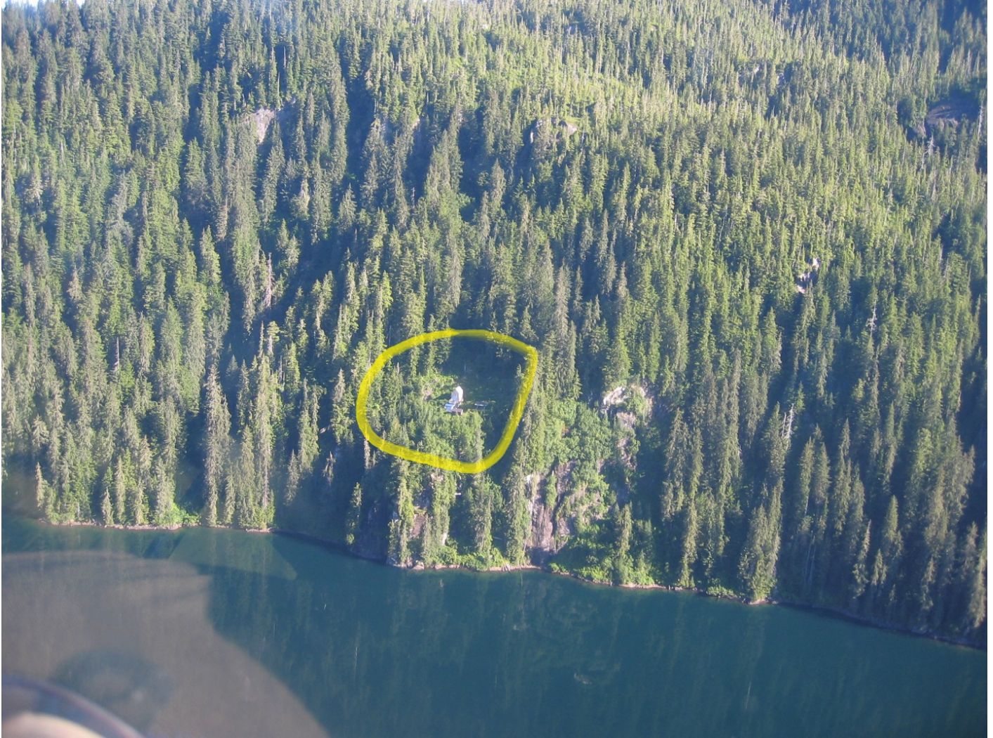
Tyee Lake Gatehouse Located at Elevation 1630.0' / Tyee Lake Elevation 1396.0'
