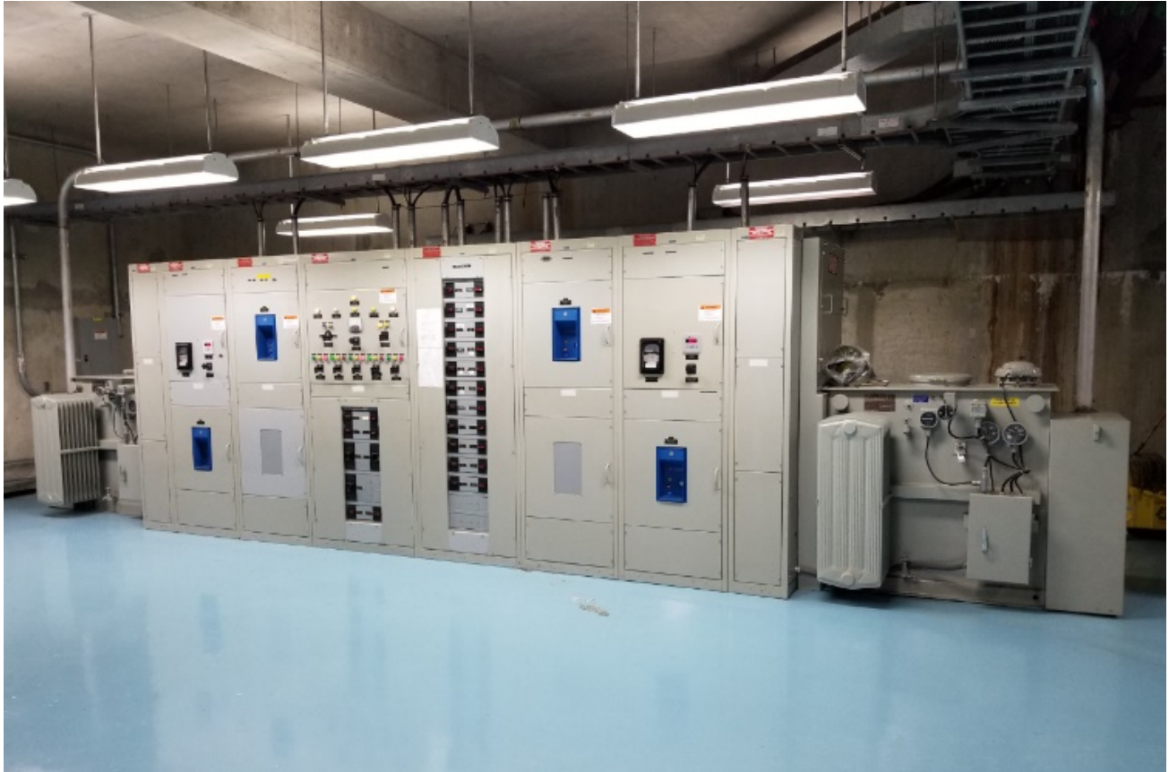
Swan Lake Existing Switchgear
