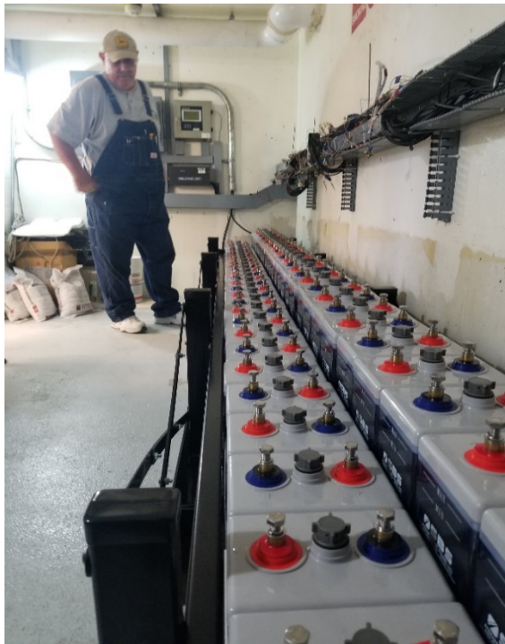
New Battery Bank and Seismic Rack Install
