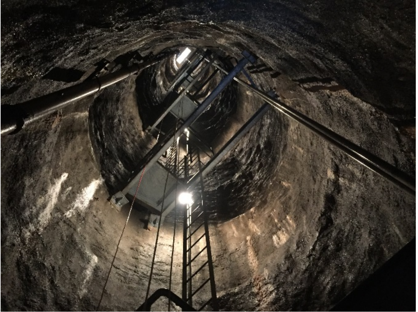
Gate Shaft & Man Ladder System
