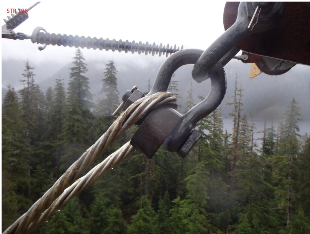
Improper spool for preform to rest in – will eventually cause failure.
