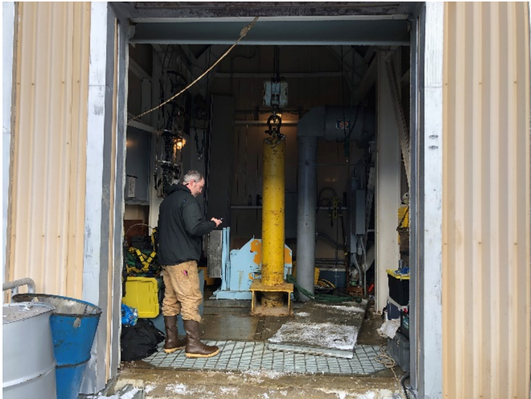
Cylinder started down Gate Shaft
