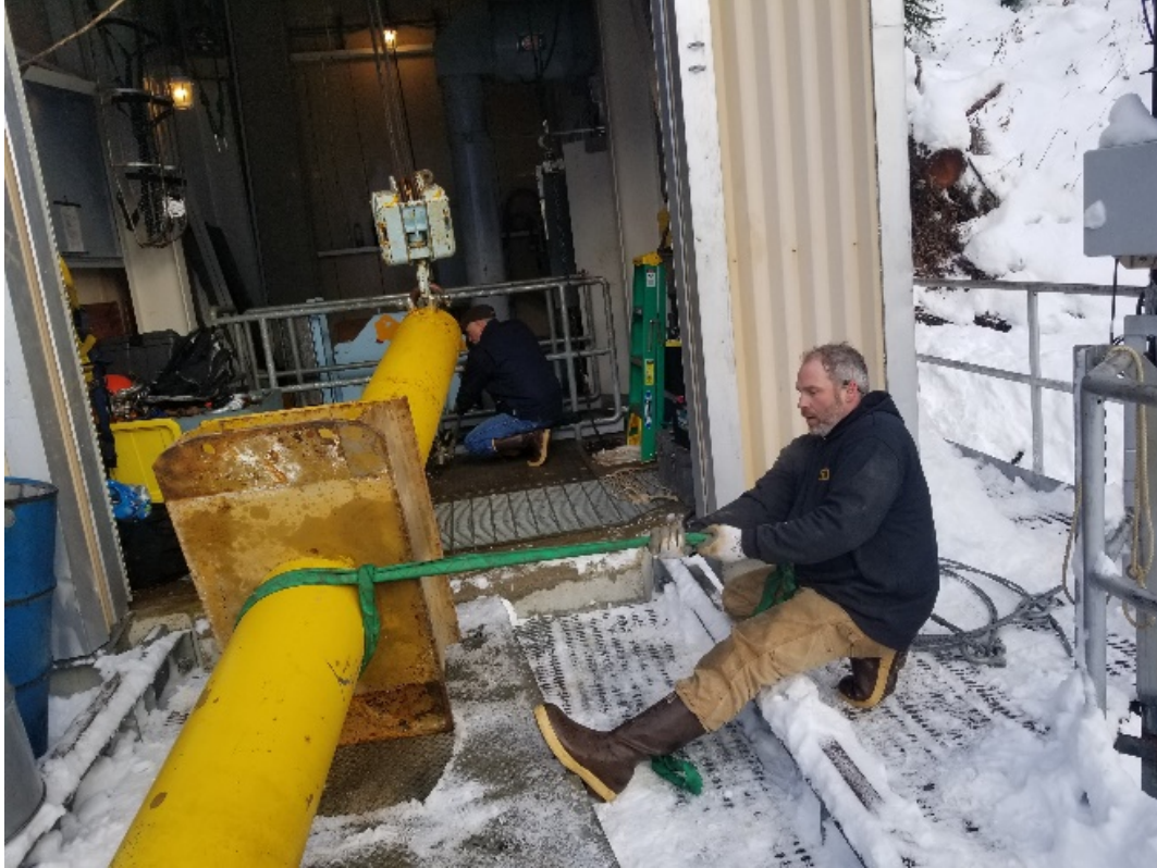
Moving Cylinder from Staging Deck into Gatehouse
