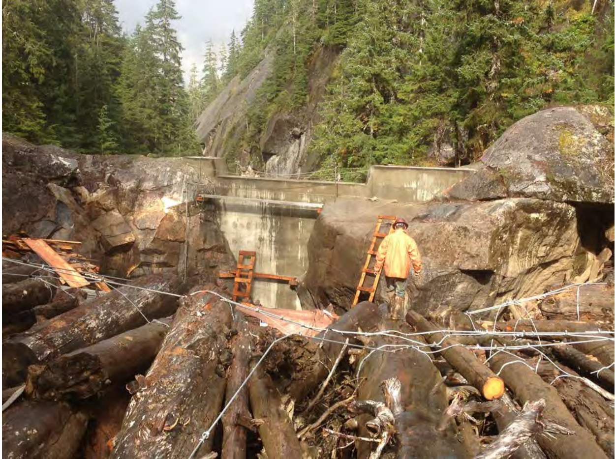
Looking at Weir from upstream approach; permanent log retention cables in foreground.
