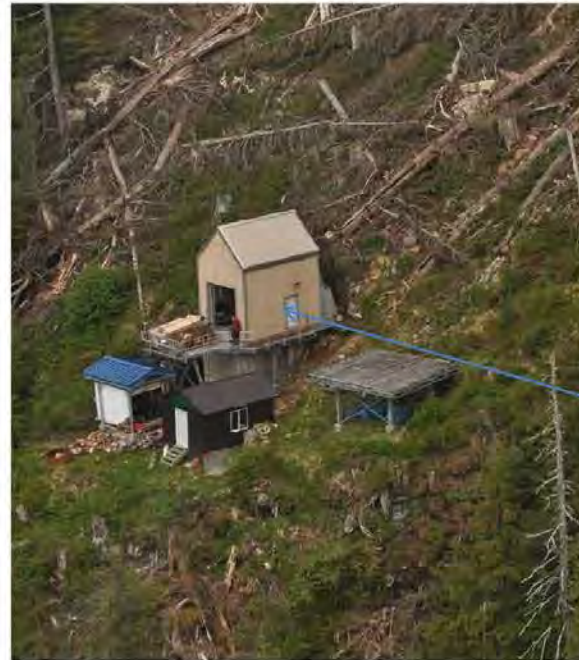
Gate House with helicopter pad, generator Building and crew shack that Steve built
