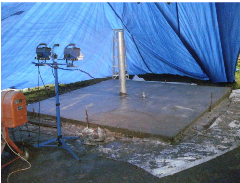
Satellite dish pad and stand installed
