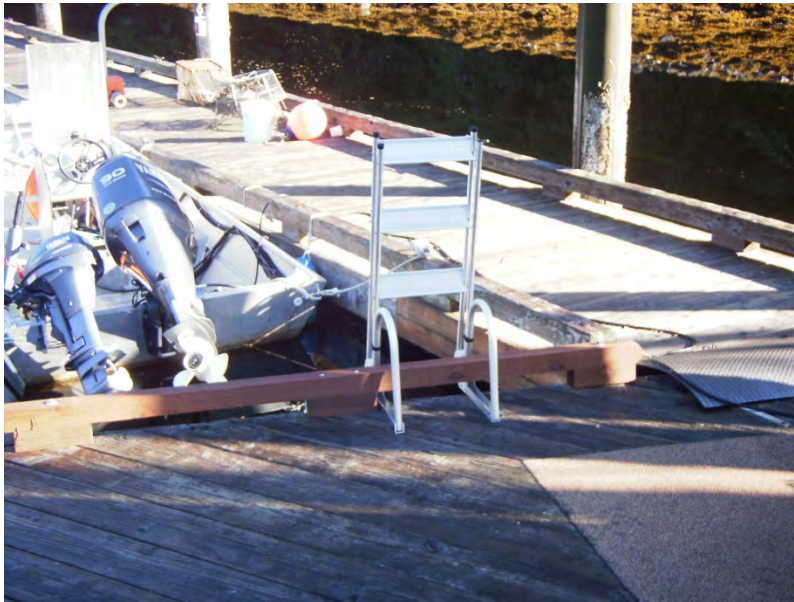
Dock ladder and toe kicks installed
