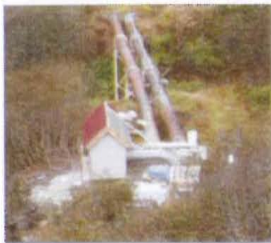
Low Level Outlet Works
