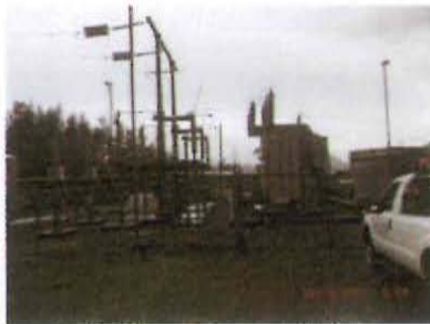
Wrangell Distribution Substation
