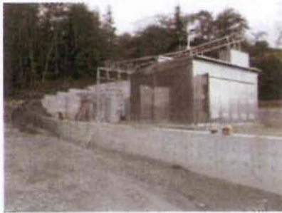
Bethe Under Construction
