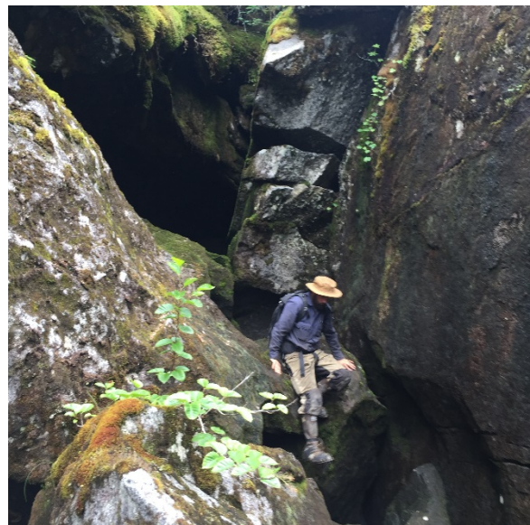
Downstream Voids of Tyee Weir
