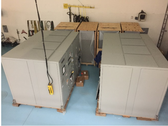
Replacement Exciters & Switchgear
