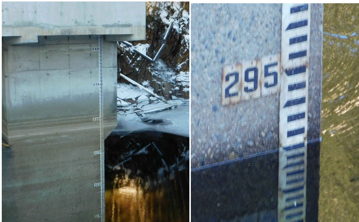
Above: Reading Lake Level Staff Gauge
