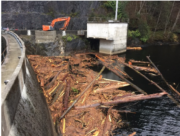
North Dam Abutment & Debris Removal Work Platform / Reservoir Access site
