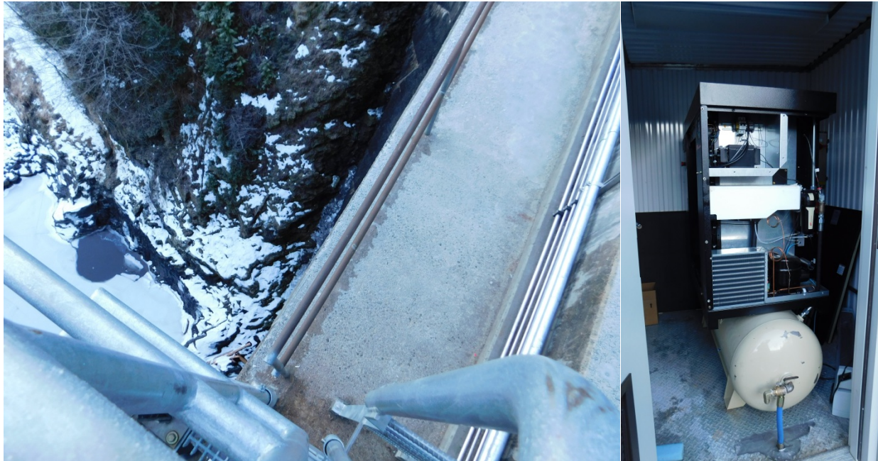
Above: Access to compressor room
