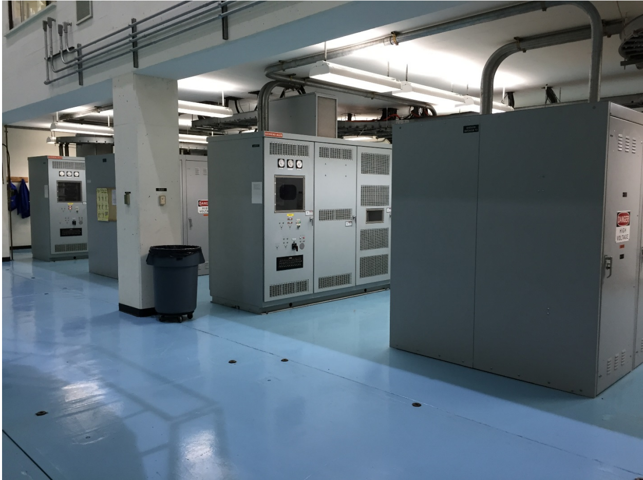
Swan Lake existing Exciter & Switchgear cabinets to be removed and replaced
