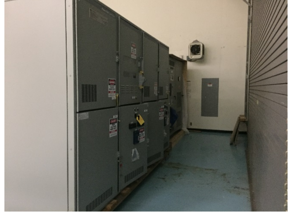
Switchgear Cabinets - access doors
