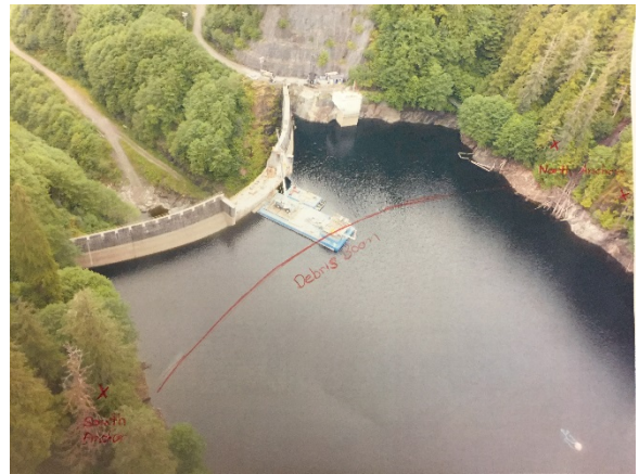
Debris Boom & Shore Anchor locations
