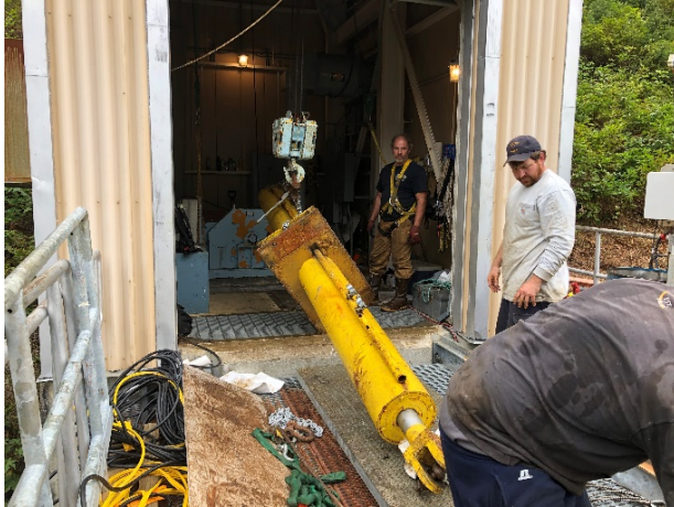
Tyee Gate Intake Cylinder Removal
