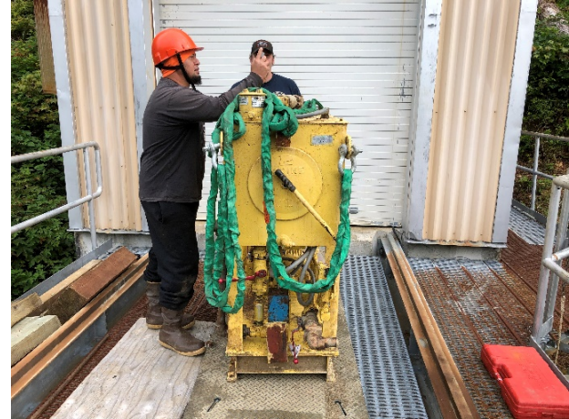
Tyee Intake Gate HPU Removal
