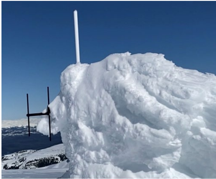
Burnett Peak Repeater Shack before Snow Removal
