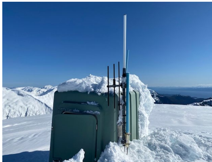
Burnett Peak Repeater Shack after Snow Removal
