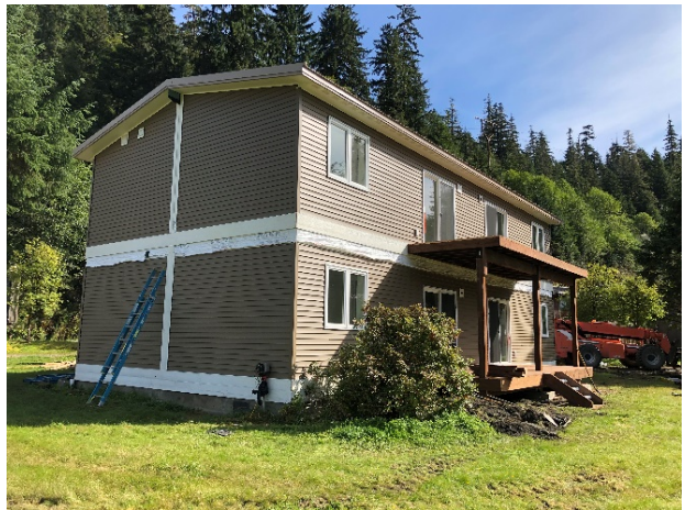
Four-Plex Front Decks Installed
