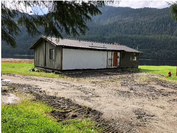
Disassembly of Existing Home #102 Removal
