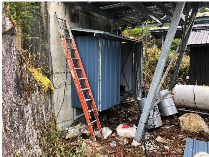
HPU Enclosure 90% Complete
