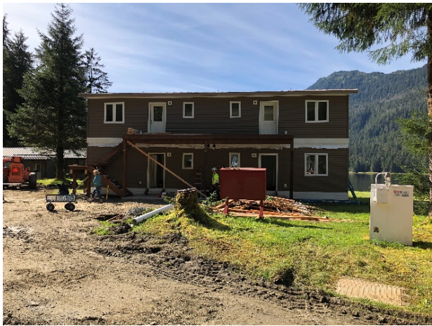
Four-Plex Assembled and Back Decks Started
