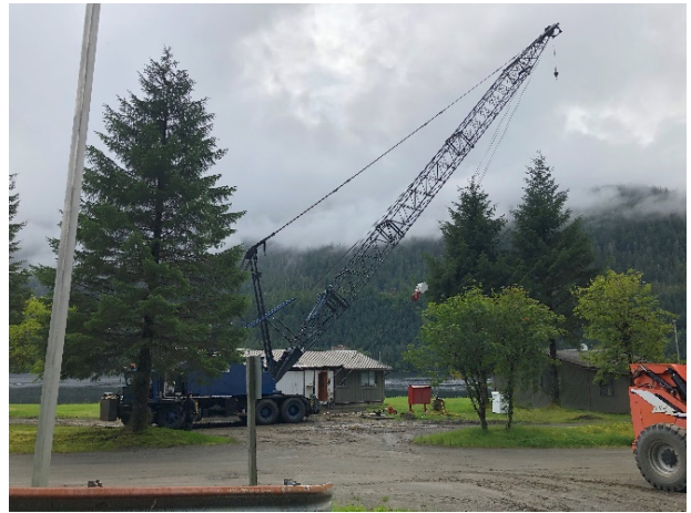
Setting Crane for Home #102
