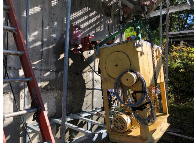
Installation of HPU on New Mounting Platform and Core Holes Being Drilled for Hydraulic Line Access
