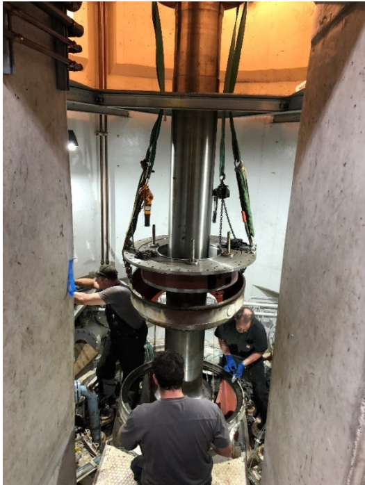
Lower Guide Bearing Disassembled
