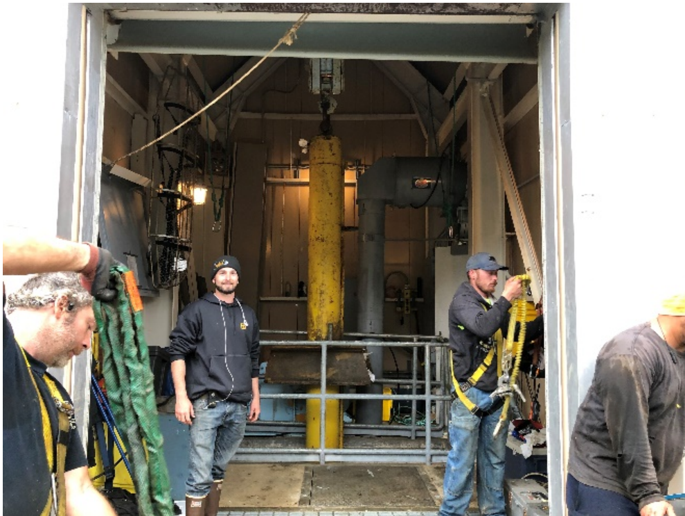
Intake Gate Cylinder Hanging from Hoist Control
