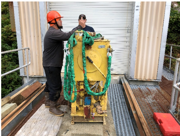
HPU Removed from Gate Shaft staged for Helicopter Removal
