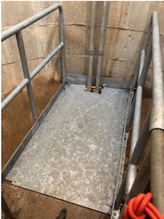
New Limit Switch Work on Deck Installed in Gate Shaft at El. 1610.0'
