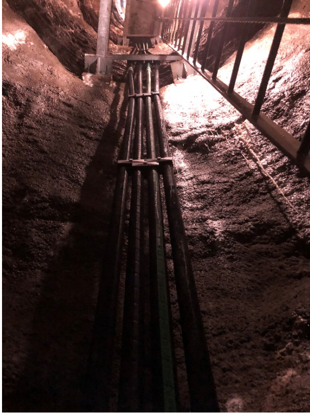
Hydraulic Oil Supply & Return Cylinder Lines Installed in Gate Shaft
