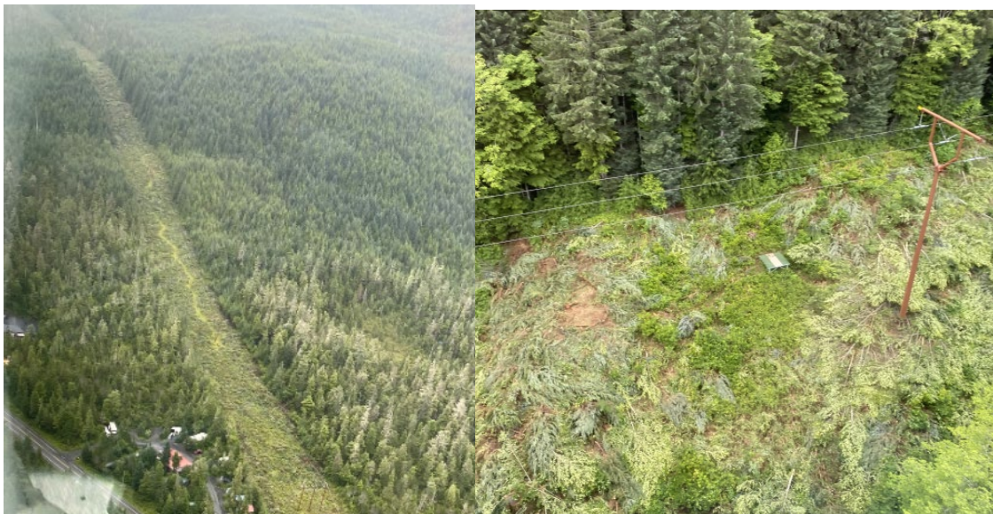
Figure #4 - Sections of completed Mitkof Island and Neets Bay brushing work
