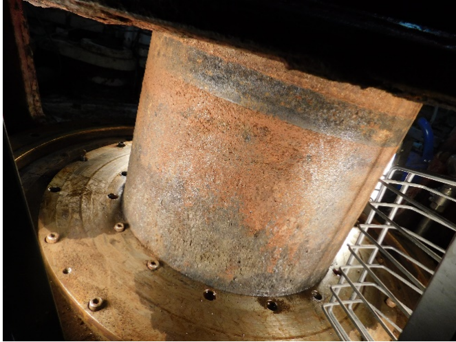
Turbine Shaft Cleaned for Epoxy Application
