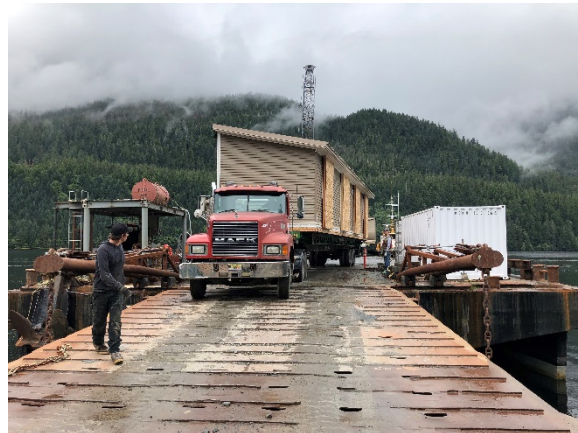
Off Loading Modular Home Units
