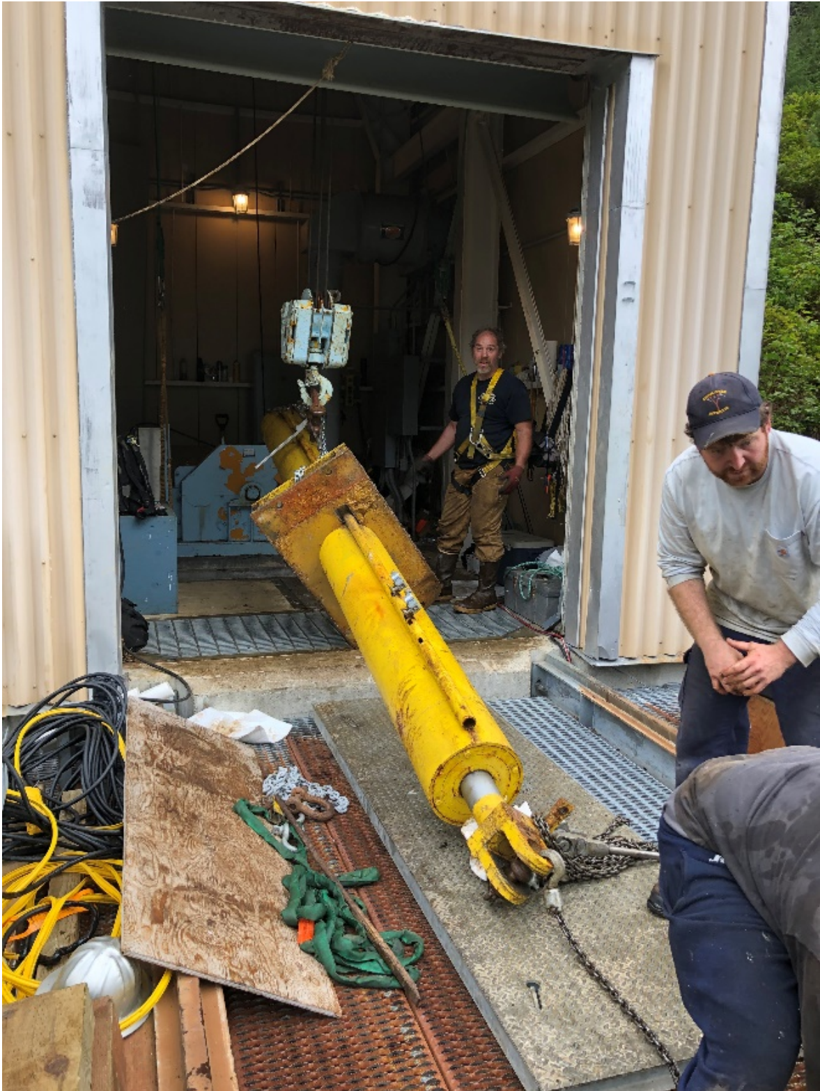
Intake Gate Cylinder Removal from Gatehouse
