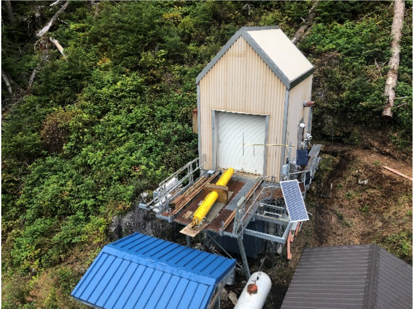
Intake Cylinder staged on Gate House Deck for Helicopter Removal
