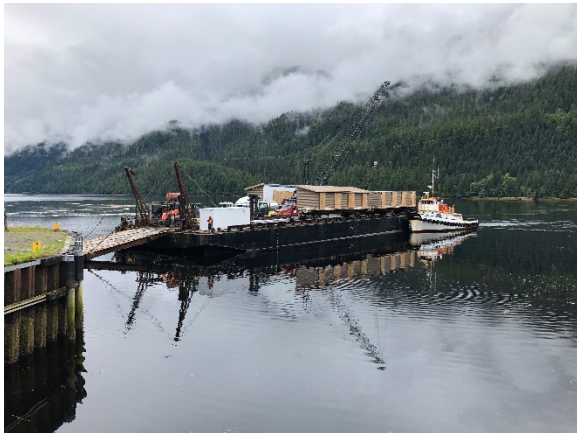
Barge Arriving at Swan Lake Bulkhead
