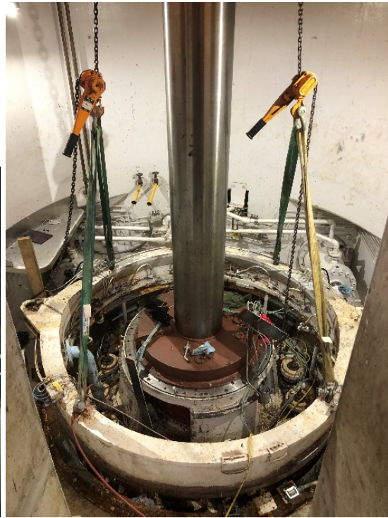
Stuffing Box Installed / Distributor Ring Removal for Bushing Replacement
