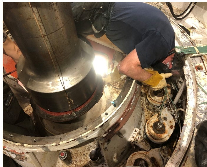
Cleaning Surface of Turbine Shaft
