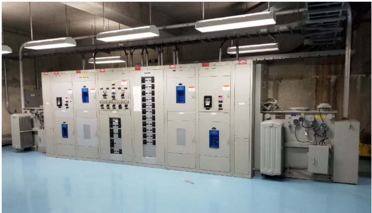
Swan Lake Existing Switchgear
