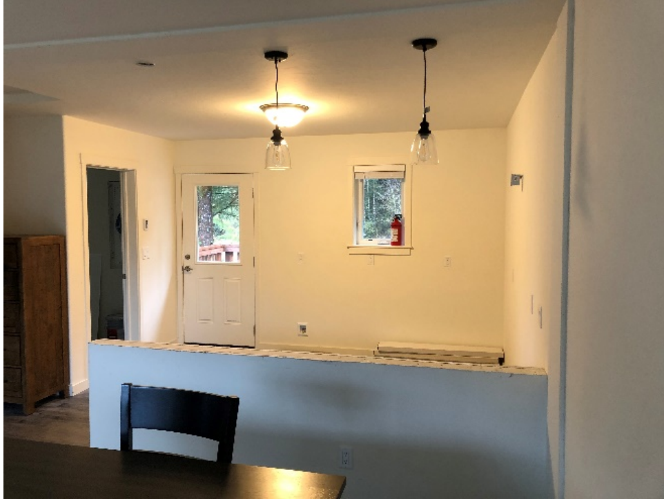
Unit 104 Unfinished Kitchen
