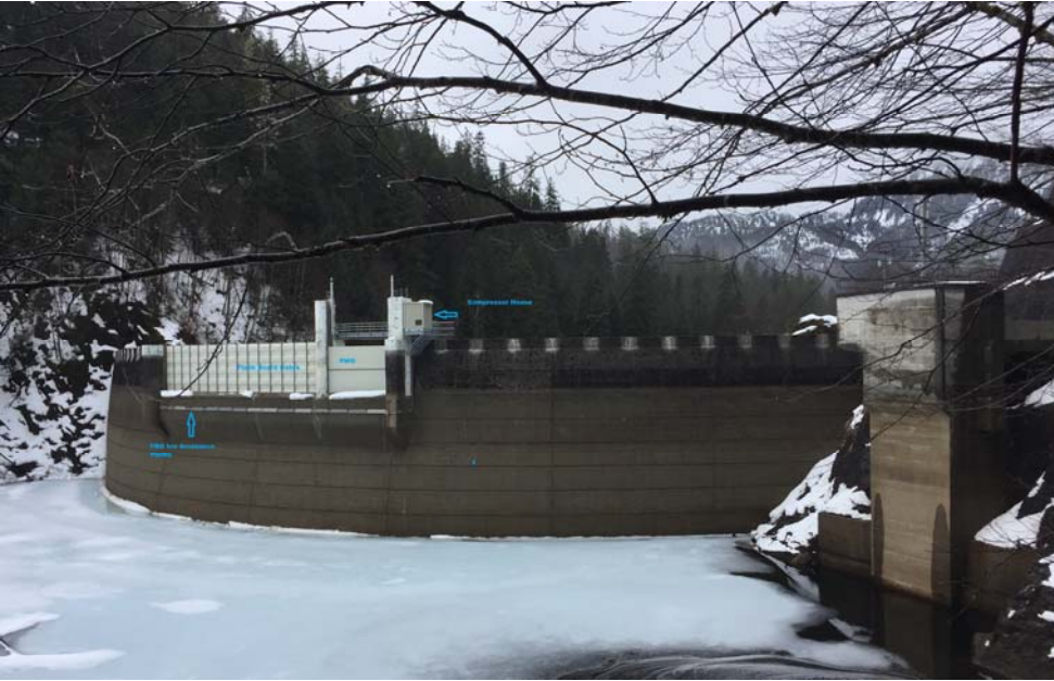
Swan Lake Reservoir Dam Spillway Control Gates Elevation 284.0'
