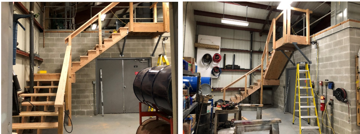
Shop Mezzanine Stairs Replaces Originally Installed Man Ladder
