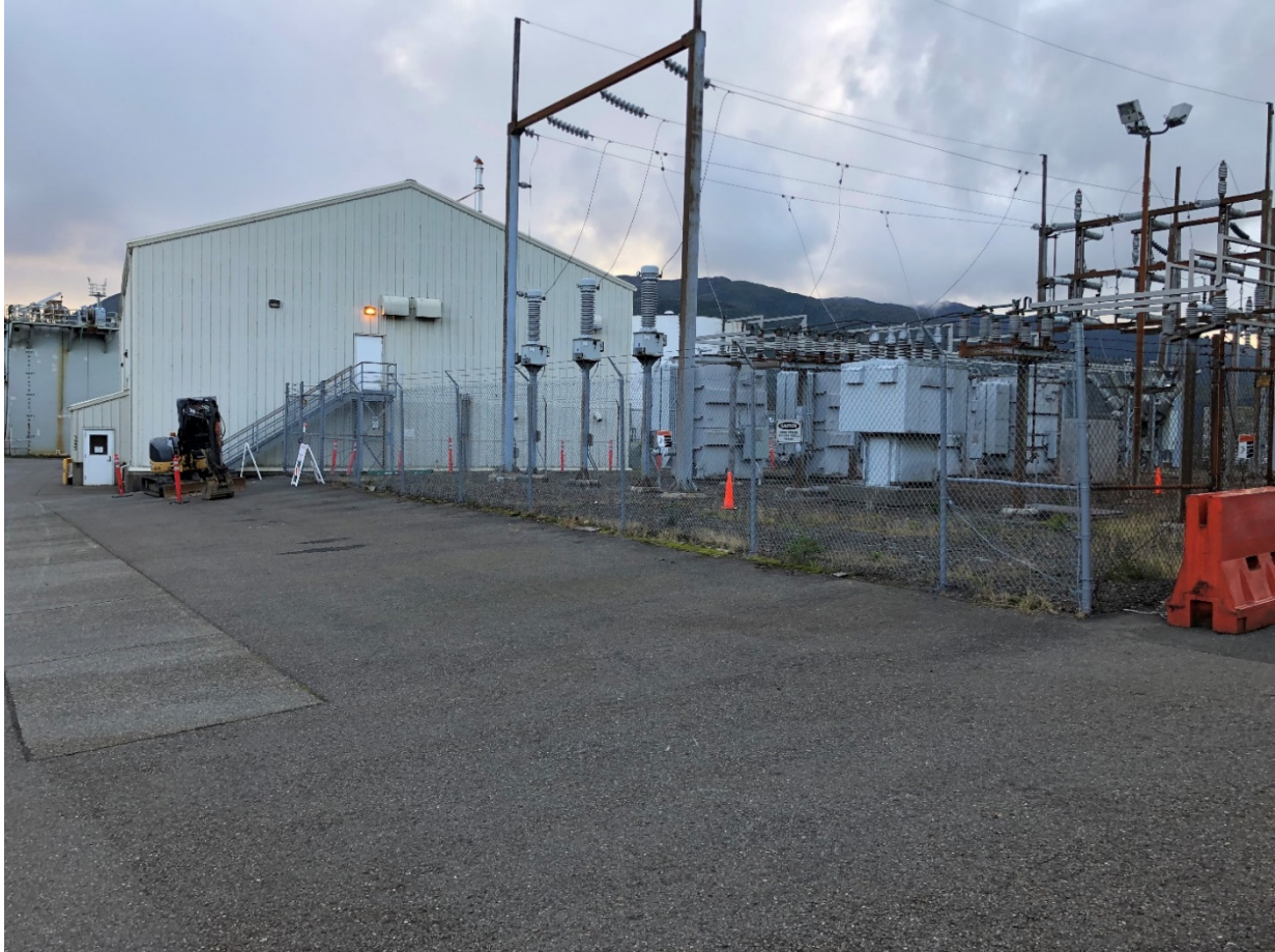
Bailey Substation after Renovations to Security Fencing
