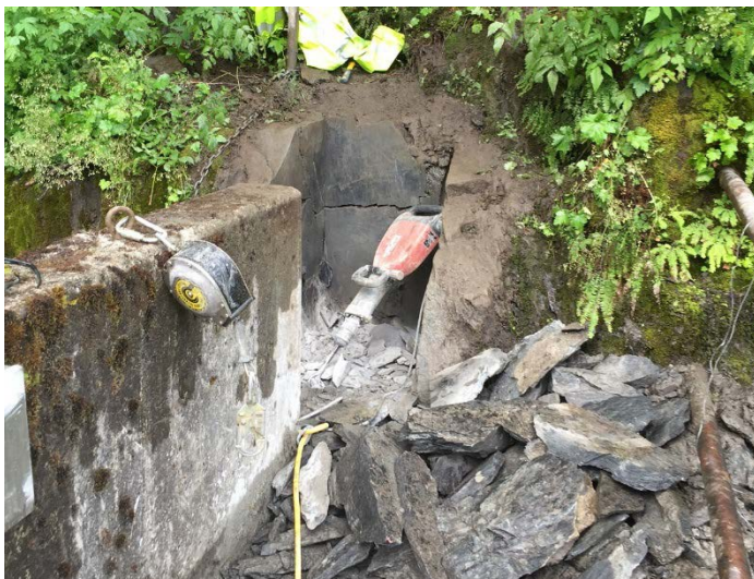
Left Dam Abutment – Parapet Wall Key
