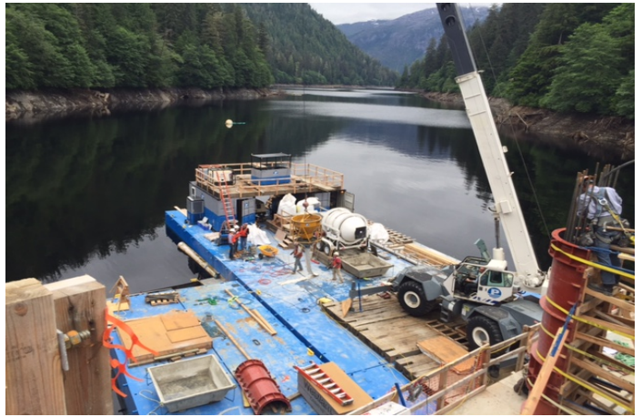
Concrete Batch Plant on Flexi-Float Barge
