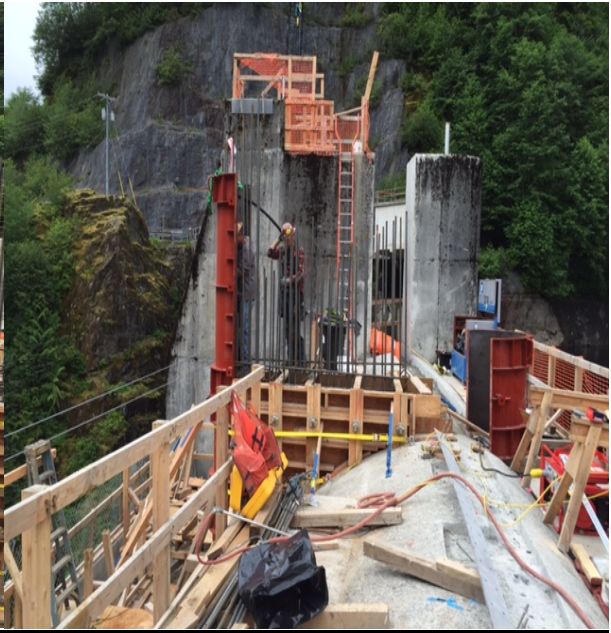
Middle Pier Base Concrete Placement
