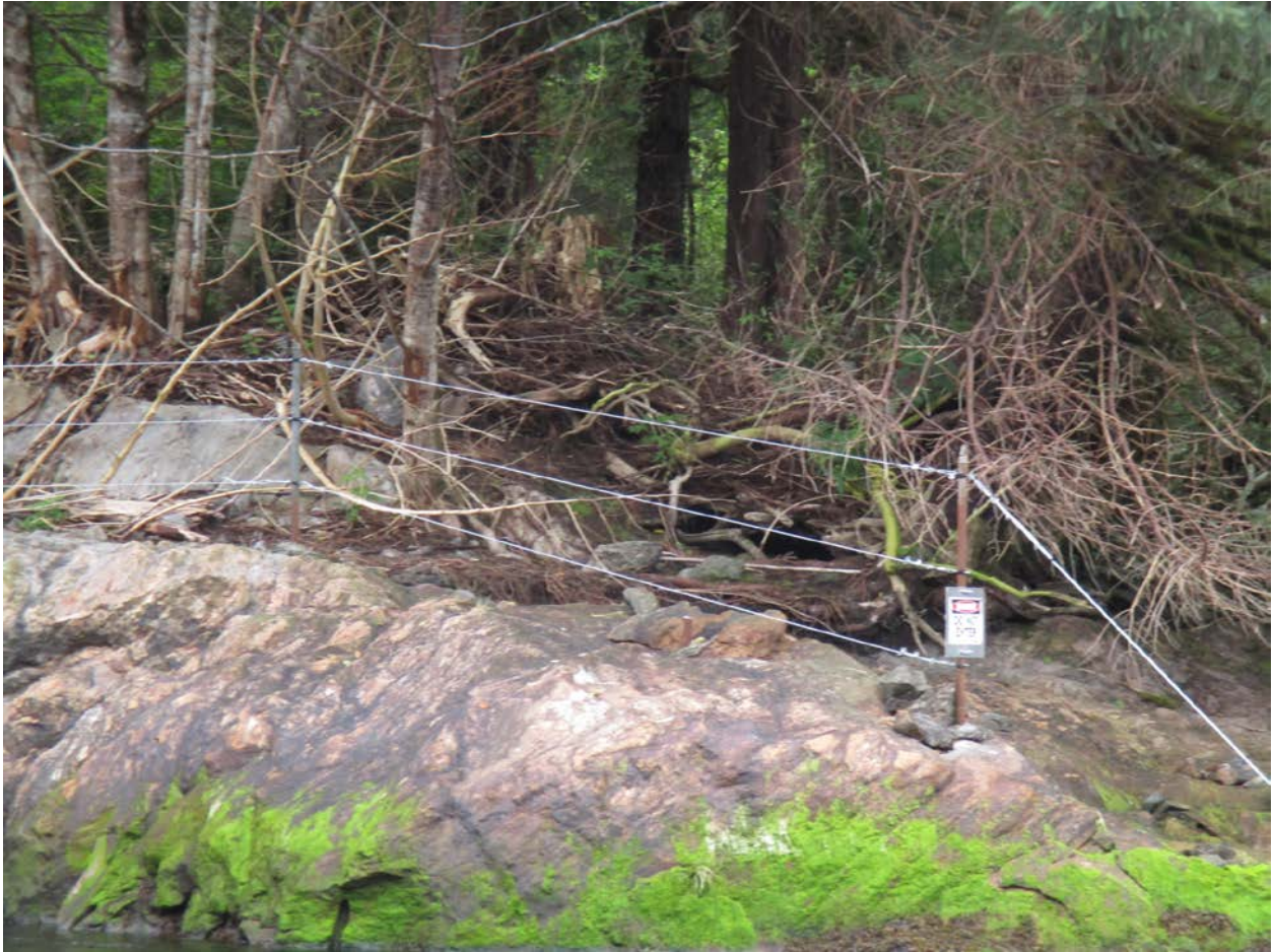
Tail race barrier fencing
