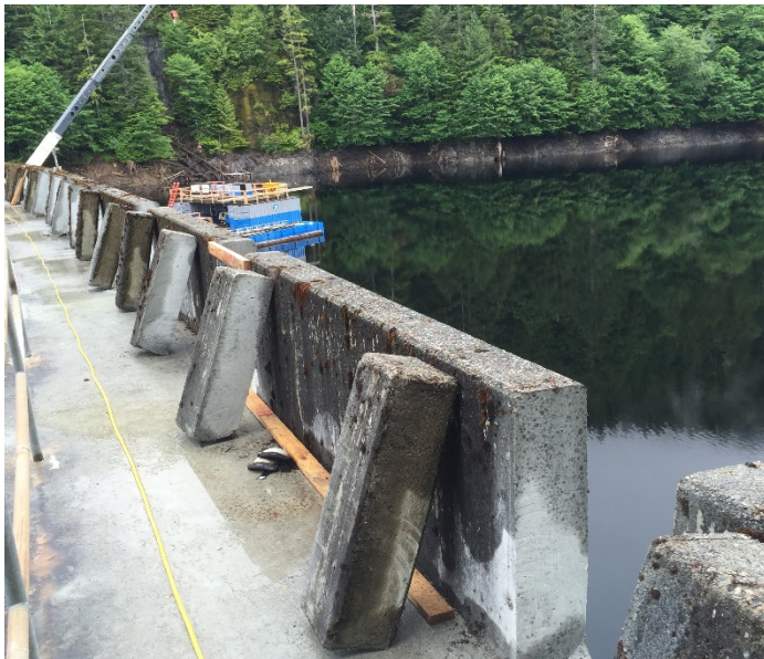
Parapet Wall Concrete Excavation
