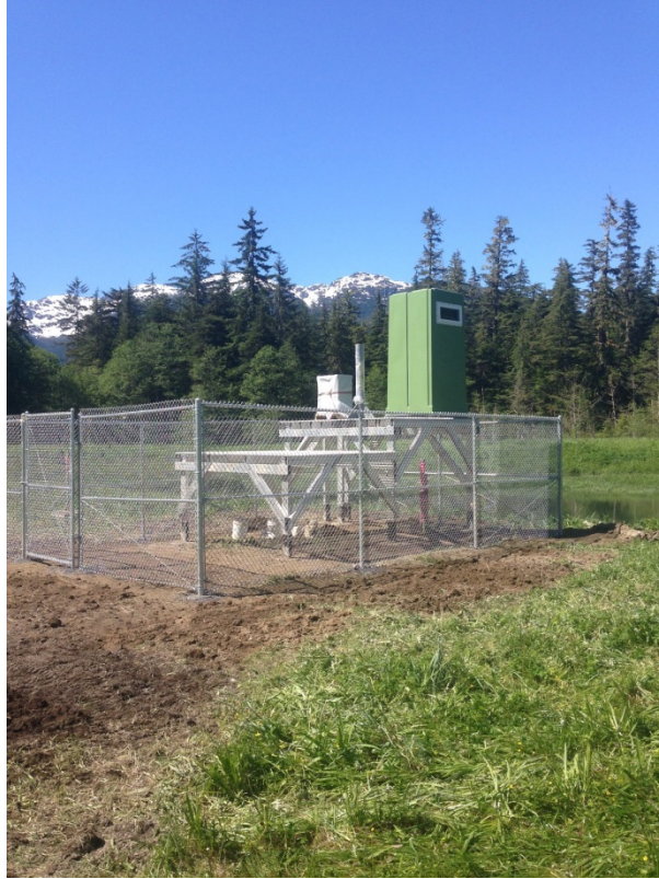
Tyee Satellite Platform installed by Alaska Clearing
