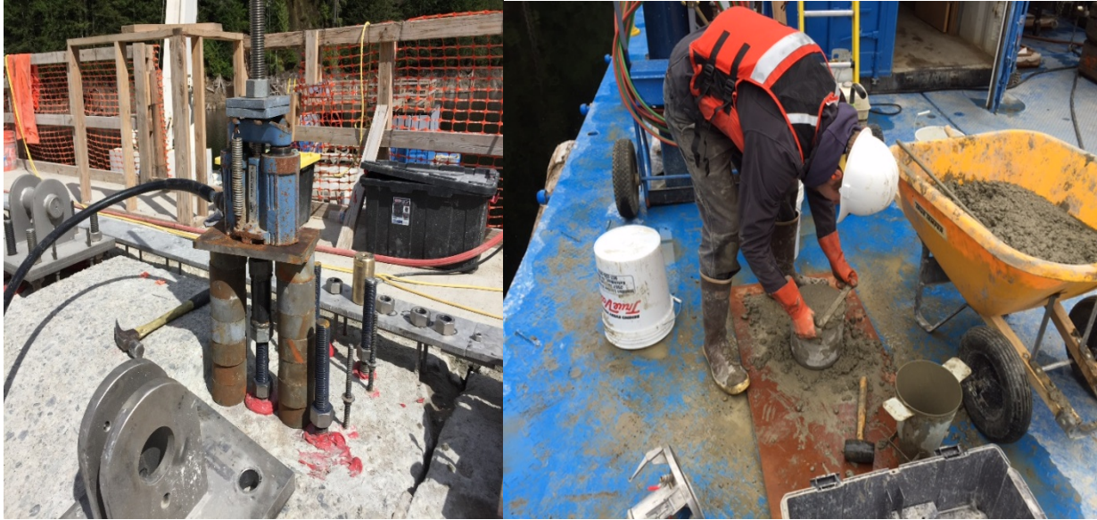
Epoxy Resin Anchor Pull Testing 42,000 lbs.
