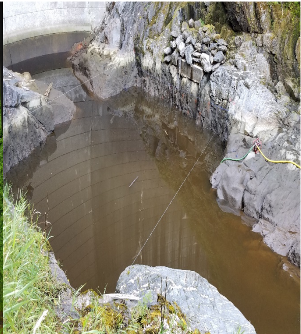
Dewatering the Plunge Pool
