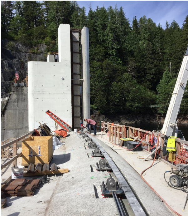
Column Chairs / Gate Guides Installed
