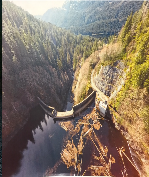
Debris in Lake (Spring 2016)
