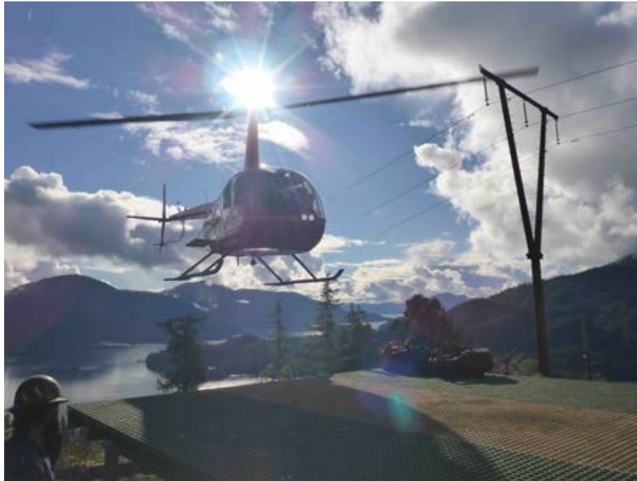
New Helipad at Tower 97 on the Intertie
