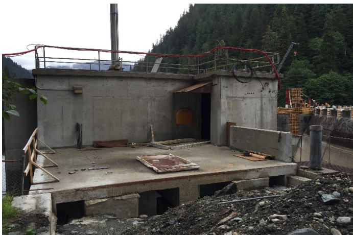
Intake Structure Excavation
