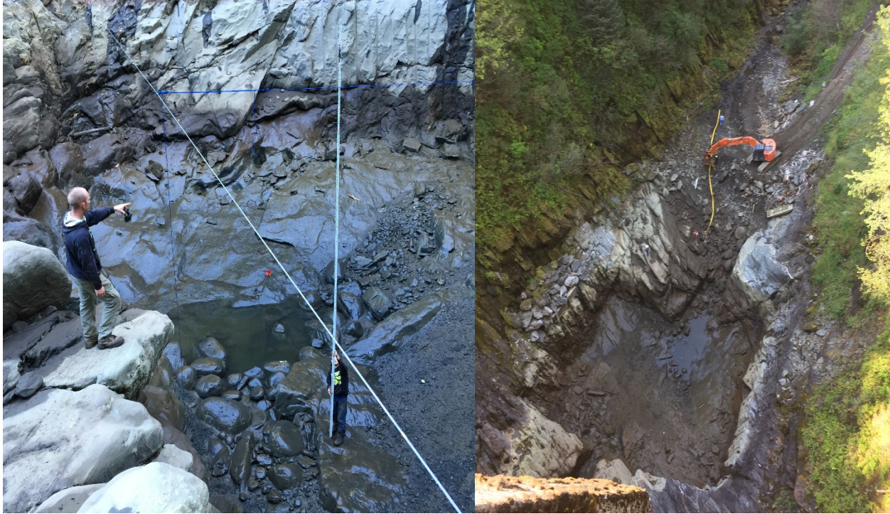
Survey of Plunge Pool Bottom
