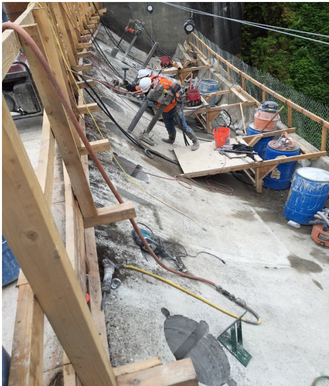
Spillway Demolition / Kicker Anchor
