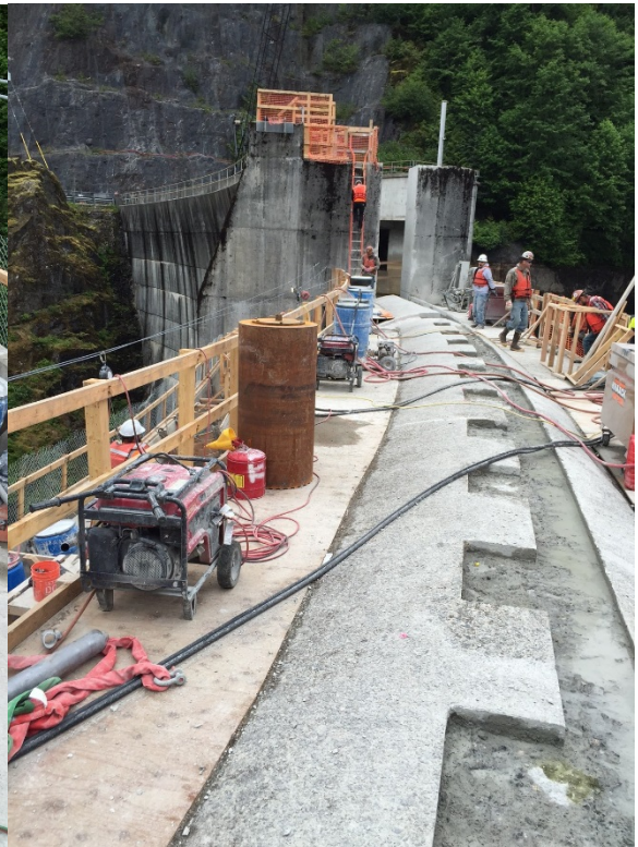
North Pier Demolition / Flash Board Sill
