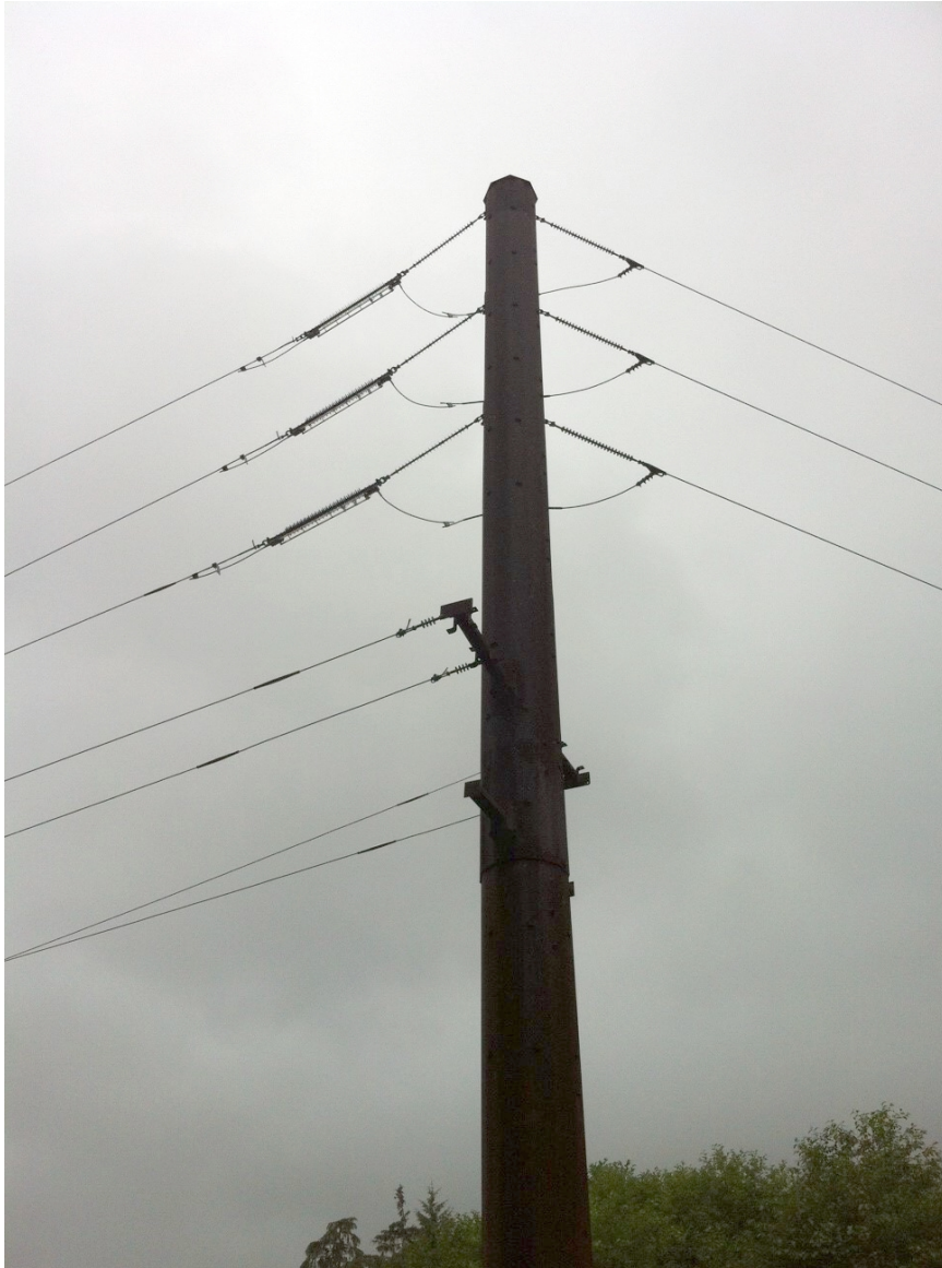
115 kV in-line switches at tower 138
