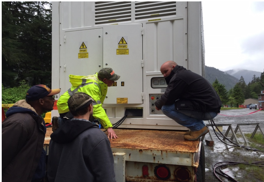
Commissioning and Operator Training of Load Bank
