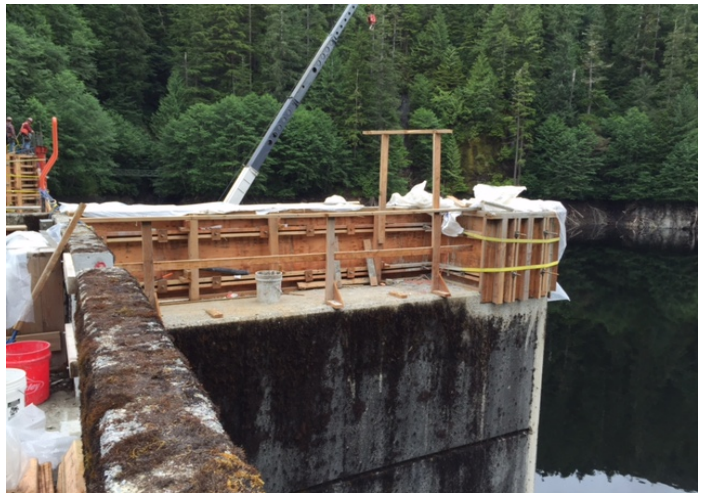
South Pier Height Increase
