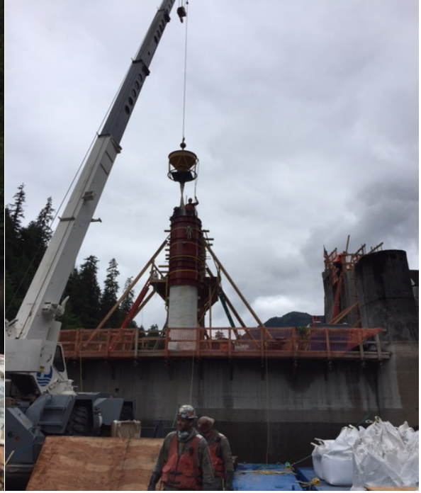
Concrete Placement Middle Pier
