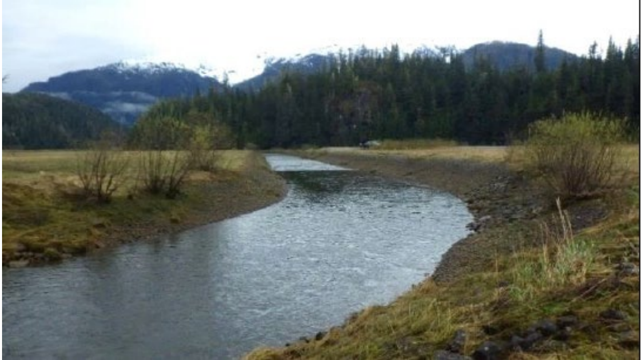
Photo 4-10 Tyee Lake Project Tailrace at -1.5 ft tide, Looking Downstream from the Powerhouse. Source: ADF&G 2018.
