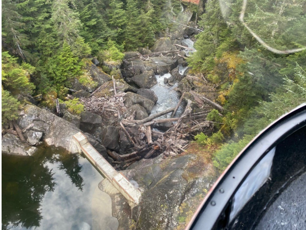
Photo 4-1 Tyee Creek at Tyee Lake Outlet Weir Looking Downstream when no Water is Flowing from Tyee Lake over the Weir.
