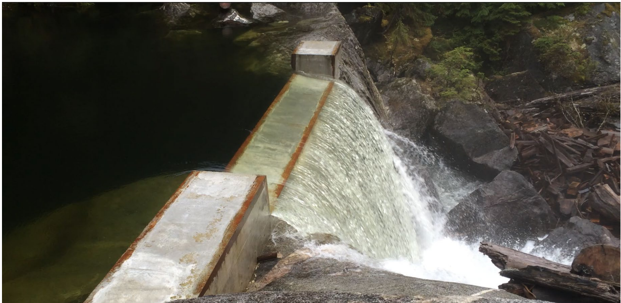
Photo 2-1 Tyee Lake Spillway Weir.
