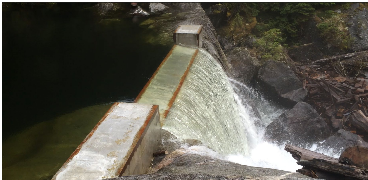
Photo 2-2 Tyee Lake Spillway Weir.
