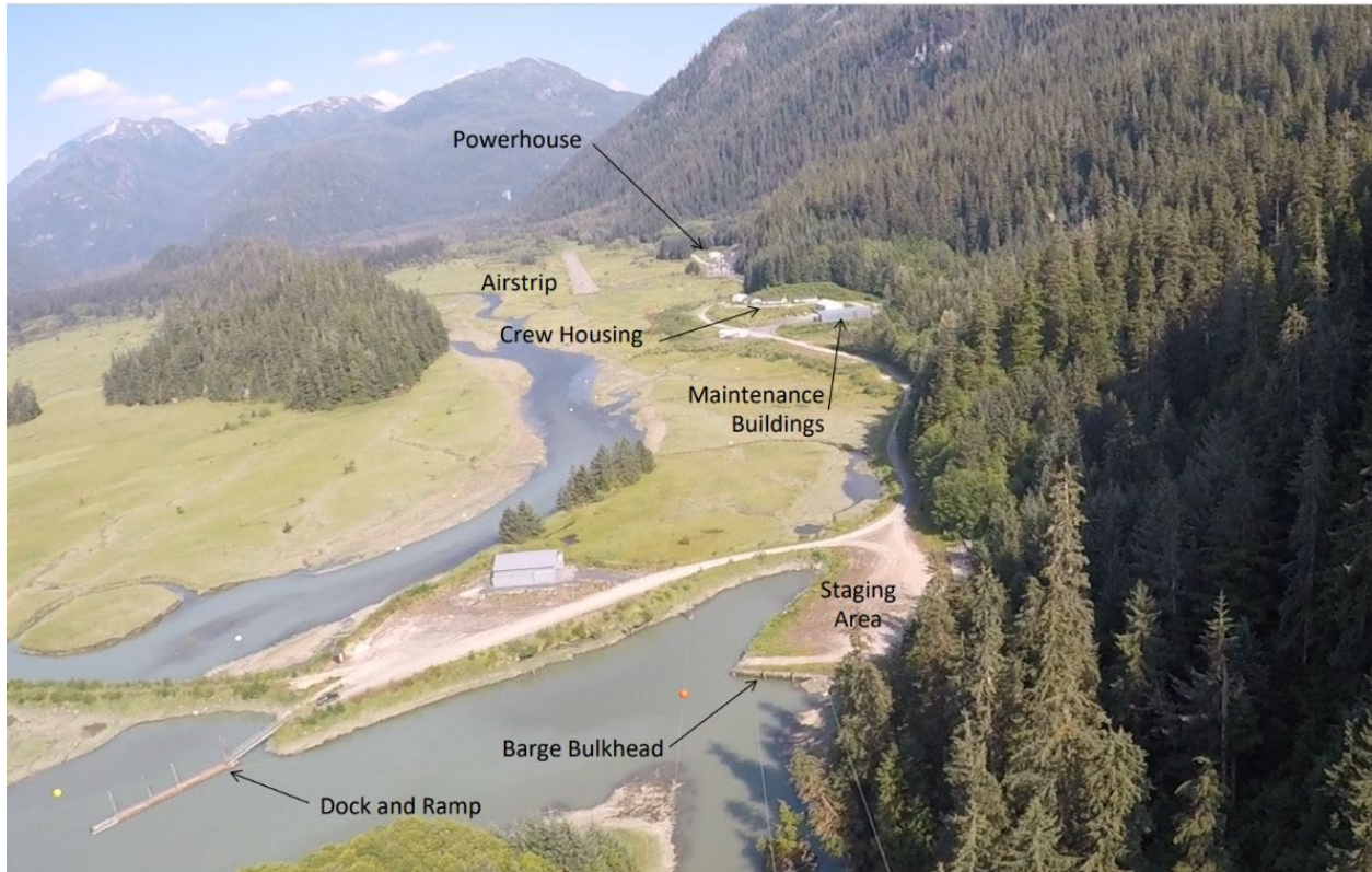
Photo 2-1 Tyee Lake Hydroelectric Project Development.
