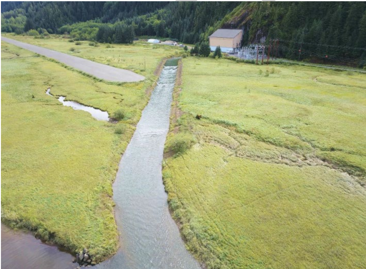
Photo 4-9 Tyee Lake Project Tailrace, Looking Upstream towards the Powerhouse. Source: ADF&G 2018.
