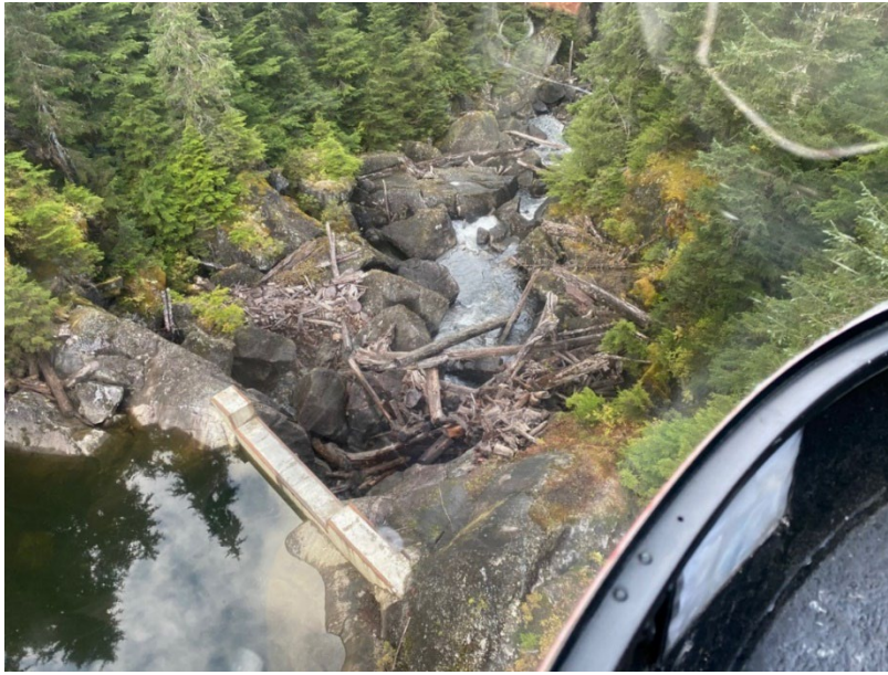
Photo 4.3-1 Tyee Creek at Tyee Lake Outlet Weir Looking Downstream when no Water is Flowing from Tyee Lake over the Weir.
