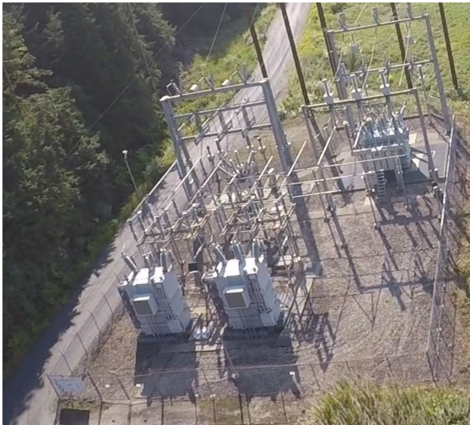
Photo 2.1-6 Switchyard Showing Space for Installation of Third Transformer.
