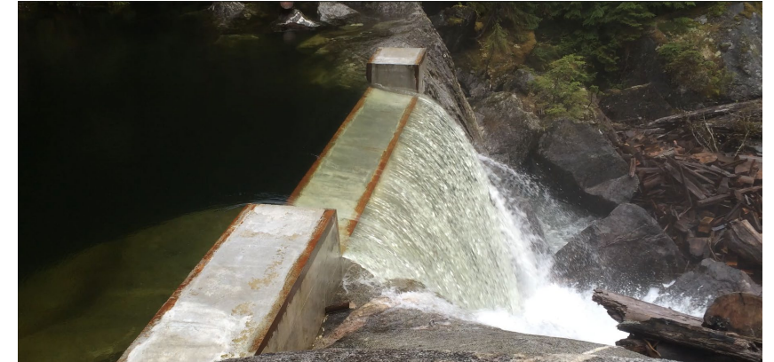
Weir constructed in 2013 at lake outlet USGS Gage 15019990 measures lake WSEL
