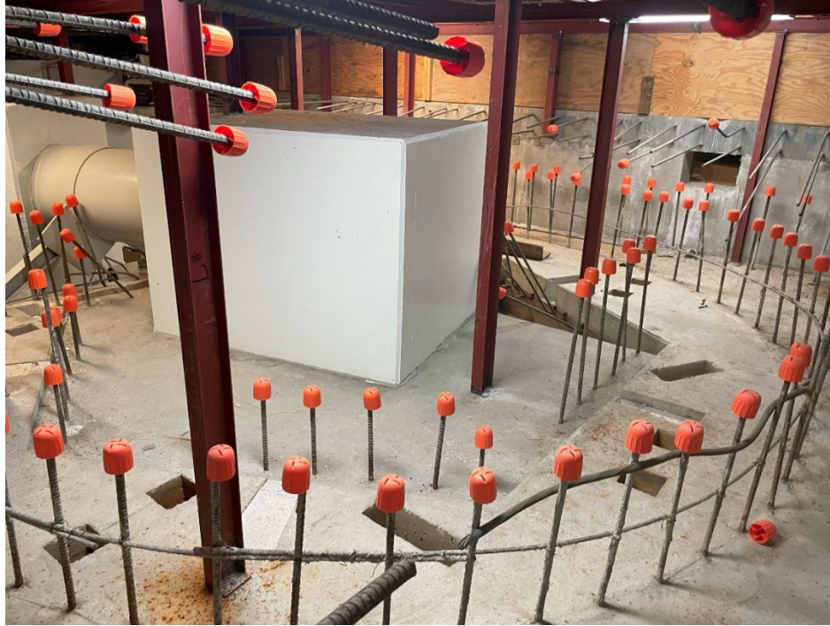
Photo 2.1-5 Penstock and Concrete Thrust Box for the Third Unit.
